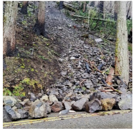
This 2018 photo shows a landslide on the historic highway triggered by trail work while it was still closed after the fire
