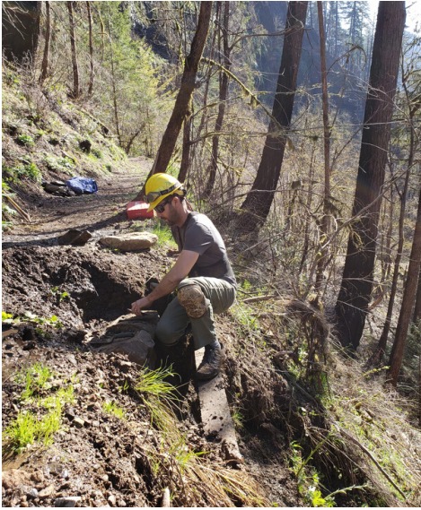
Installing a stone retaining wall on Eagle Creek Trail
