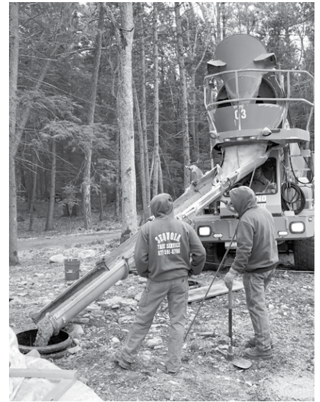
Pouring the footings.
