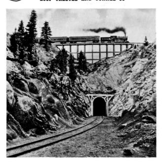
A train going through Tunnel 33 had to ascend one and a half miles of loop track (circling a mountain in the process) before it reached the Loop Trestle. The vertical distance between the two sections of the track is 150 feet.
