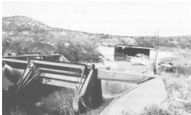
Figure 81—Middle Rio Grande Conservancy District water control facility south of Isleta Pueblo. Photo by author.
