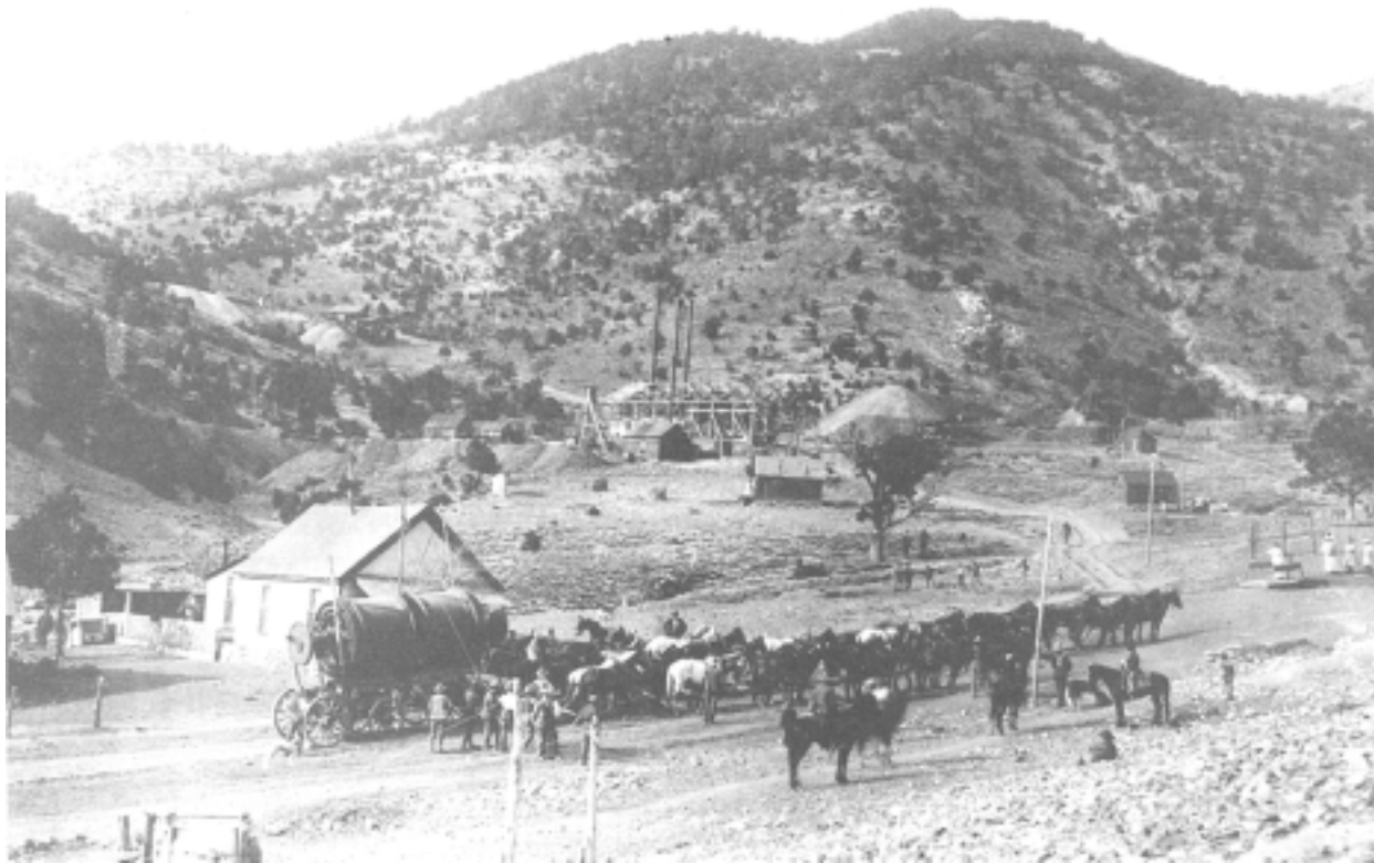
Figure 38—Mining operation, Kelly, Socorro County, 1905. Courtesy Mary Louise (Brown) Dillard and New Mexico Bureau of Mines Photo Archives, Socorro.
