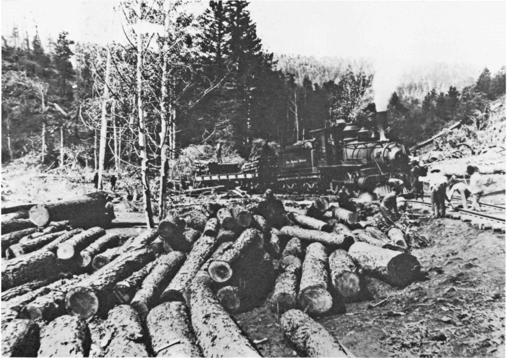
Figure 20. Zuni Mountain Railway locomotive Number 4 on a track-laying job. On a big logging show, it was quite a job to coordinate logging and railroad construction in order to cut trees efficiently and to use the limited length of available rail effectively. In many instances, the logging was done before the rails were laid, and this view appears to be such an example. Cibola National Forest collection.
