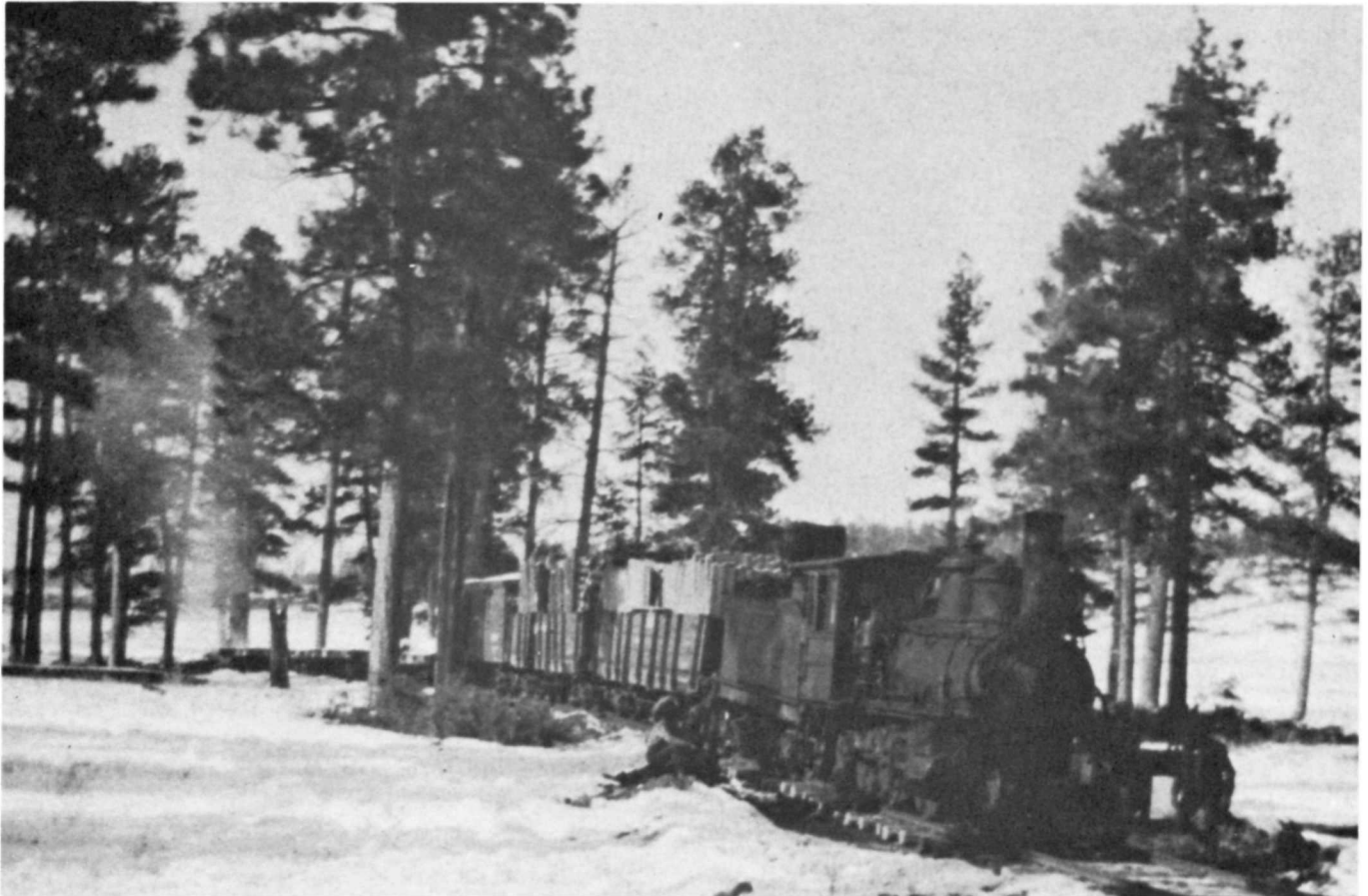
Figure 52. A borrowed Santa Fe Railway locomotive, Number 2303, off the rails on new logging track of the Zuni Mountain Railway, January 4, 1906. V. J. Glover collection.
