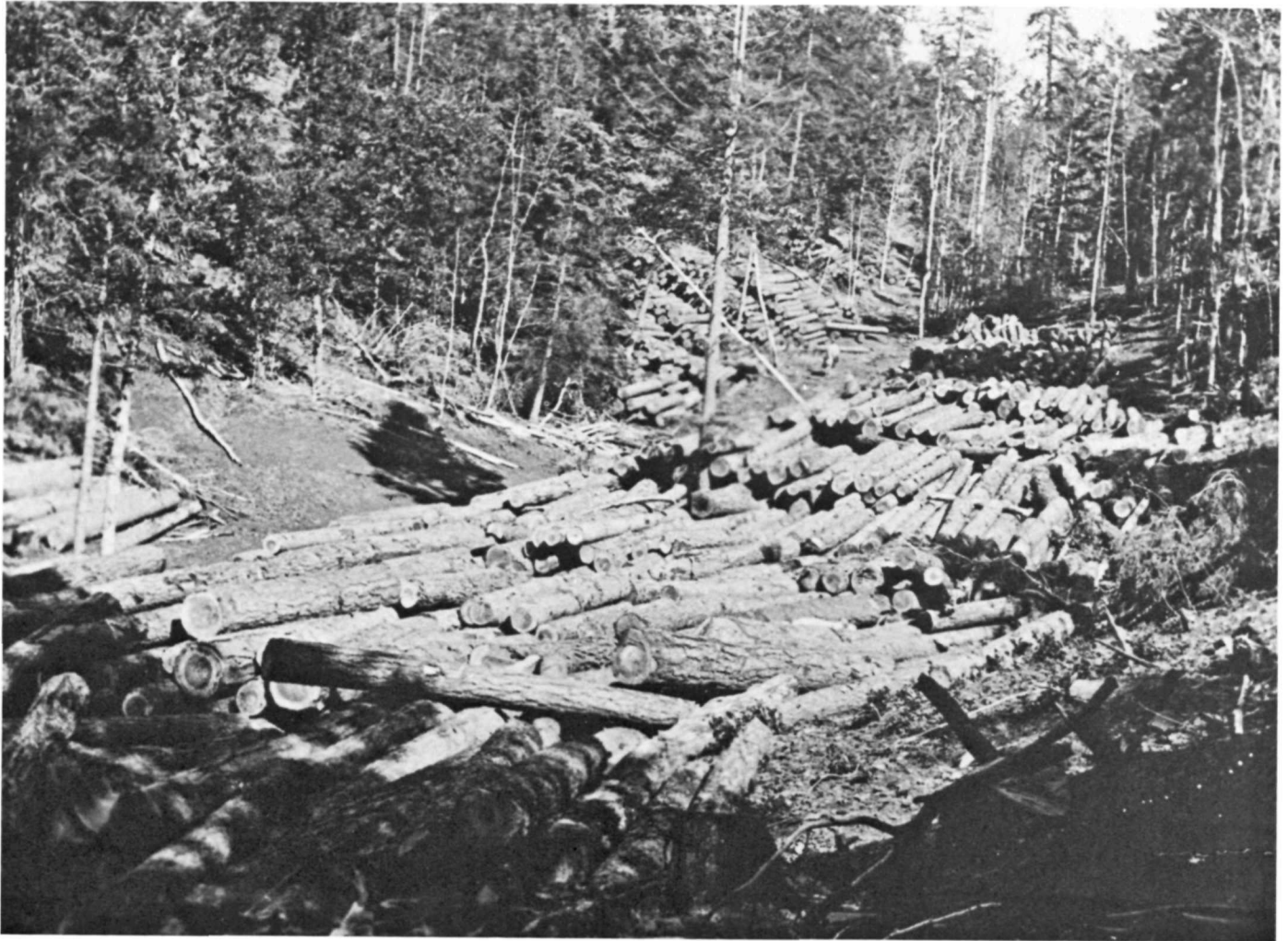
Figure 19. Log landing along a future spur track, American Lumber Company. These logs have been yarded in a little valley preparatory to loading on the cars when the spur track is built. It appears the roadbed has already been graded. Cibola National Forest collection.
