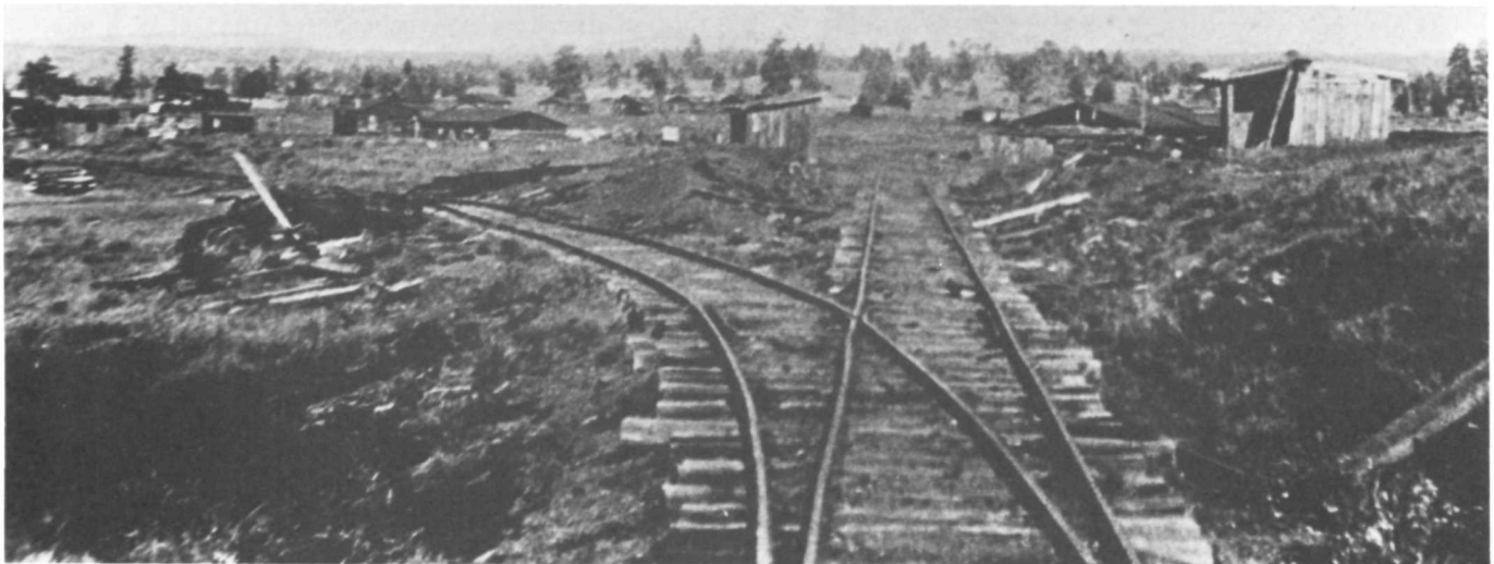
Figure 24. The logging camp at Sawyer on the American Lumber Company. The railroad track construction is typical of logging railroads with a minimum of grading, steep grades, and earth ballast between the ties. Locations of switches such as this one can often be determined long after the track was removed through surviving examples of the long switch ties, which ranged from 8 to 16 feet in length. Cibola National Forest collection.
