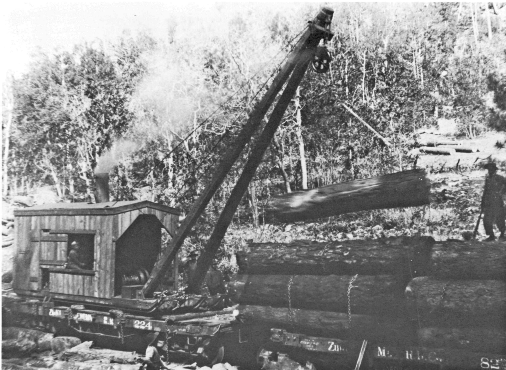
Figure 7. One of the American Lumber Company's steam loaders at work. The skids on which the loader rides and the construction of the stiff-leg boom can be clearly seen. The log cars are the wooden type owned by the Zuni Mountain Railway. Note that the chains used to secure the logs to the cars are wrapped around the first two layers of logs, then tightened by the upper two or three logs laid on top. Cibola National Forest collection.
