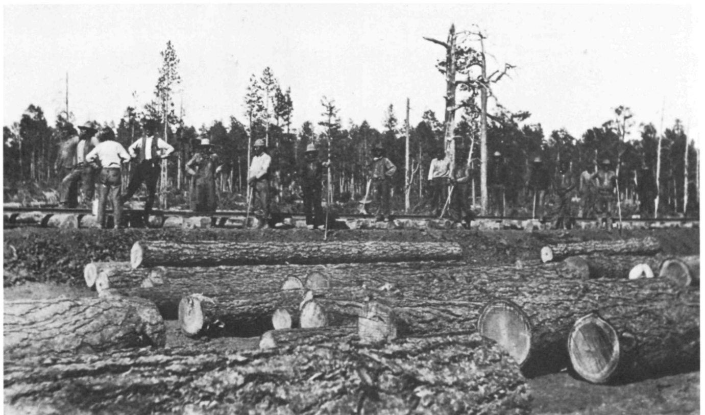
Figure 65. Zuni Mountain Railway track gang comprised mostly of Navajo Indians. The track is not yet ballasted, and is laid on a newly graded roadbed. Cibola National Forest collection.
