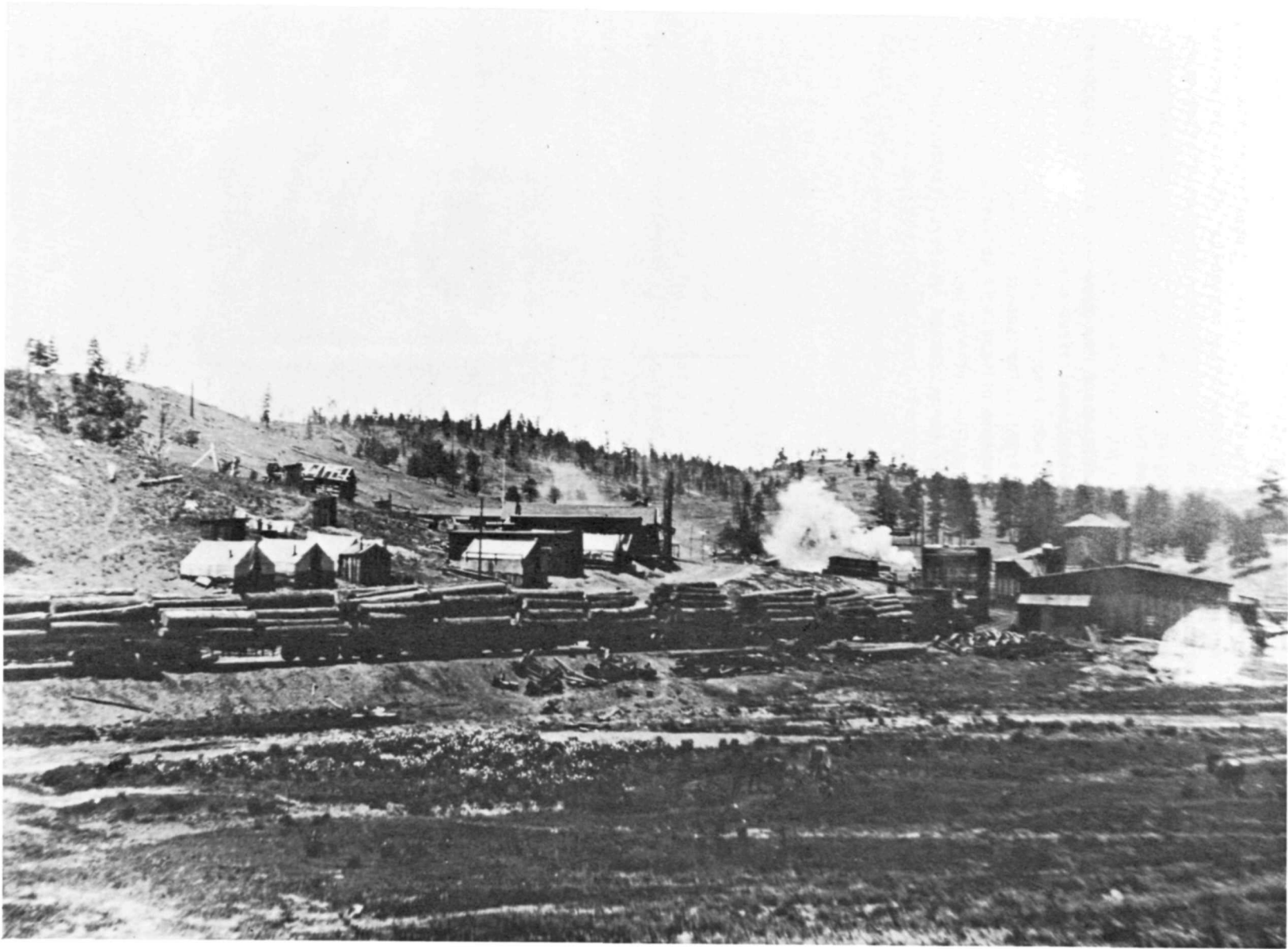
Figure 9. An overall view of the main logging camp at Kettner. This was the area devoted to railroad and mechanical matters, with workshops and maintenance facilities of all kinds. Cibola National Forest collection.
