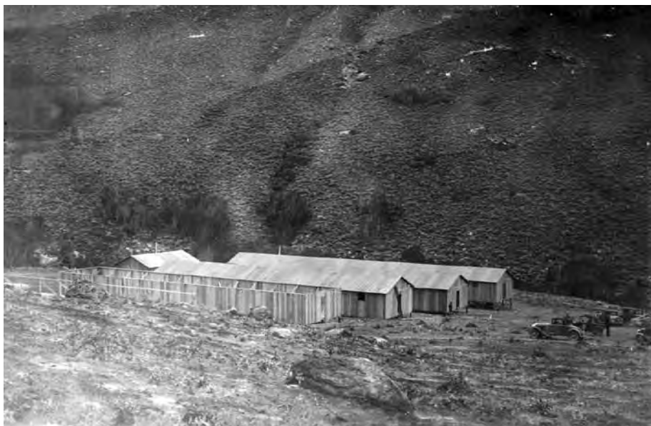
Camp Lamoille Barracks under Construction, 1933. ( Northeastern Nevada Museum Archives, Elko, Nevada )
