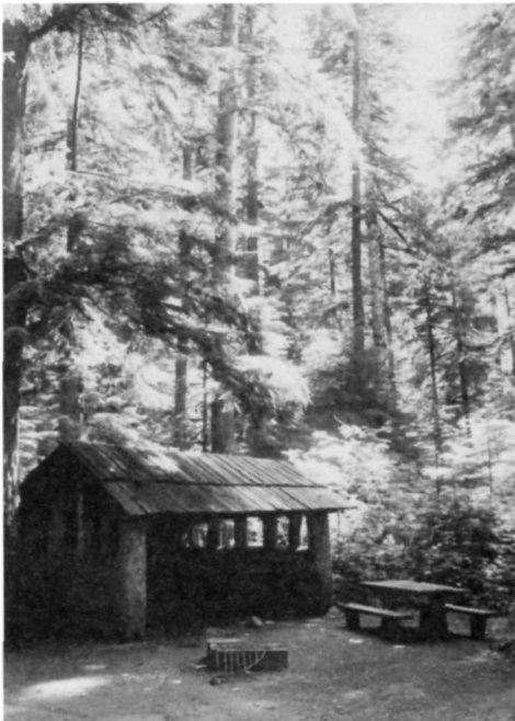
CCC shelter at one of the campsites in Bedal Campground
