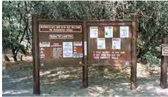
Figure 10B-29—This bulletin board structure is made of steel pipes, which is appropriate in this off-highway vehicle (OHV) site. Shawnee National Forest, Northeastern BEIG Province.
