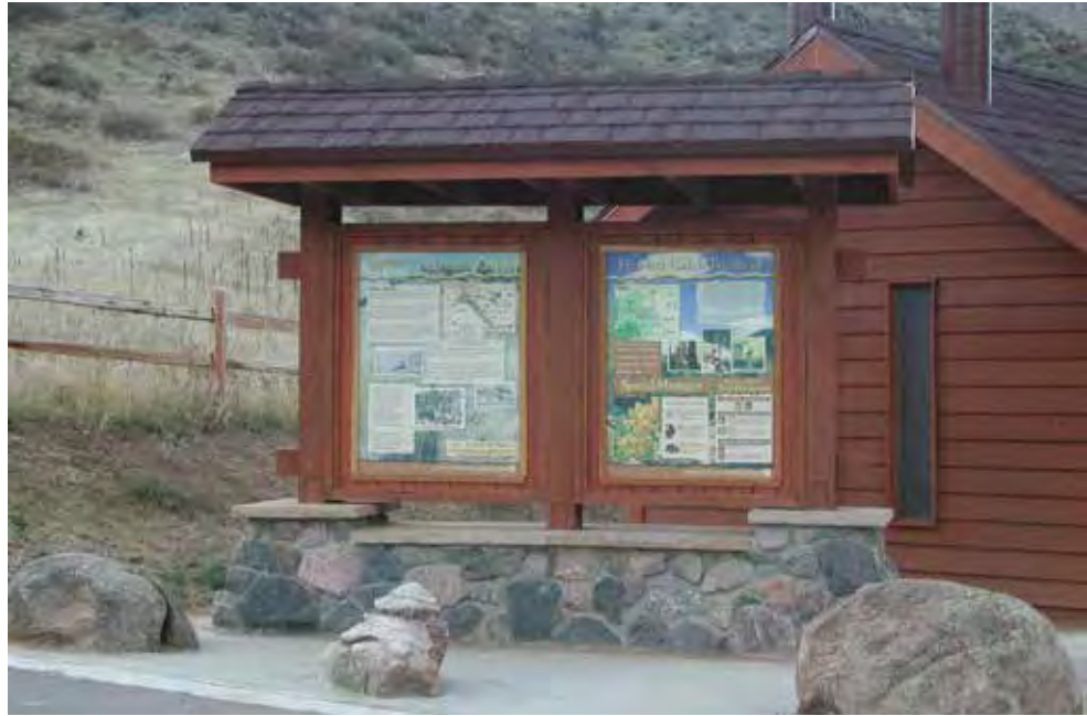
Figure 10B-9—Trailhead VIS is built to complement the adjacent building. Rock barriers prevent vehicles from encroaching into the space. Arapaho-Roosevelt National Forest, Rocky Mountain BEIG Province.
