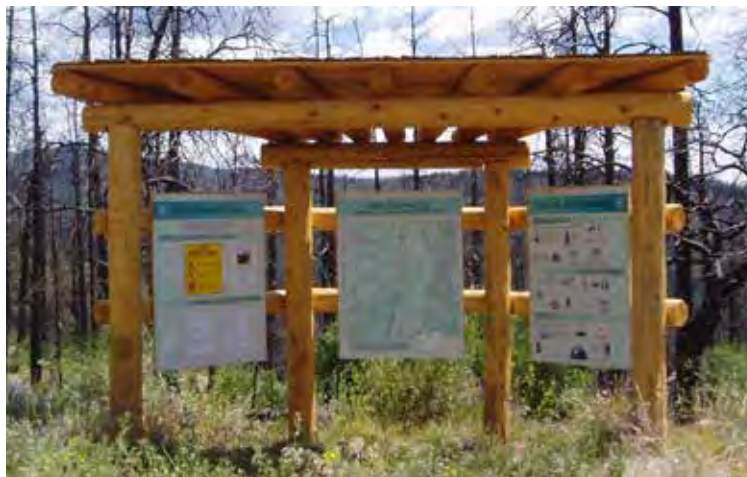
Figure 10B-30—Trailhead VIS structure built with round timbers appropriate for its setting. Santa Fe National Forest, Southwest BEIG Province.
