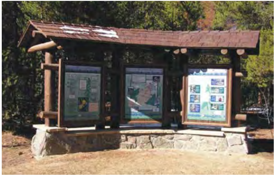
Figure 10B-33—This kiosk has heavy timbers that fit well in this forested environment; the rock anchors the structure. The kiosk is a combination of VIS and interpretive information. Byers Creek Campground, Arapaho and Roosevelt National Forest, Rocky Mountain BEIG Province.
