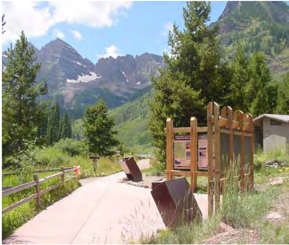
Figure 10B-37—This VIS structure easily can be made longer or shorter to hold more or fewer panels. There are two VIS and one interpretive fiberglass embedded panels all addressing wilderness values, use, and scenic views. Maroon Bells Recreation Area, Aspen Ranger District, White River National Forest, Rocky Mountain BEIG Province.
