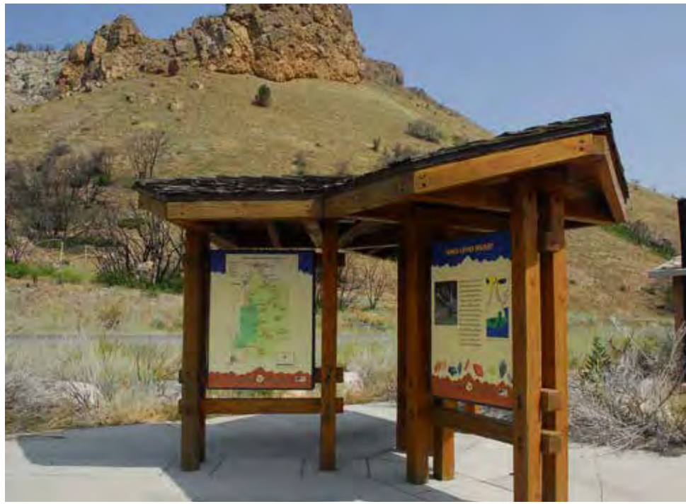
Figure 10A-24—This kiosk uses colors reflected in the landscape and appropriately sized lumber for the area. Nebo Loop National Scenic Byway, Unita National Forest. Rocky Mountain BEIG Province.
