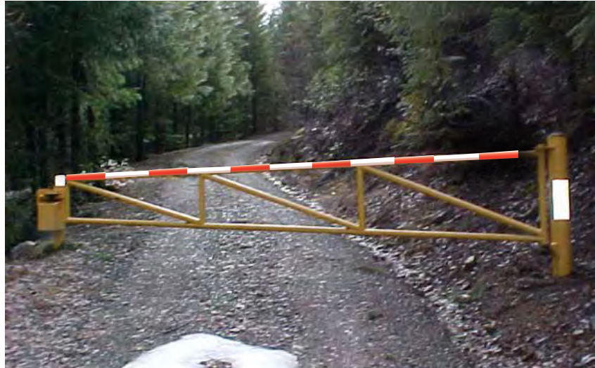
Figure 3B-1—Retroreflective tape on gate arm.
