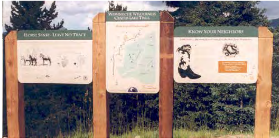
Figure 10B-35—Three-panel VIS structure for a campground with information on digital laminate. Posts have the same motif and can vary in height. San Juan National Forest, Rocky Mountain BEIG Province.
