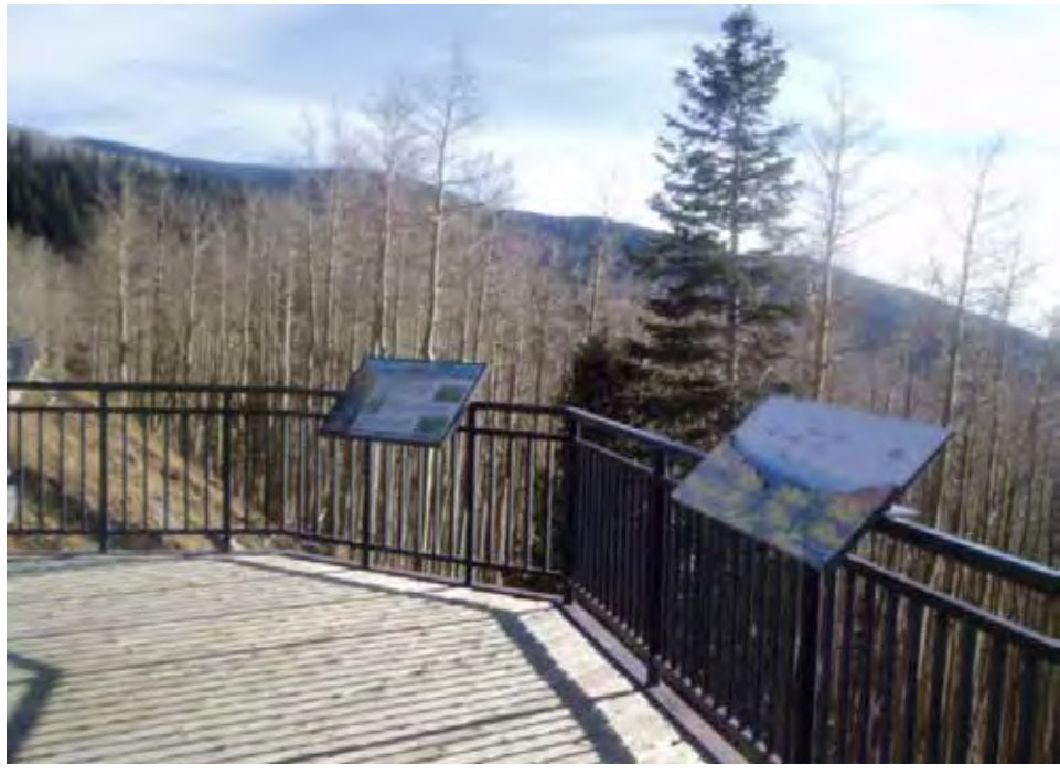
Figure 10A-29—Low-profile signs are attached to a railing. Santa Fe National Forest. Southwest BEIG Province.
