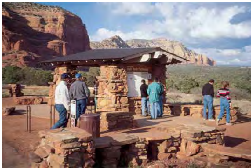
Figure 10B-34—This VIS has information about the Bell Rock Pathway. The structure incorporates the surrounding rock to tie it to the setting. Coconino National Forest, Southwest BEIG Province.
