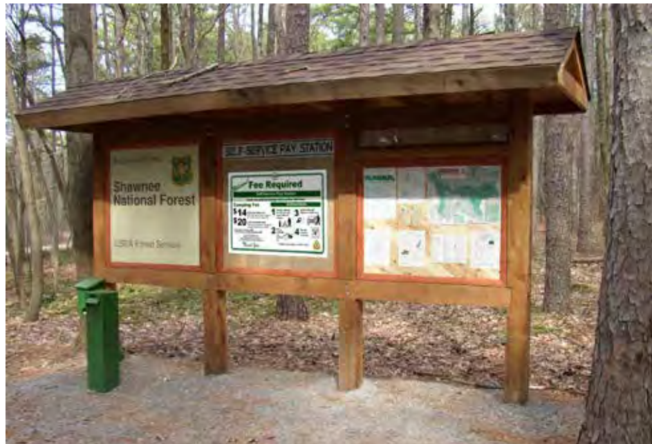
Figure 10B-7—A roof is provided over this VIS pay station. Shawnee National Forest, Northeastern BEIG Province.
