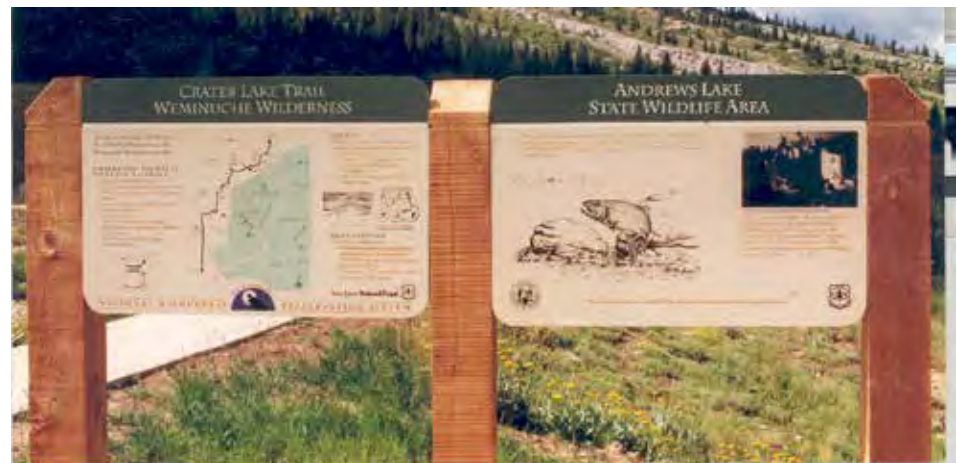
Figure 10B-36—Two-panel VIS structure uses the same motif as the three-panel structure in figure 10B-40. The center post is facing a different direction. San Juan National Forest, Rocky Mountain BEIG Province.
