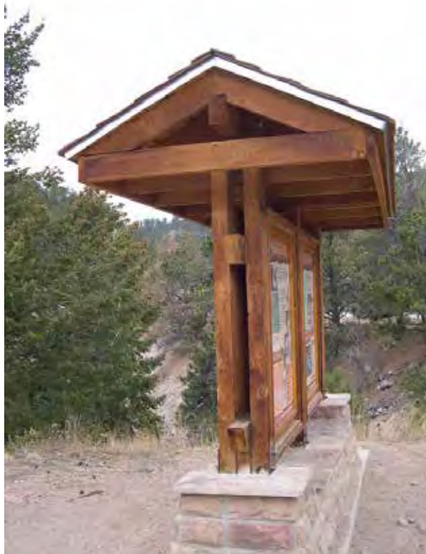
Figure 10B-32—Side view of structure at Indian Gulch Trailhead. Arapahoe and Roosevelt National Forest, Rocky Mountain BEIG Province.
