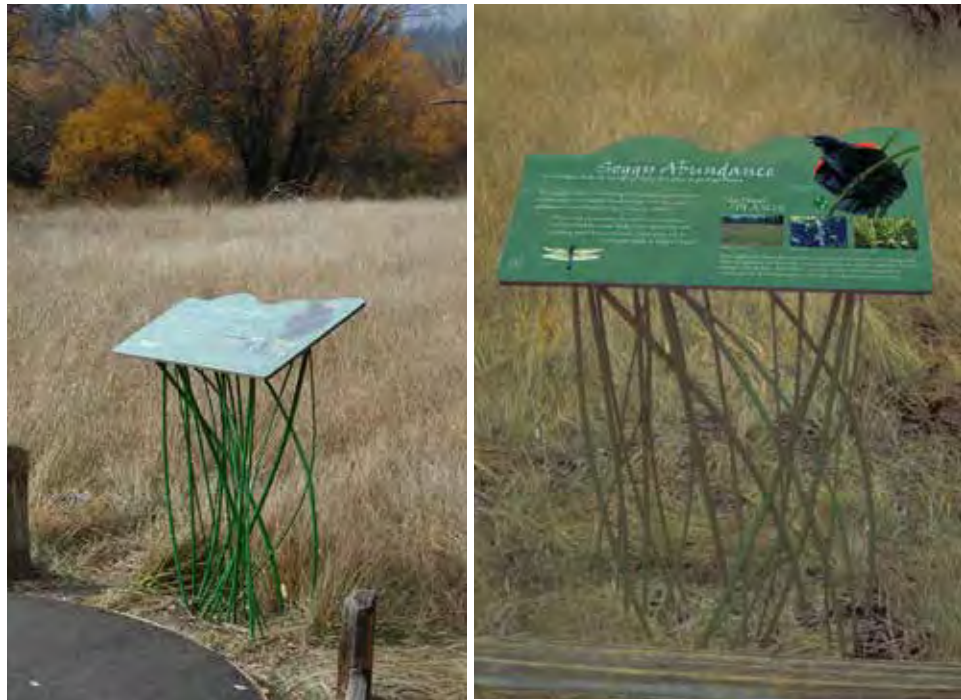
Figures 10A-31 and 32— The sign supports are designed to look like the reeds seen in the visitor center area. They continue from the sign face to the ground. Taylor Creek Visitor Center, Lake Tahoe Basin Management Unit, North Pacific BEIG Province.
