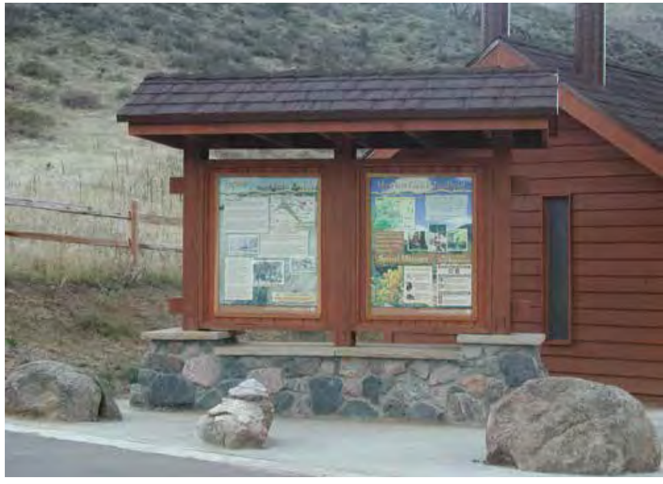
Figure 10A-34— This support uses local stone, and continues the design theme from the nearby building in size of wood and color at Hewlett Gulch. Arapaho-Roosevelt National Forest. Rocky Mountain BEIG Province.
