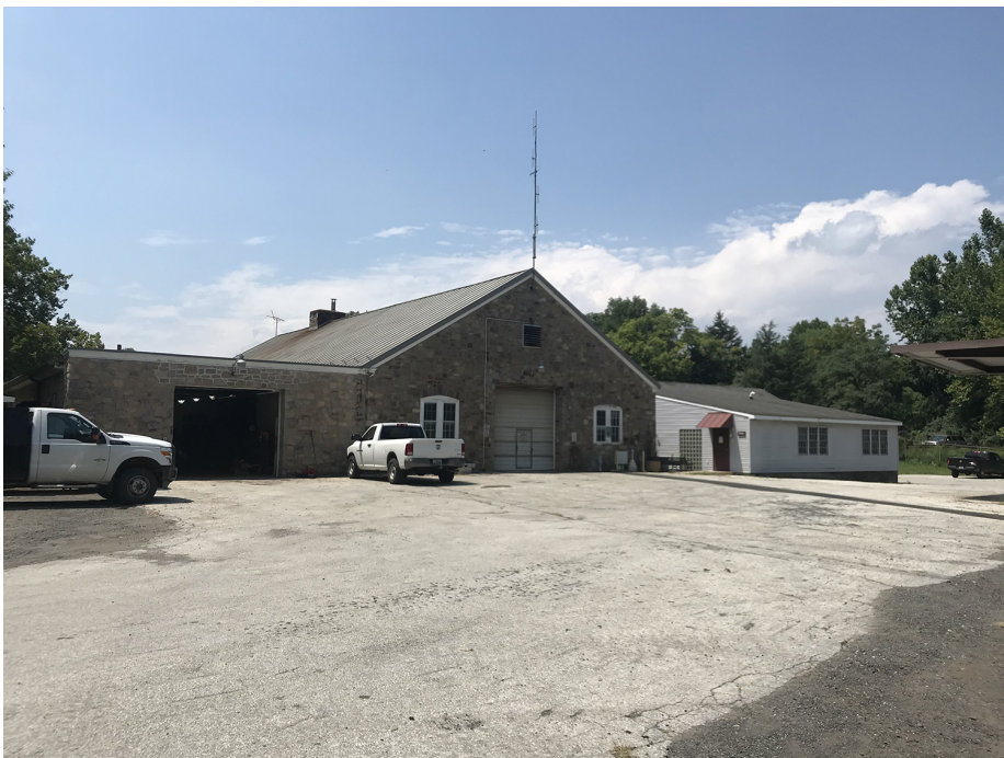
Figure 16. Maintenance Building, B-91, view southwest. (OCLP, 2019)
