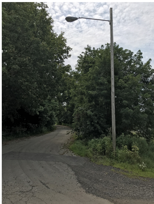
Figure 17. Overhead Lights, SS-85, view southeast. (OCLP, 2019)
