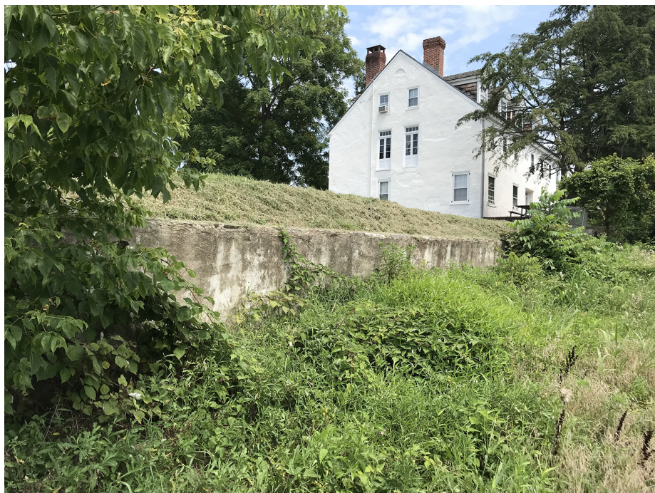
Figure 11. Mordecai Moore Retaining Walls, S-121, view northeast. (OCLP, 2019)
