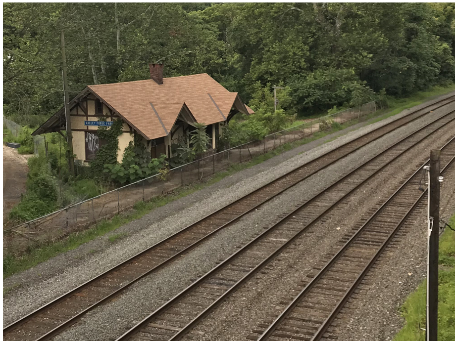
Figure 13. Port Kennedy Railroad Depot, B-98, view southwest. (OCLP, 2019)
