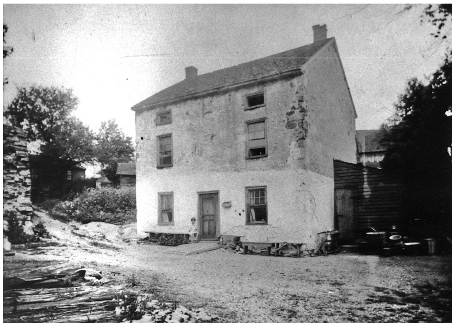
Figure 5. The Bird House/Port Kennedy Commissary, ca. 1880s.
