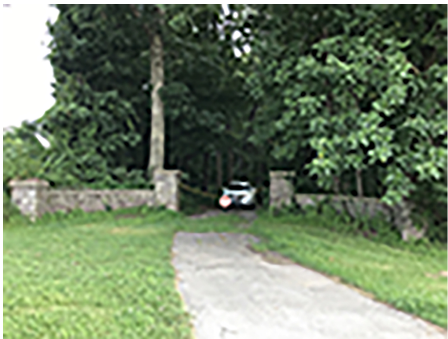
Figure 21. Walnut Hill Estate Stone Gate Post System, S-99, view south. (OCLP, 2019)
