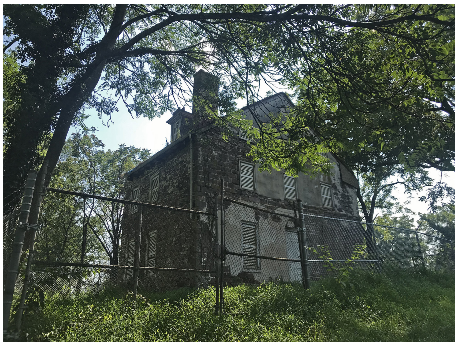
Figure 17. Pawling Mansion, B-86, view southwest. (OCLP, 2019)
