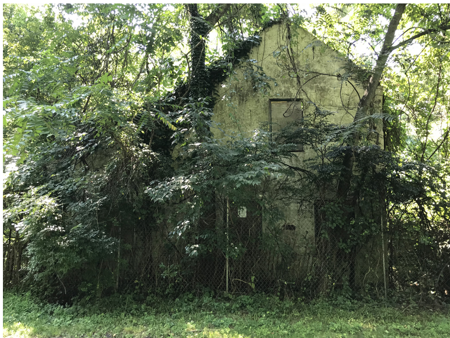
Figure 16. Meadow Grove Spring House Ruin, B-81, view southwest. (OCLP, 2019)
