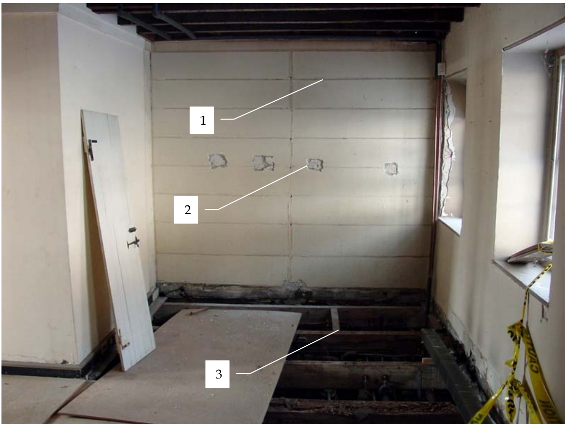
Photo 102a – View of west wall, Room 102.
