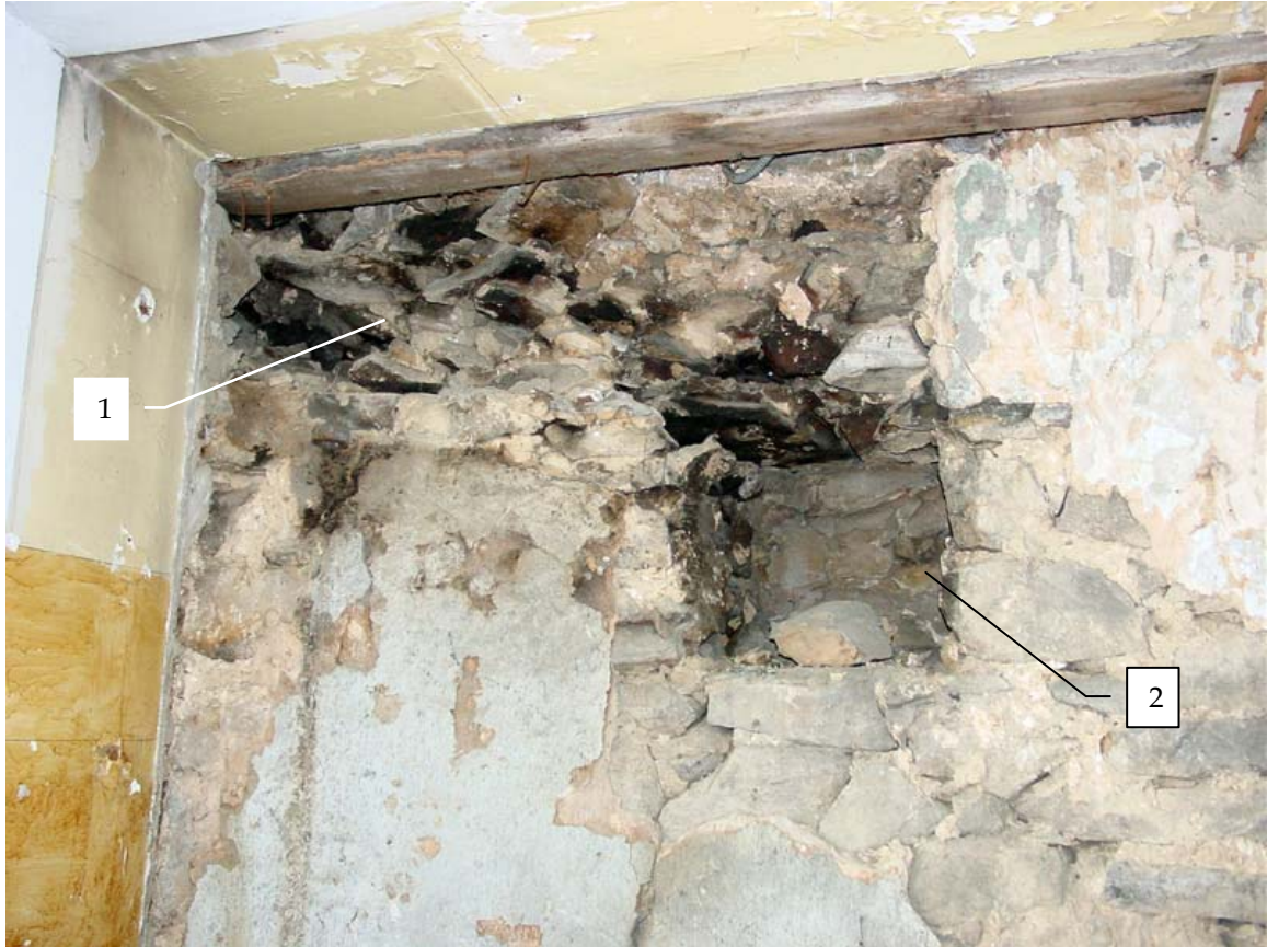
Photo 106a - Detail view of northwest corner of Room 106, looking north.
