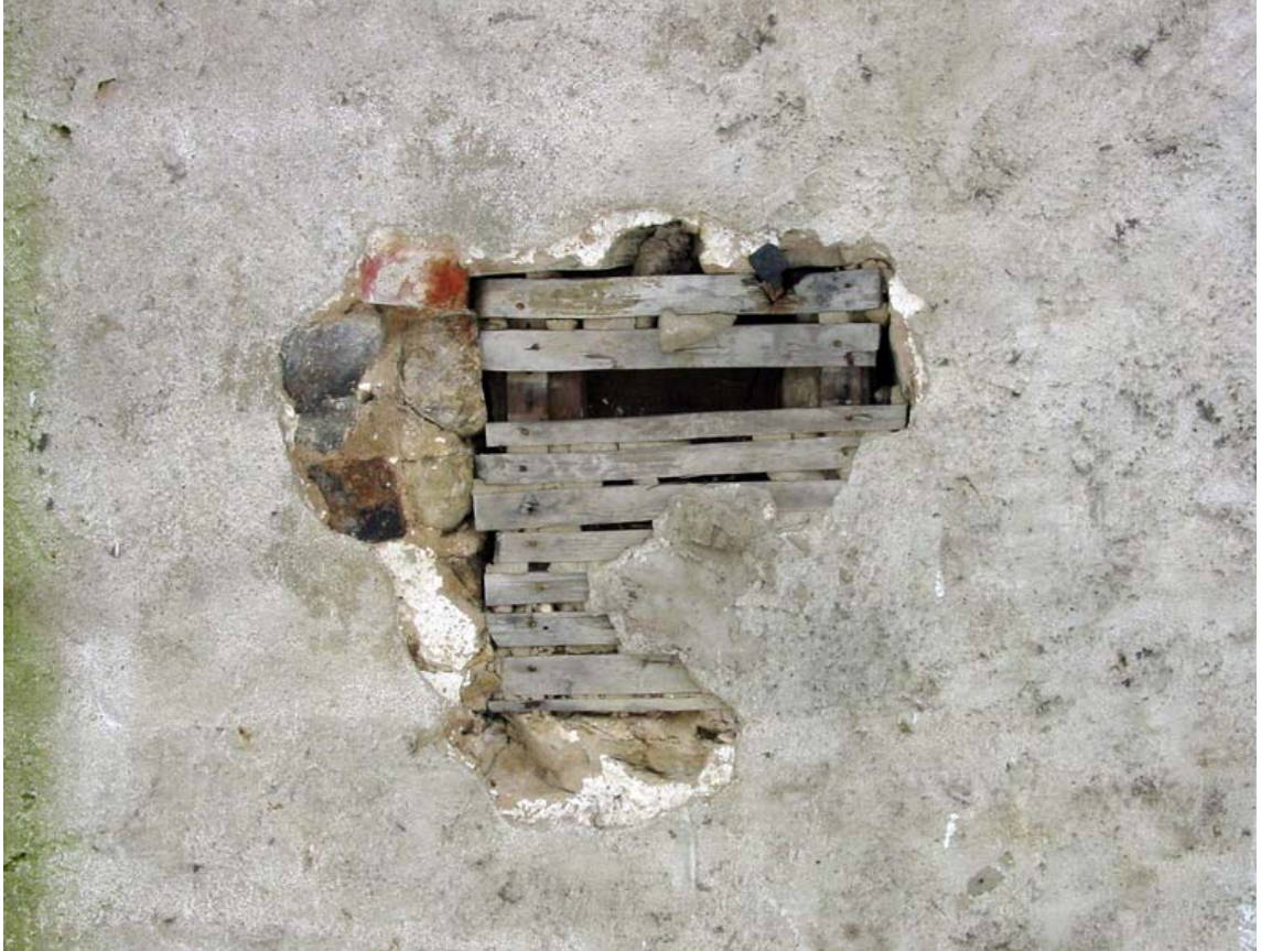
Photo NEb - Detail view of lath at lintel pocket, north façade of east addition, looking south.
