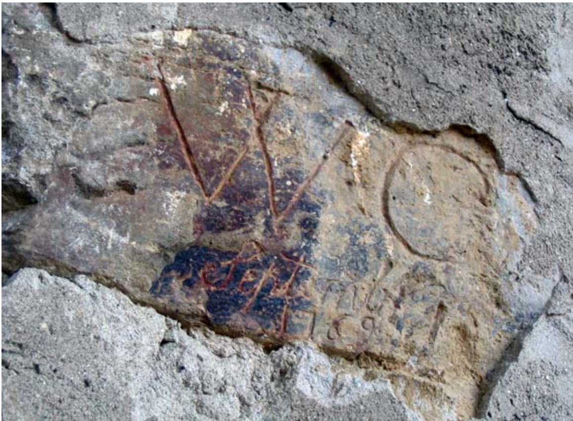
Figure 6: Detail view of one of the corner stones at the southwest corner of original kitchen block with the inscription, "W C September 1769."
