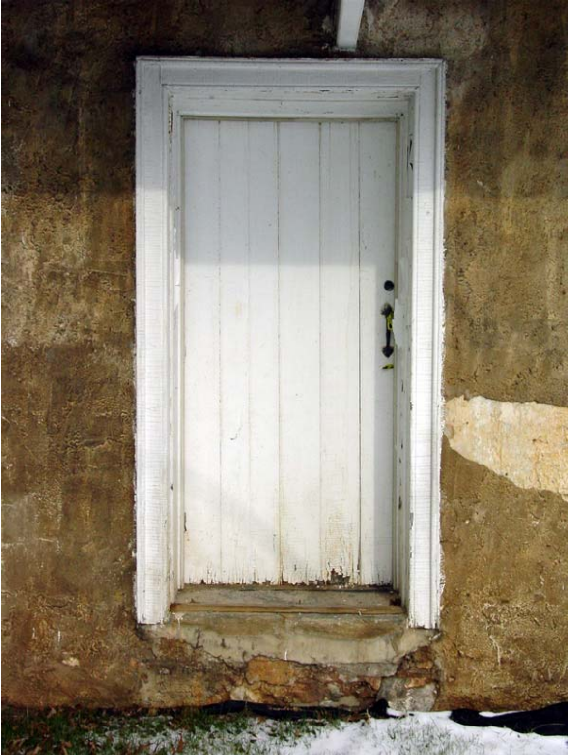
Photo SEd – Exterior view of door to east addition, looking north. Wood door and frame appear to be original, c. 1830.
