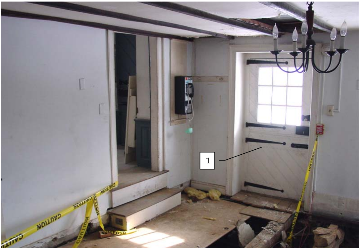
Photo 104c – Interior view of Room 104, looking southeast.
