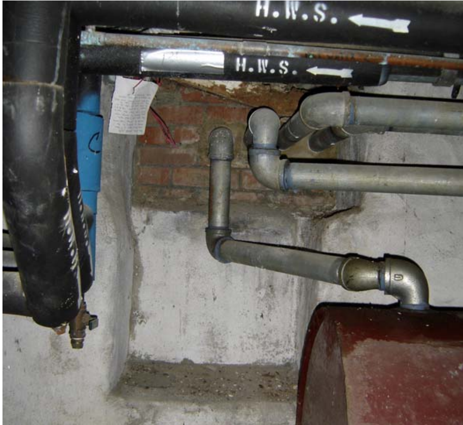
Photo 002b - Former masonry opening and niche at north wall, Room 002, looking north.
