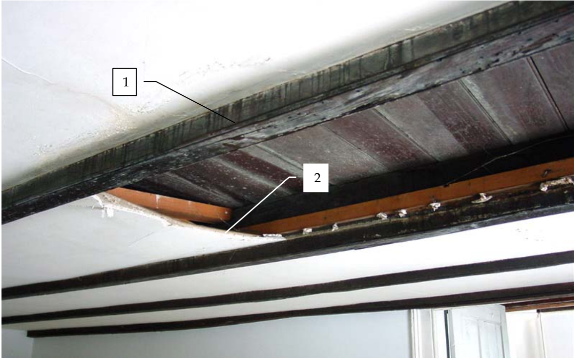
Photo 104b – View of ceiling, Room 104, looking northeast.
