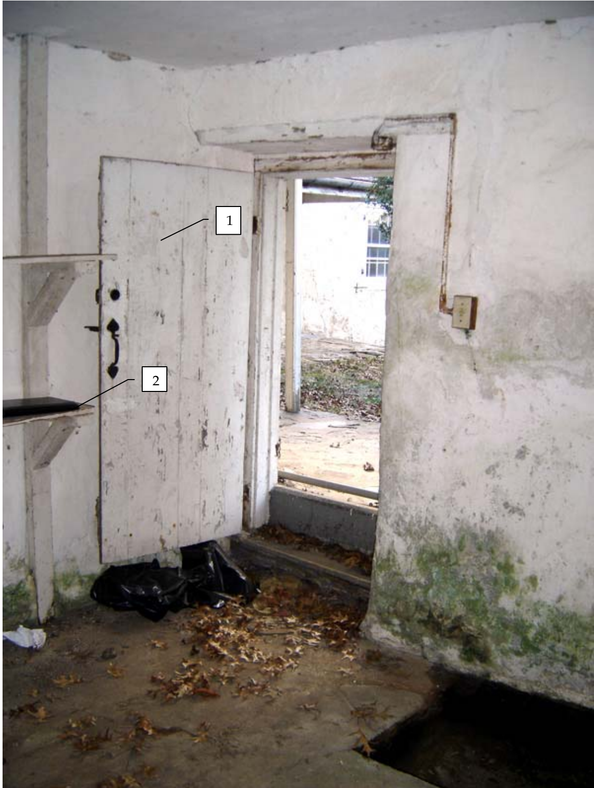
Photo 109c - Segment of springhouse interior, Room 109, looking southeast.
