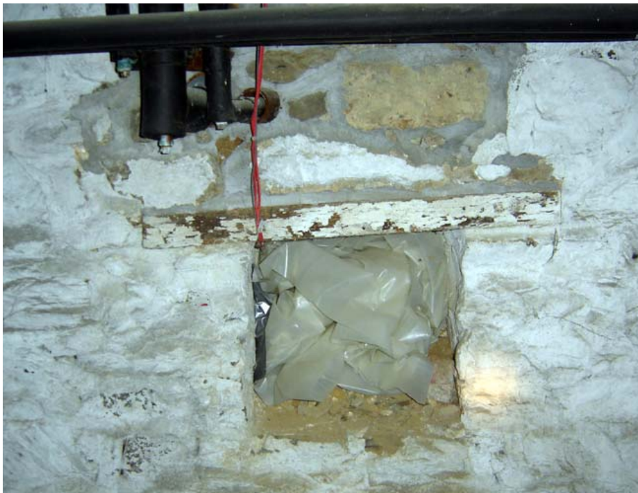
Photo 002c - Former masonry opening at west wall, Room 002, looking west.
