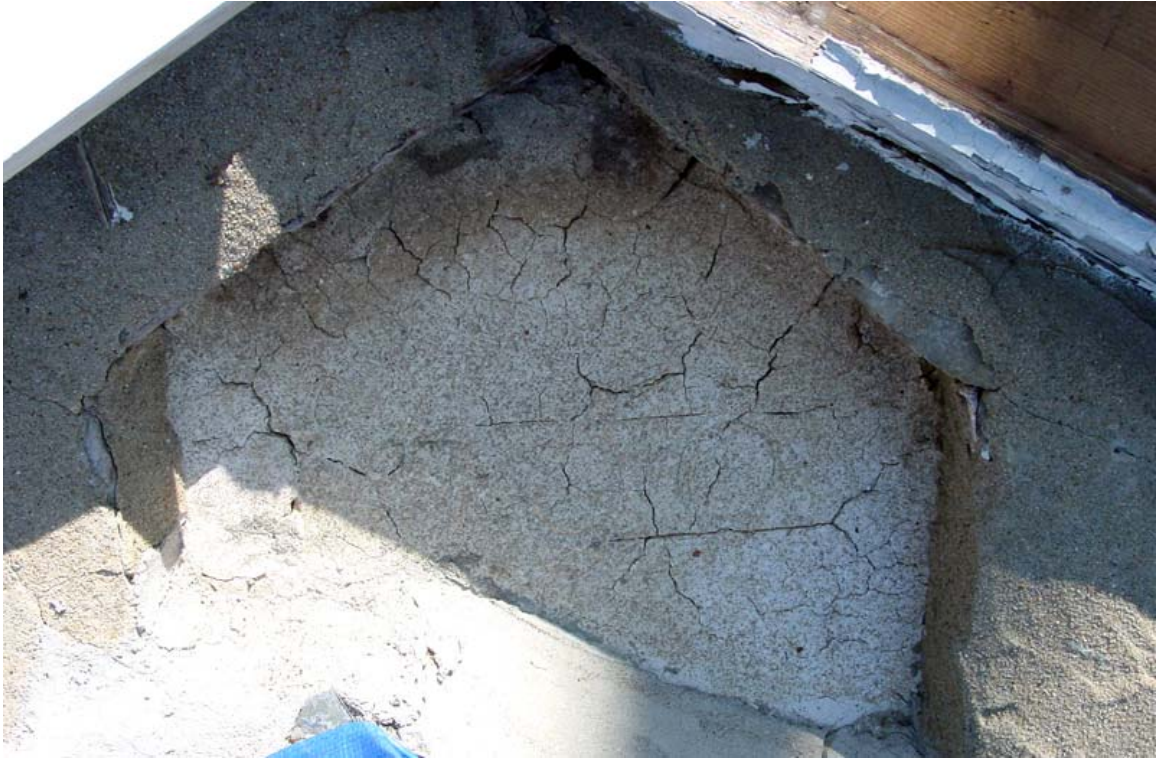
Photo WEc - Detail view of recessed stucco panel at west gable peak of main block, looking east. The inscription "1769" is faintly visible.
