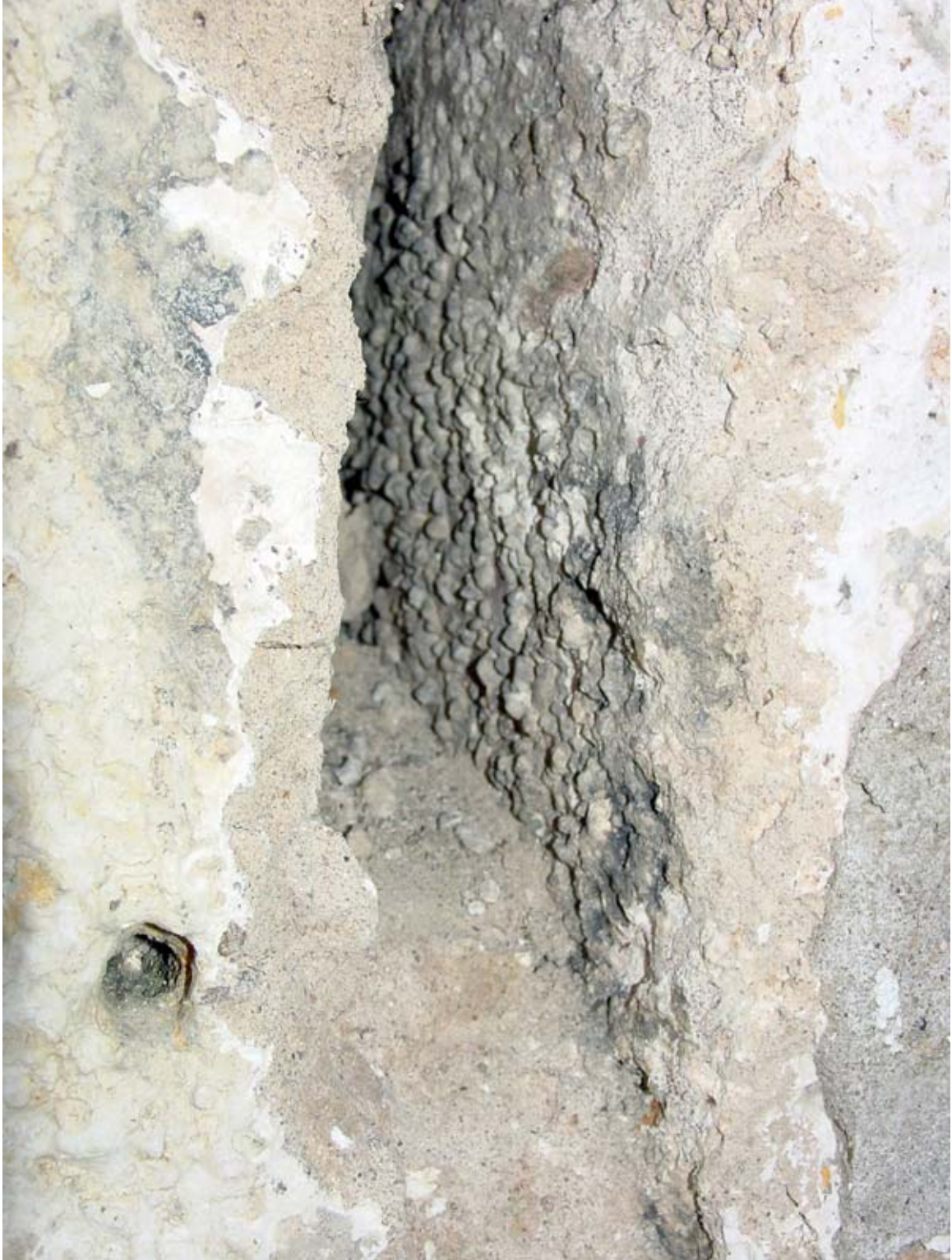
Photo NEd - Detail view of seam at north elevation between main block (right) and east addition (left), looking south. Note textured surface of stucco and that stucco wraps around east side of the main block. View represents the general location of Material Sample 26.
