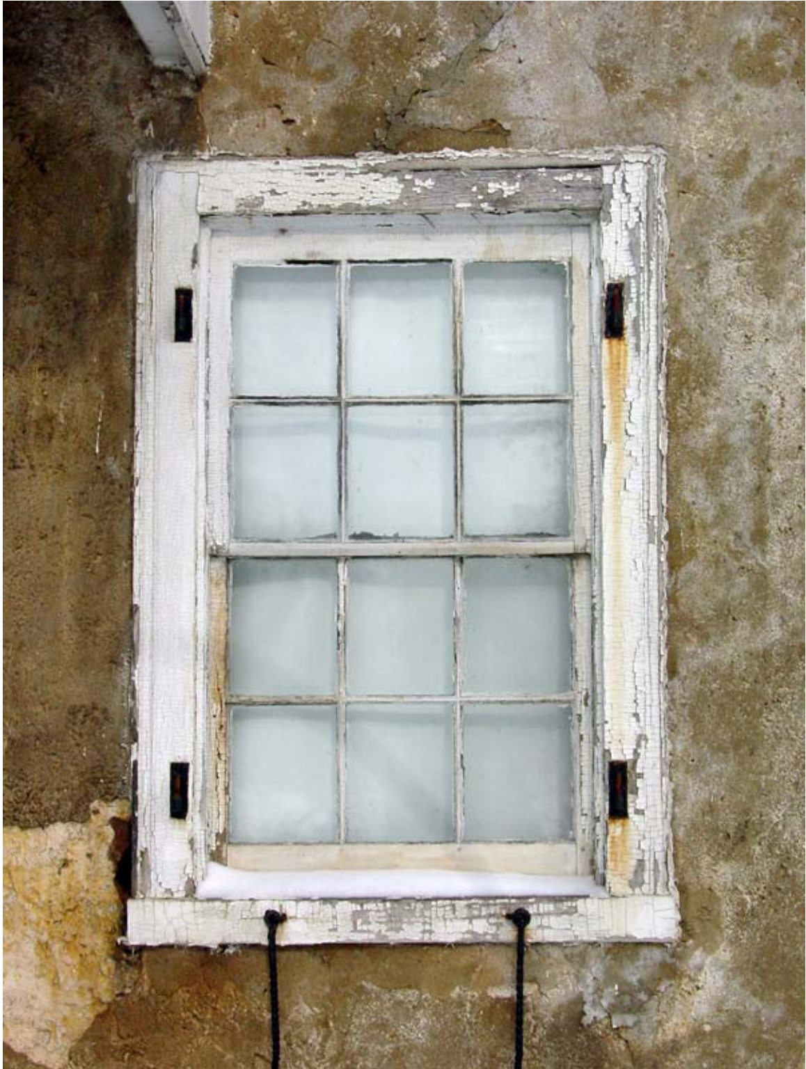
Photo SEe - Exterior view of Window 101, looking north.
