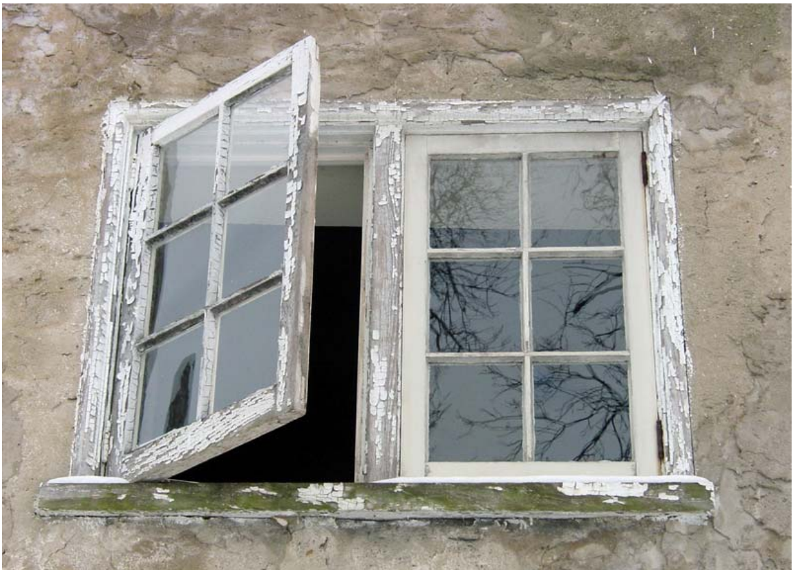
Photo WEd - Exterior view of Window 207, looking east.
