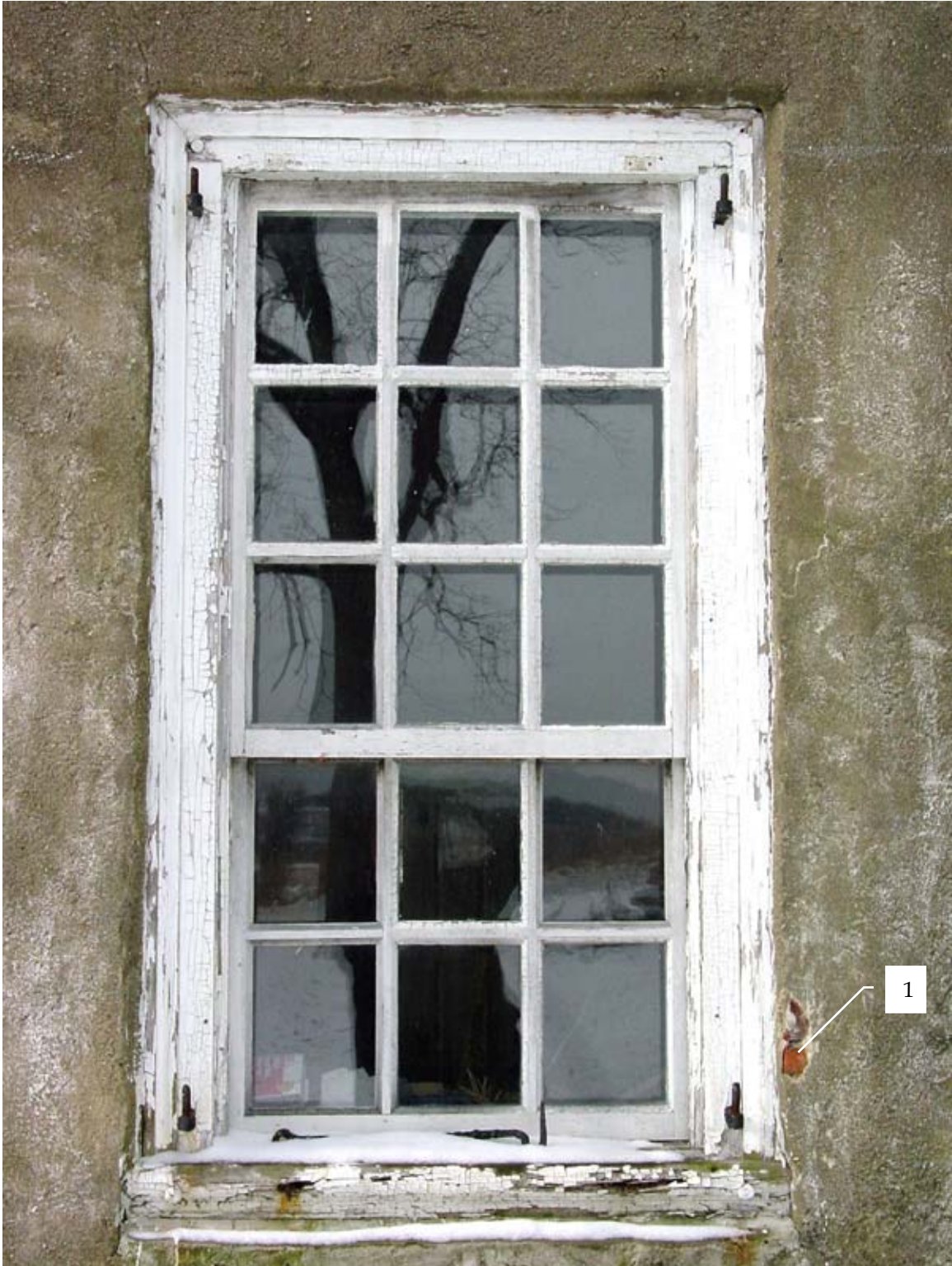
Photo EEd - Exterior view of Window 102, looking west.
