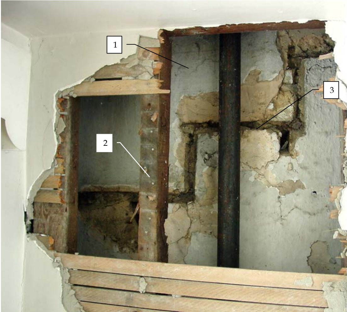
Photo 105a - Detail view of north wall, Room 105, looking north.
