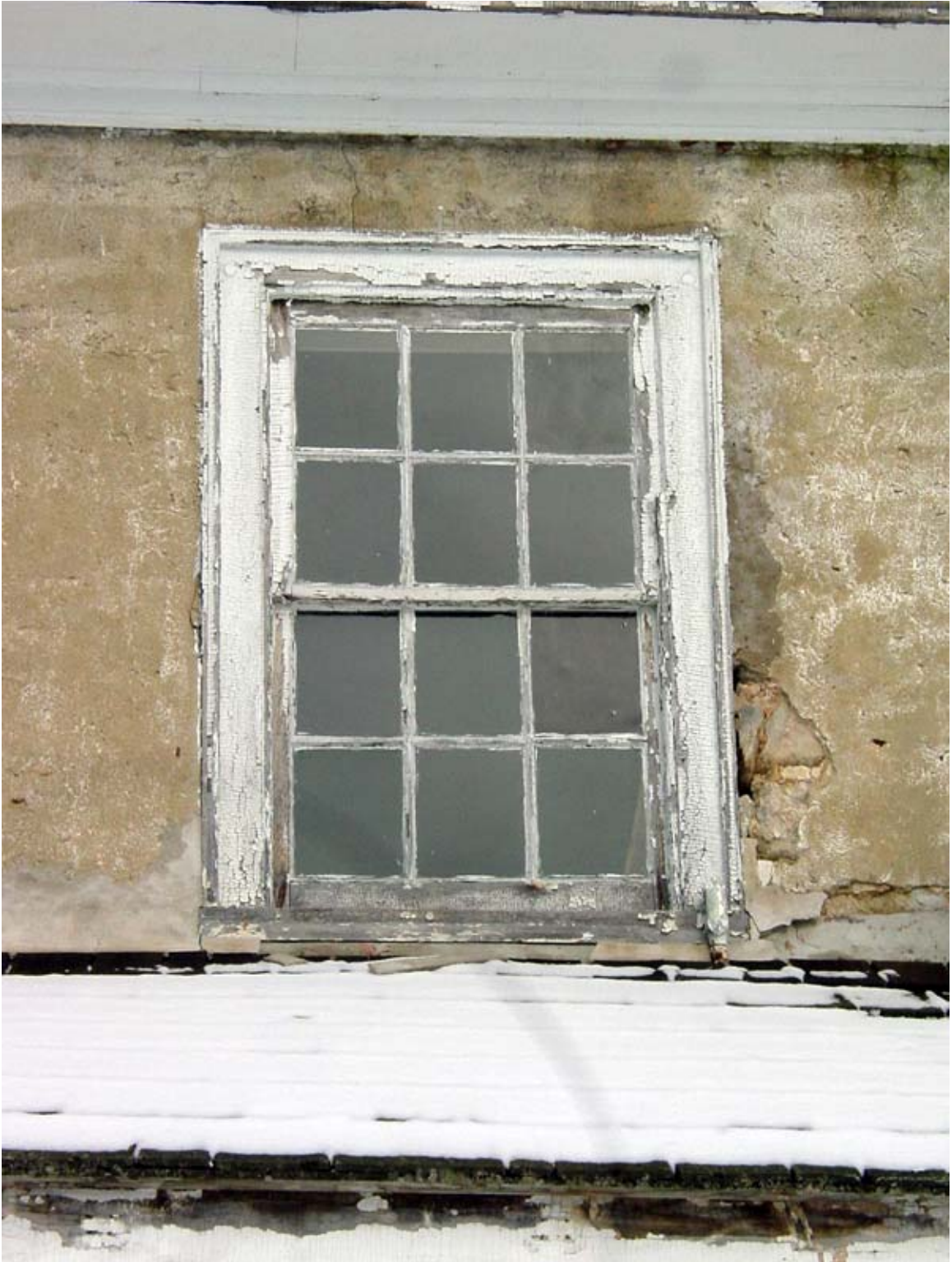
Photo SEi - Exterior view of Window 205, looking north.
