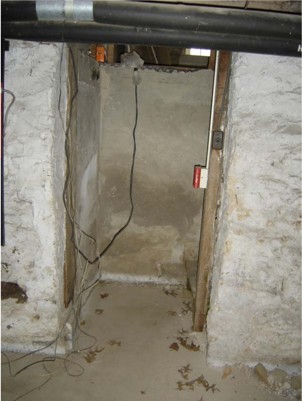
Photo 002d - Masonry opening at west wall, Room 002, looking west, into areaway for stair to Room 106. This opening was likely added as part of the c. 1926 alterations to the house to enable access to the basement from the first-floor kitchen.
