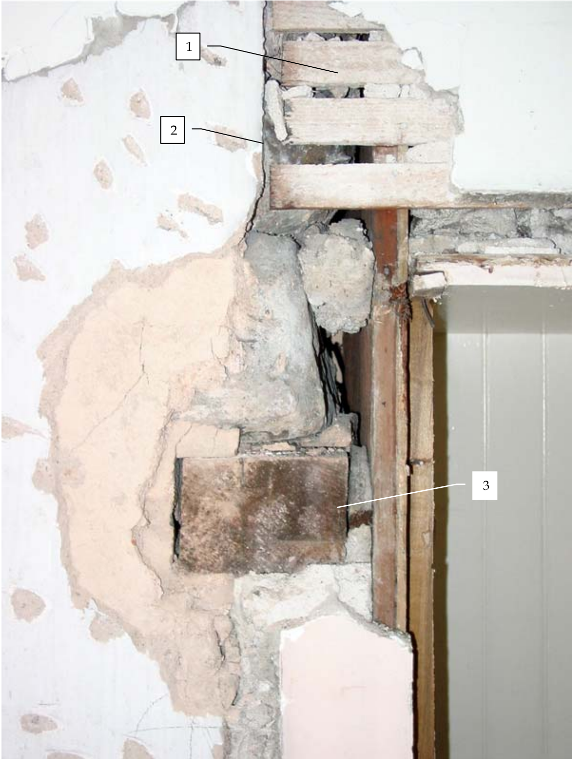
Photo 207a – Detail view of north jamb of former doorway between Rooms 203 and 207, looking east.
