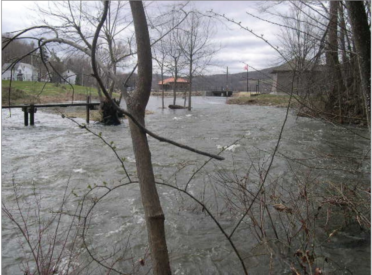
Figure 16. Flooding near the southern boundary of Vanderbilt Mansion National Historic Site in April 2007. The confluence of Crum Elbow Creek and the Hudson River is a low-elevation floodplain region susceptible to flood events and daily tidal fluctuations. NPS / DAVID HAYES
