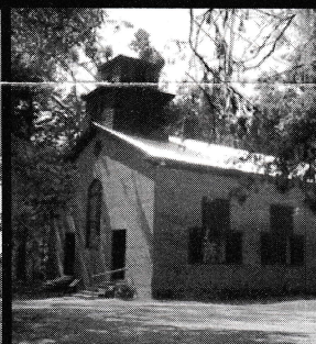
Rocky Springs Methodist Church
