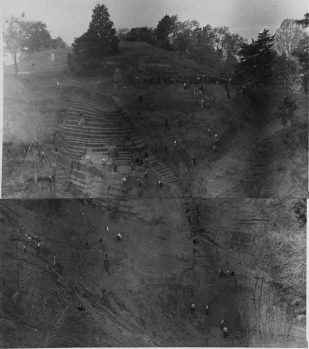
5. View of erosion No. 27 near Fort Micala, Louisiana
