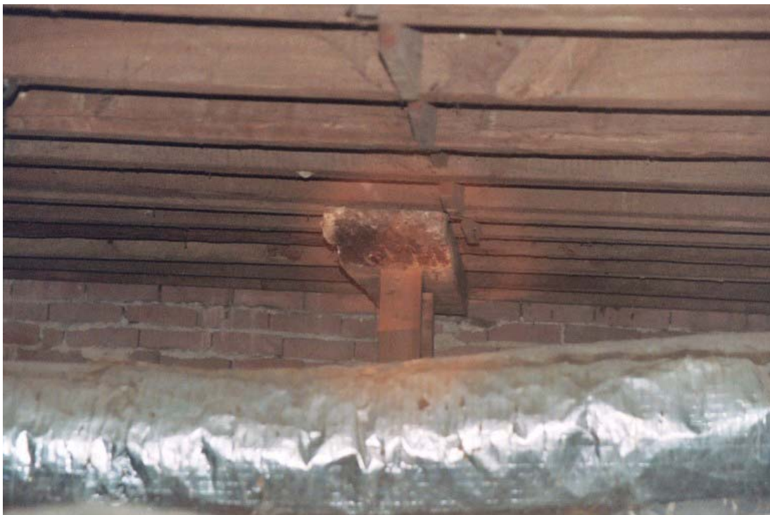
Figure 2 Added supports under northeast room (Room 101)
