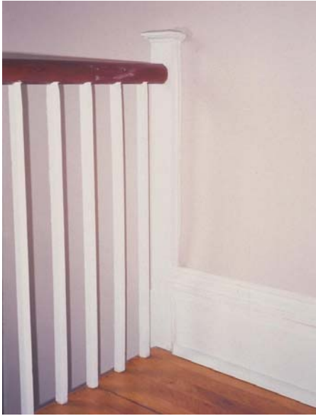
Figure C – 34 Top stair post
