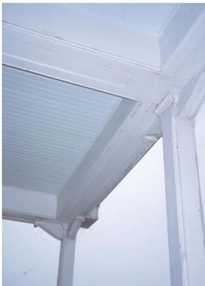
Figure C – 14 Construction of the front porch
