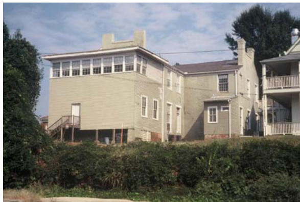
Figure B - 6 Southeast oblique of the house showing two-story frame portion with sleeping porch on second floor
