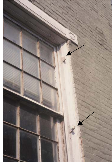
Figure C – 10 Shutter hinges; the upper hinge dating from the second quarter of the nineteenth century, the lower dating from the third or fourth quarter or the nineteenth century
