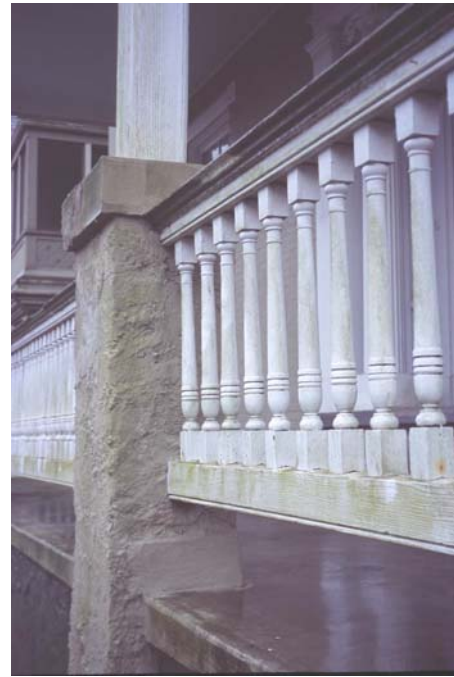
Figure C – 13 Front porch balustrade
