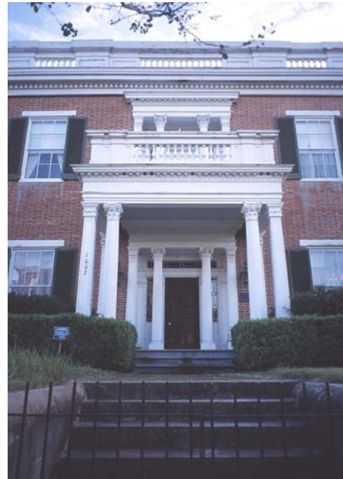
Figure B - 2 Front view of the adjacent Balfour House; it is likely the Willis-Cowan House originally had a similar front porch
