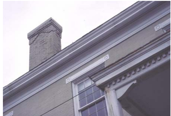
Figure C – 6 Cornice of west porch and original house, and corbelled chimney
