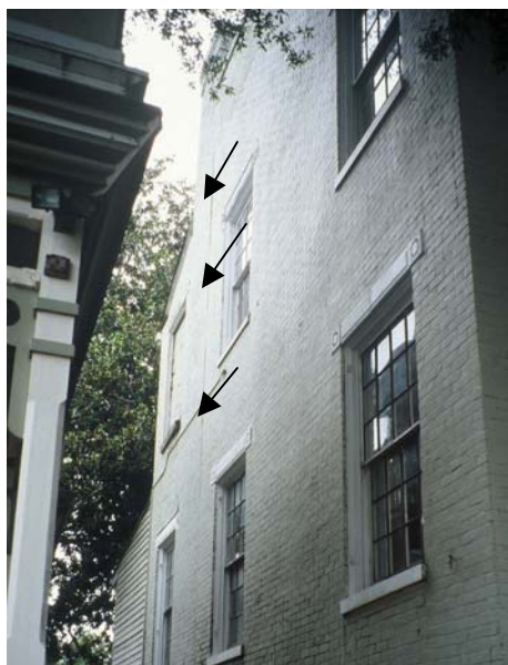
Figure C – 1 Stack joint on east elevation
