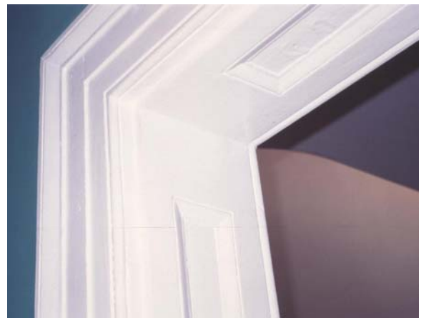
Figure C – 24 Simpler door casing
