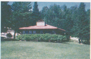
Ellsworth Home Current location of Picnic Shelter (14)
