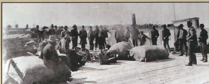
The first cargo of freight being unloaded at the dock at Rainy Lake City. Photo: Koochiching County Historical Society
