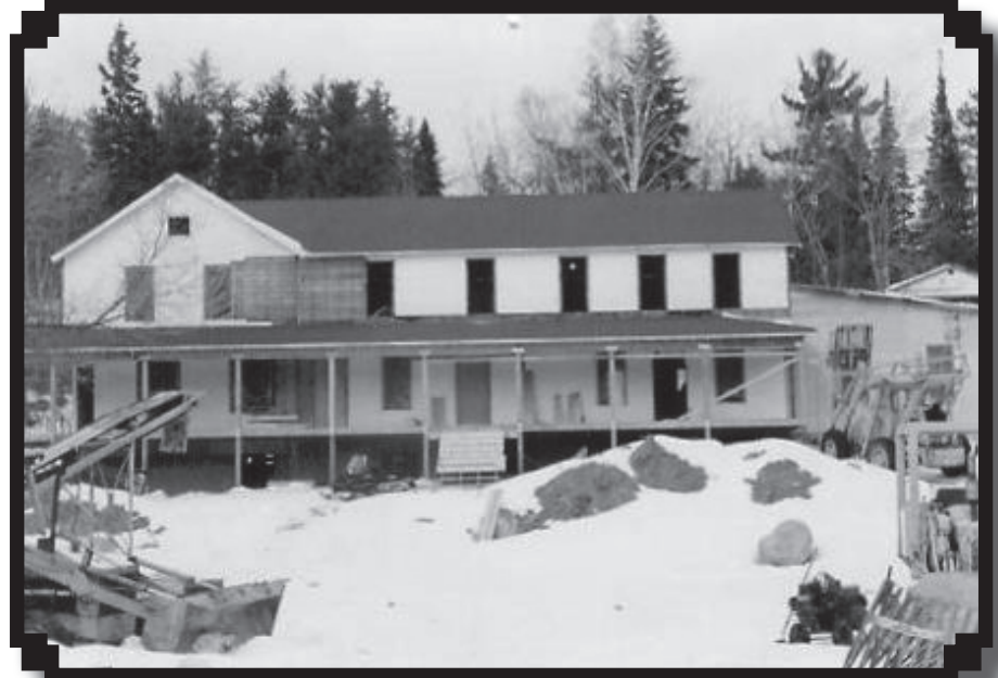
Kettle Falls being renovated, 1986-87, NPS.
