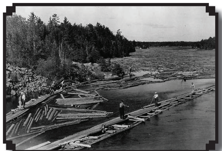
Photo: Sluicing logs through the dam at Kettle Falls, circa late 1930s, Minnesota Historical Society (MHS).
