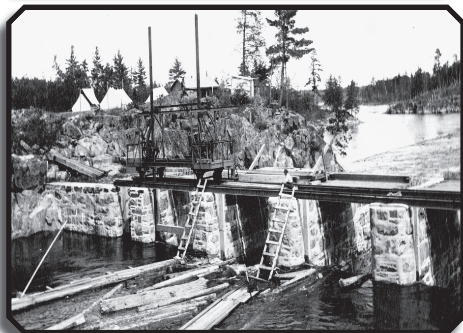
Photo: construction of the dam, 1910 - 1914, NPS.
