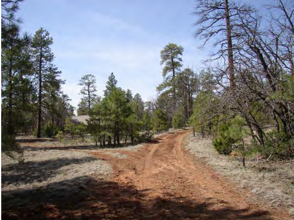
Figure 12. "Old 303" in proximity to Ranger Cabin, 2005 (NPS photo).
