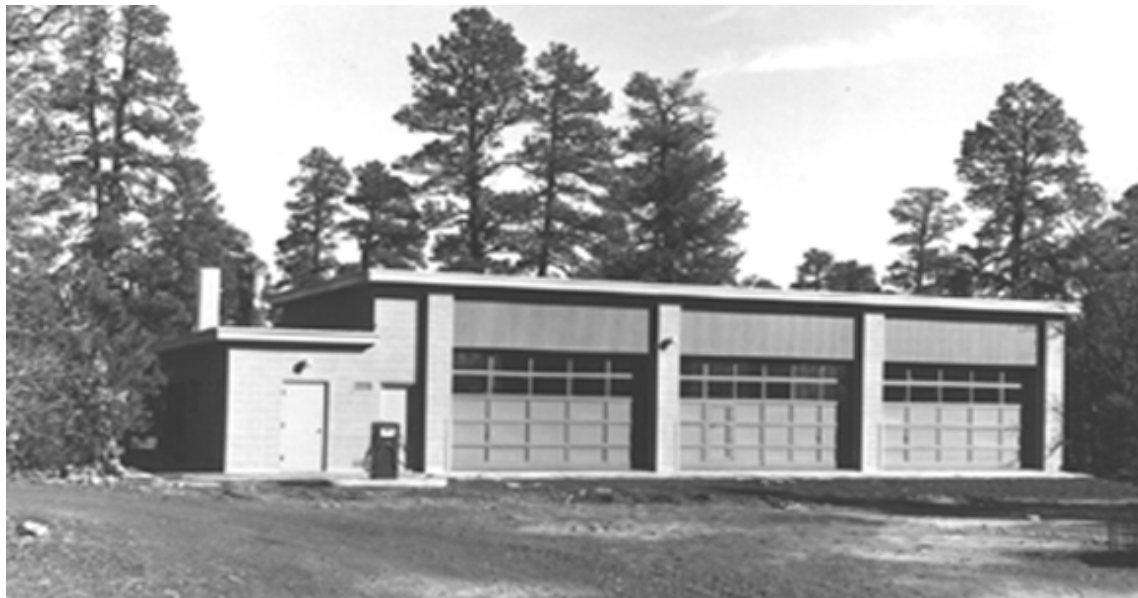
Figure 85. Utility Building after completion, n.d. (NPS photo).
