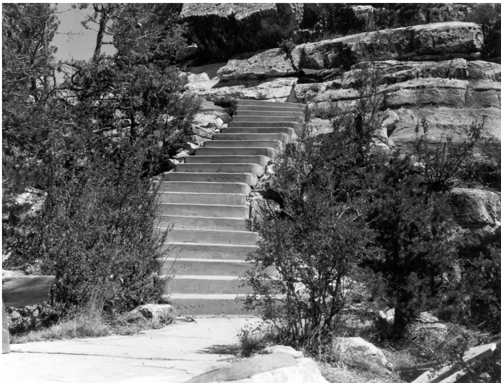
Figure 74. Mission 66 staircase directly above loop level of Island Trail, 1966 (NPS photo).
