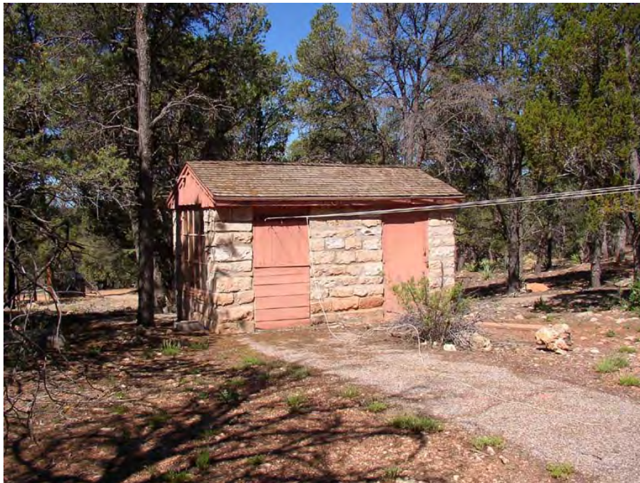
Figure 101. Generator House, 2004 (NPS photo).
