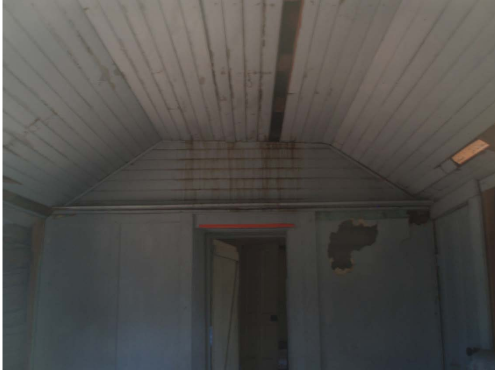
Figure 38. Ranger Cabin Ceiling, 2009. (NPS photo).
