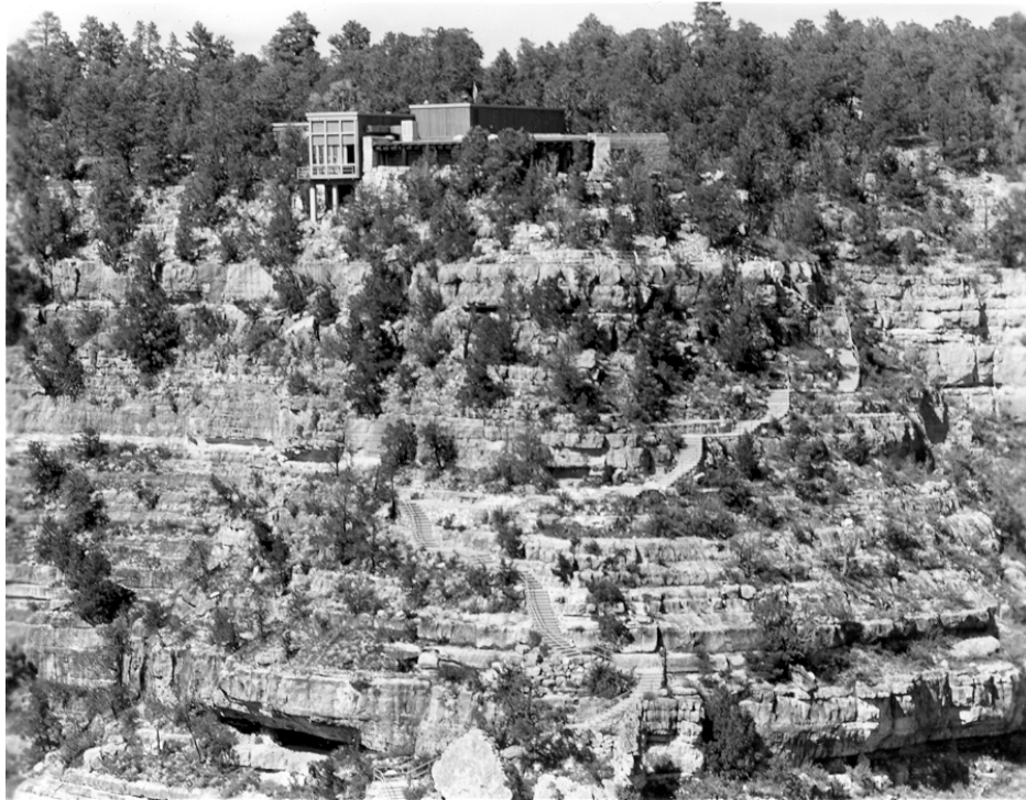
Figure 106. Administration building with Mission 66 addition, c. 1966-1979 (NPS photo).
