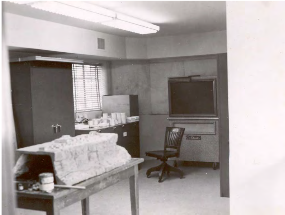
Figure 114. Work room after Mission 66 remodel, 1965 (NPS photo).
