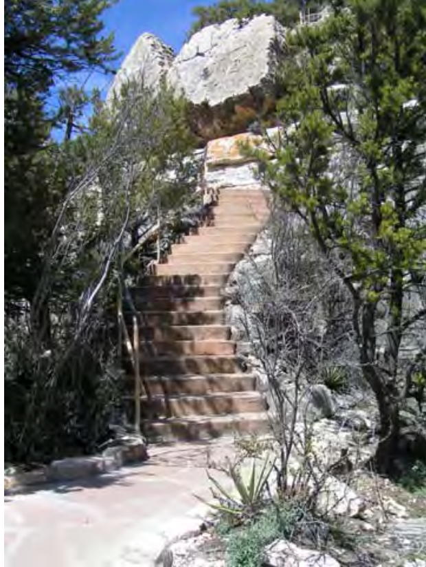
Figure 75. Mission 66 staircase above loop trail, 2005 (NPS photo).
