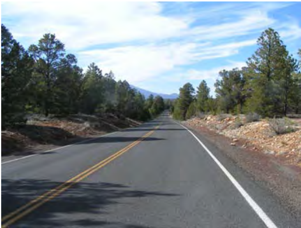
Figure 26. Approach Road, 2005 (NPS photo).
