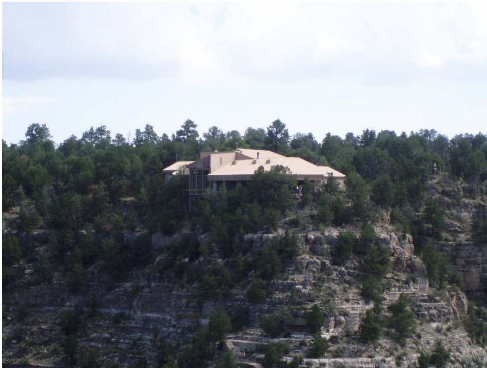
Figure 121. Visitor Center with pitched roof, 2009 (NPS photo), as compared to the structure before the roof in Figure 104.
