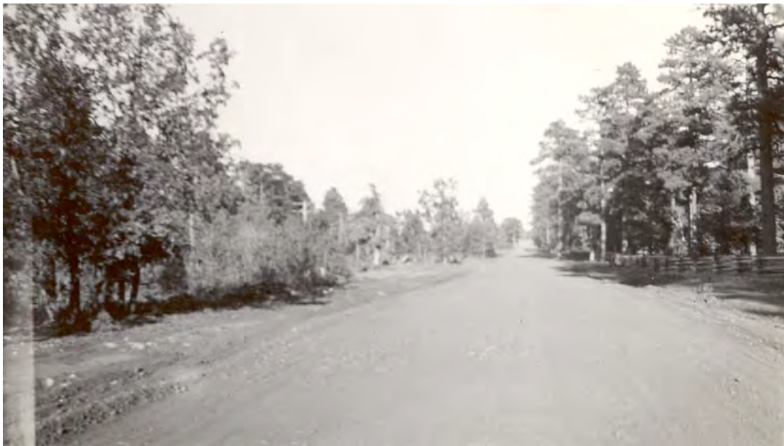
Figure 61. After the construction of the new 303 alignment.
