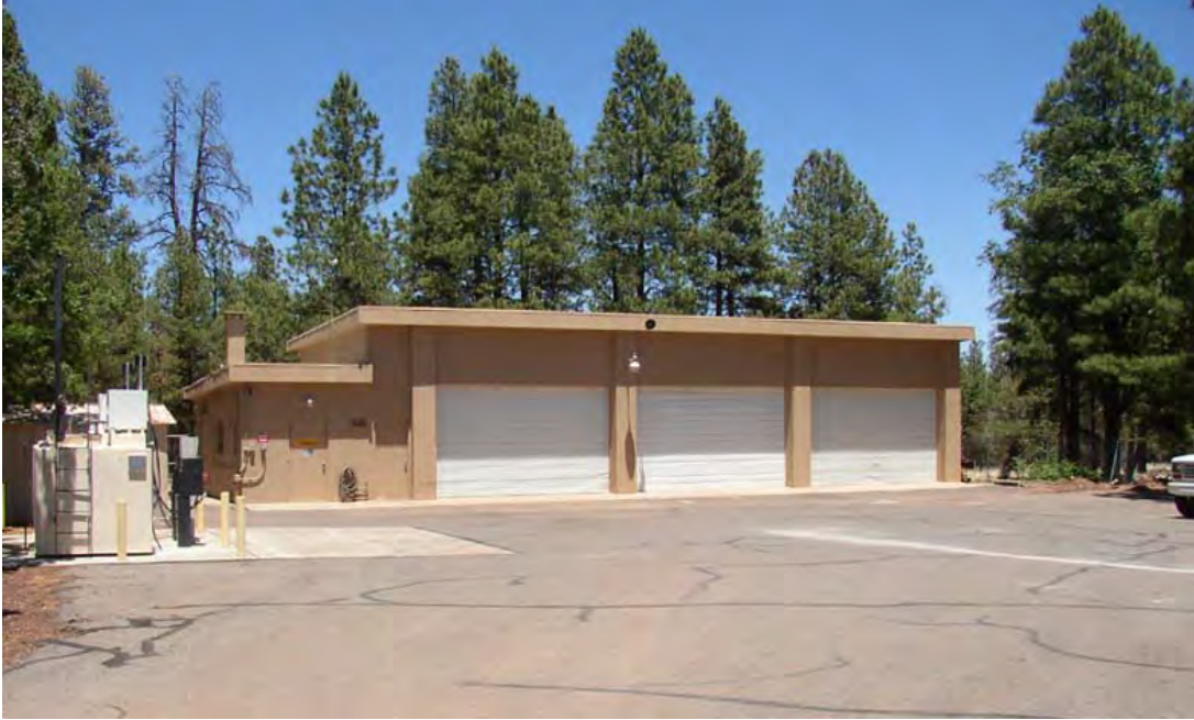
Figure 86. Utility Building, 2004 (NPS photo).
