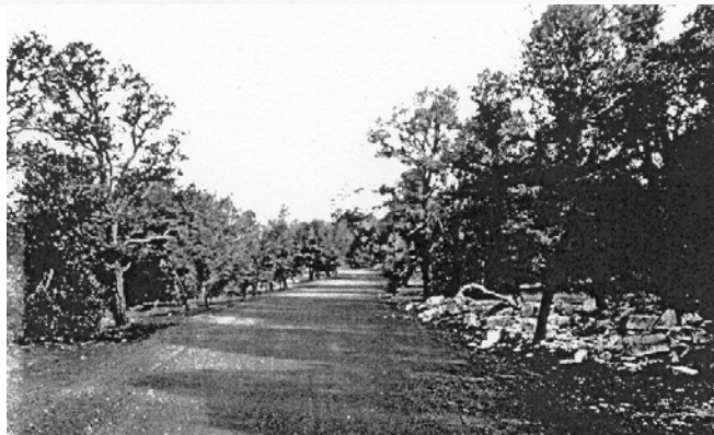
Figure 57. Completed CCC entrance road, 1941 (NPS photos).
