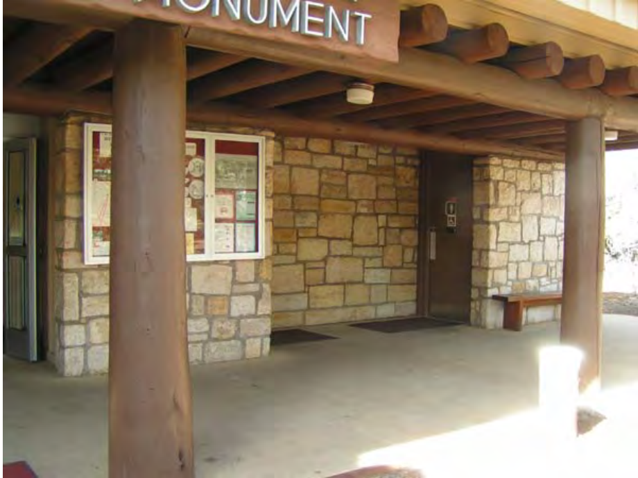
Figure 128. Entrance to restrooms, exterior of Mission 66 Visitor Center, 2005 (NPS photo).
