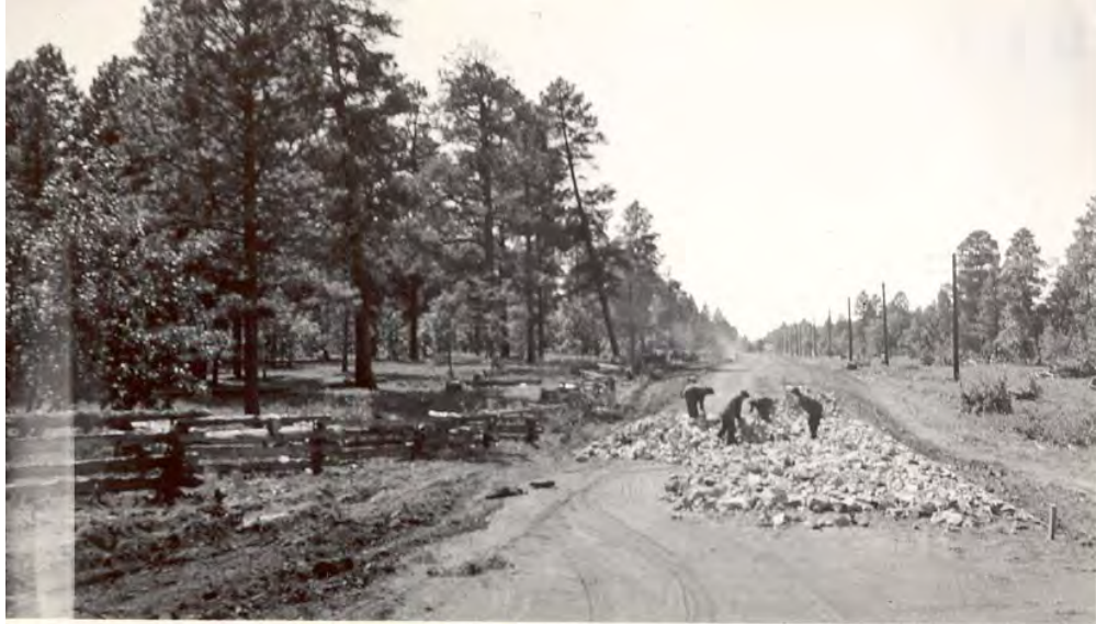
Figure 60. During the construction of the new 303 alignment (NPS photo).
