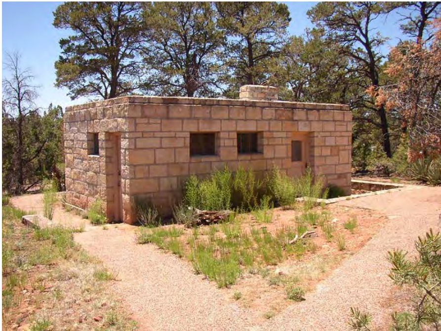
Figure 51. Comfort Station, 2004 (NPS photo).
