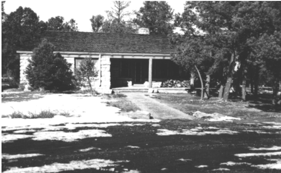
Figure 55. Residence No. 2, date taken unknown (NPS photo).
