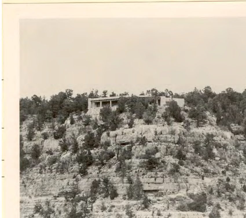
Figure 116. CCC Adminstrative Building, date unknown (NPS photo)
