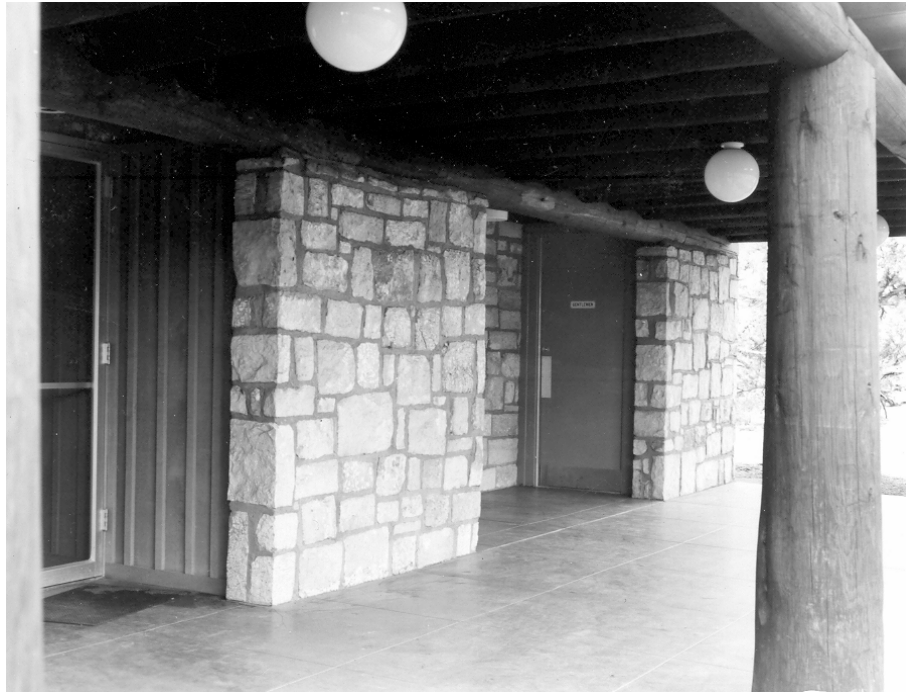
Figure 127. Entrance to restrooms, exterior of Mission 66 Visitor Center, 1965 (NPS photo).
