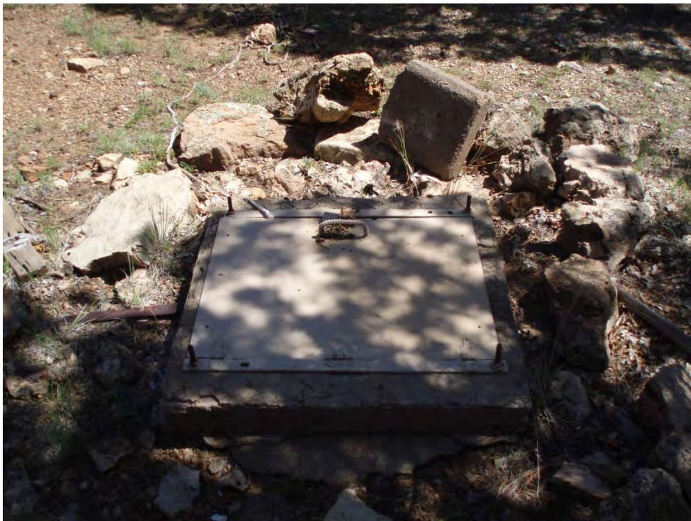
Figure 41. Ranger Cabin Cistern, 2009. (NPS photo).
