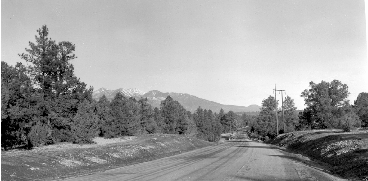
Figure 25. Newly constructed Approach Road, ca. 1956-7 (NPS photo).
