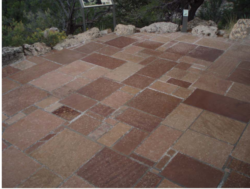
Figure 130. New flagstone on back porch of the Administration Building, 2009 (NPS photo).
