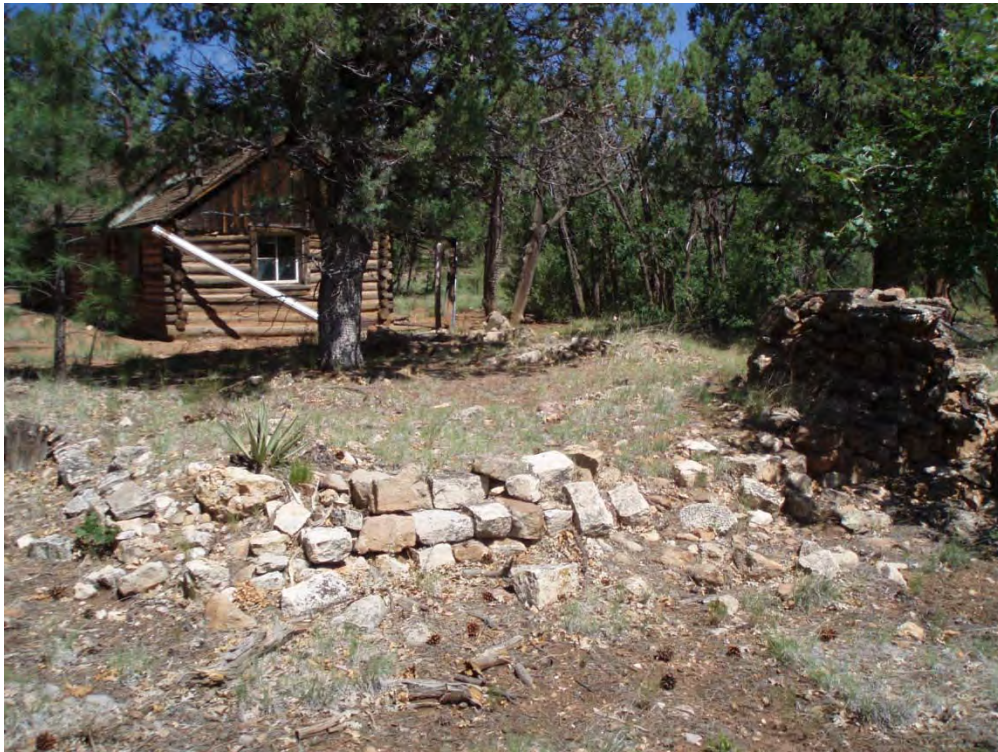
Figure 39. Ranger Cabin Terraced Garden, 2009. (NPS photo).
