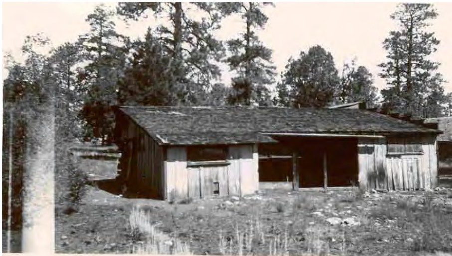
Figure 45. Barn that was near the Ranger Cabin (background right) until approximately 1935, date taken unknown (NPS photo).
