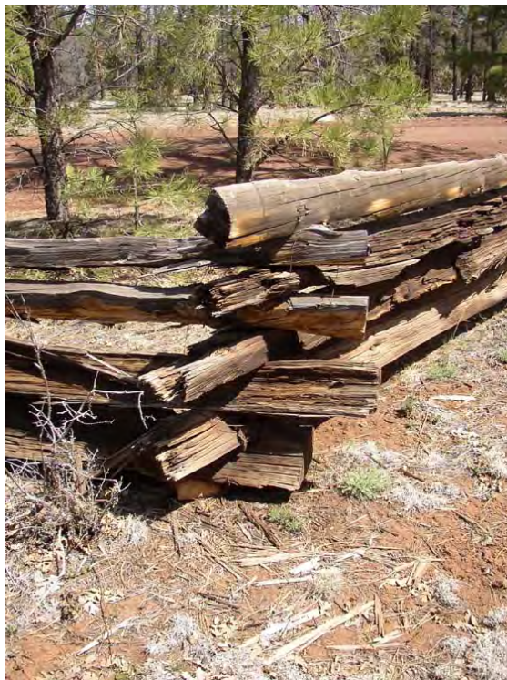
Figure 67. Closeup of worm-rail fence. corner construction, 2005 (NPS photo).
