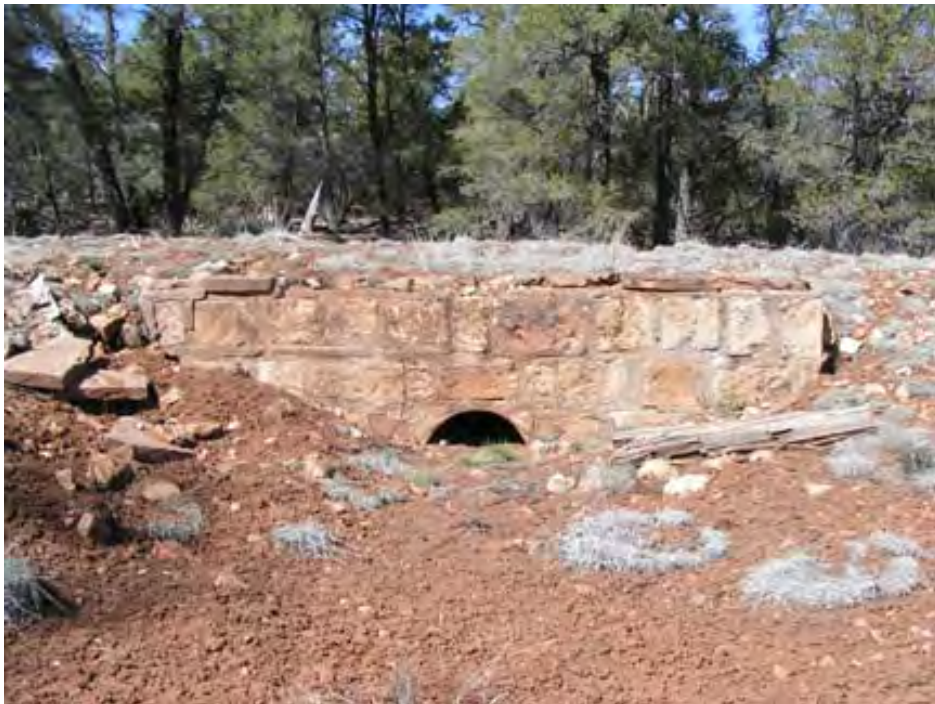
Figure 59. Stone culvert along CCC entrance road, 2005 (NPS photo).
