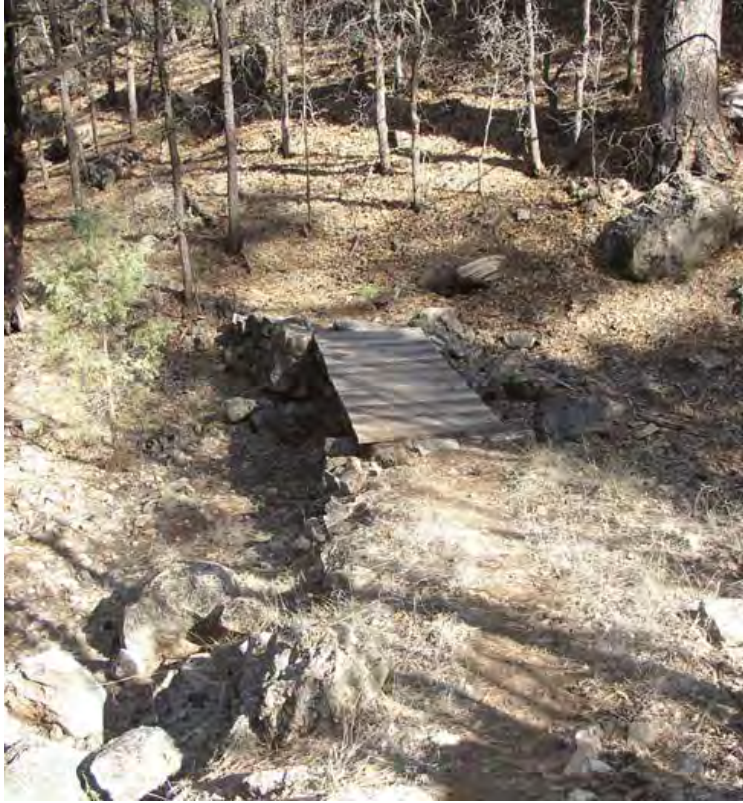
Figure 46. Bridge along canyon section of Ranger Ledge trail, 2002 (NPS photo).
