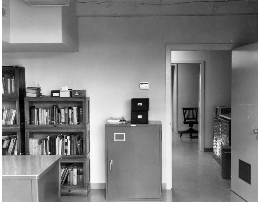
Figure 112. Walnut Canyon Exhibit Room after Mission 66 remodeling into office space, 1965 (note painted wooden viga at the top of the photo) (NPS photo).
