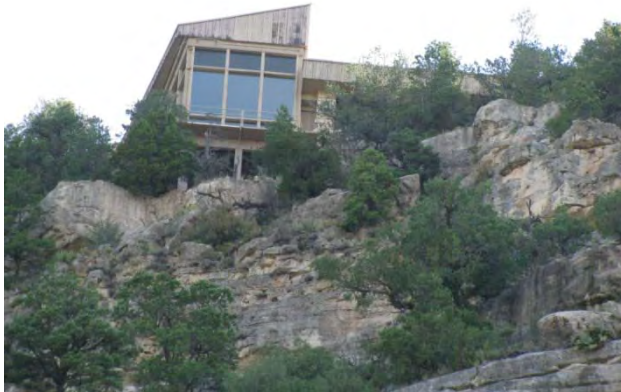
Figure 122. Mission 66 portion of the VC with the pitched roof, taken from within the canyon, 2009 (NPS photo).
