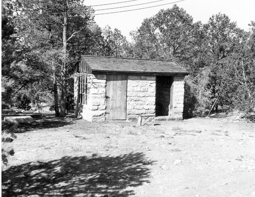
Figure 100. Generator House, 1952 (NPS photo).
