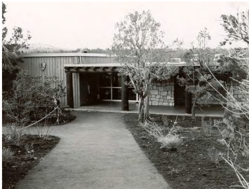
Figure 107. Entrance to Mission 66 Visitor Center ca. 1965 (NPS photo).
