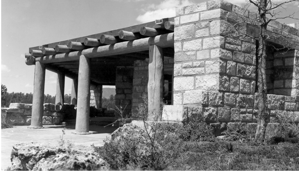
Figure 102. Back Porch of Administration Building, 1942 (NPS photo).
