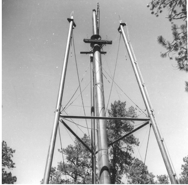
Figure 88. Elevated water tower under construction, 1961 (NPS photo).
