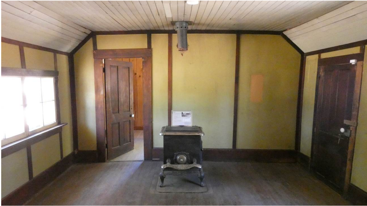
Figure 6. (a) Top, view of Room 3 interior by Paul Beaubien, August 1938, looking northwest. WACA 5530. (b) Bottom, Room 3 as it appeared in 2017, same view. (Photo credit: David E. Purcell).
