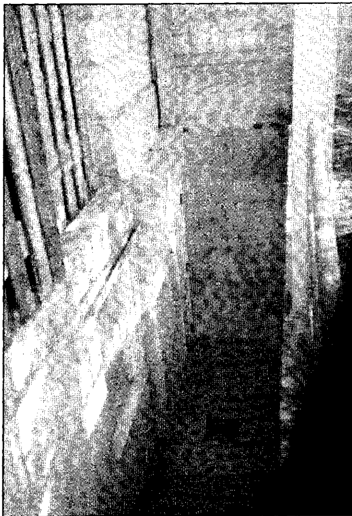
Figure 4.11: Basement areaway, view to southeast.
