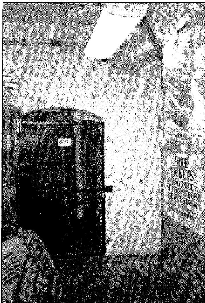
Figure 4.32: Staff locker room, view to southeast with arched doorway into east storage room.
