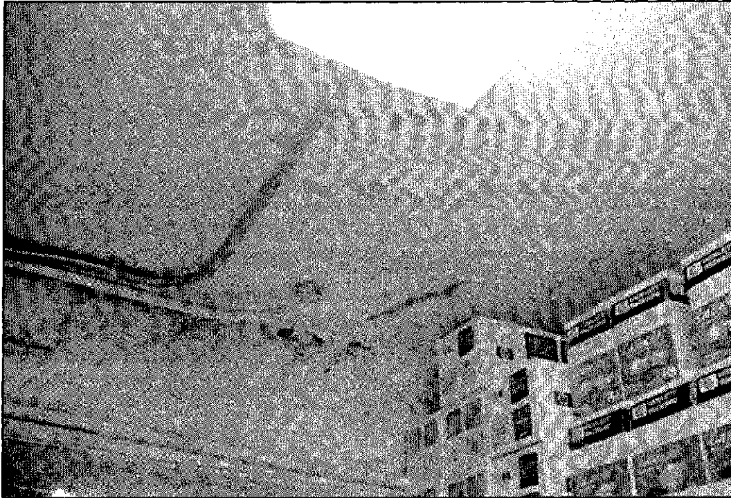
Figure 5.19: Detail of paint failure and water infiltration at concrete ceiling of north storage room. The painted concrete and brick wall at this location has also eroded and is showing signs of rust bloom from embedded ferrous elements.
