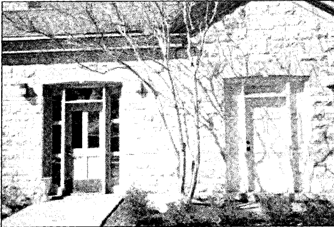
Figure 4.8: Southeast elevation with current entry on left and historic entry on right.
