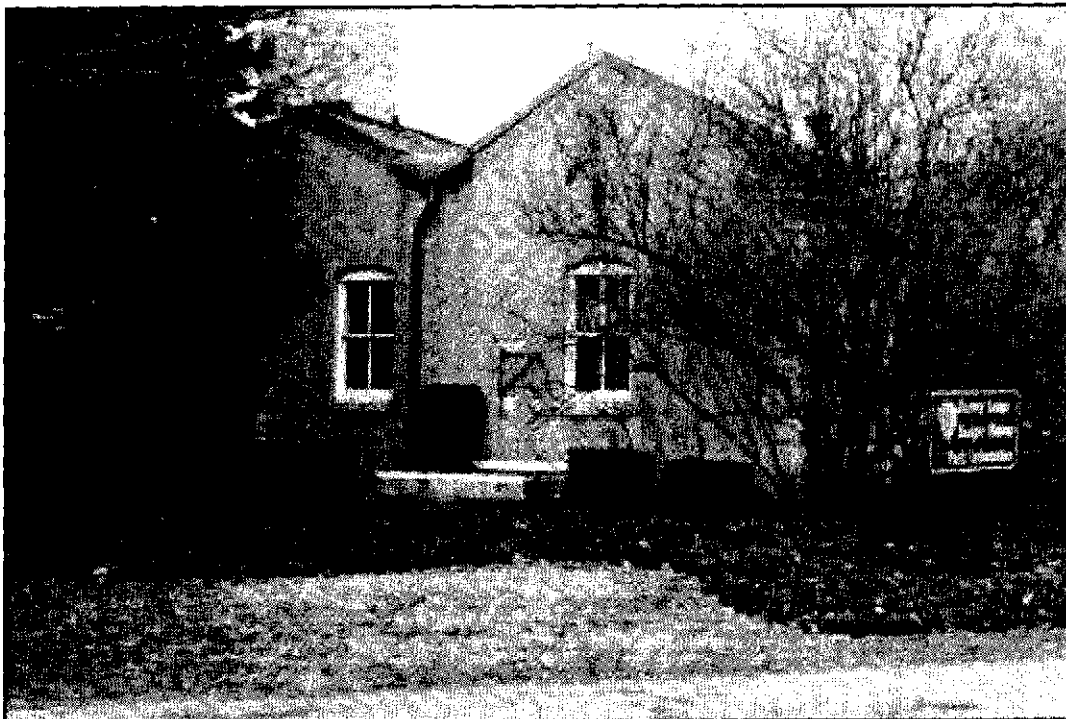
Figure 4.9: Southwest elevation with 1901 stucco addition.
