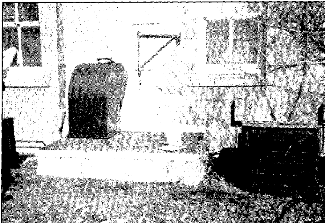
Figure 4.10: Mechanical vault roof.
