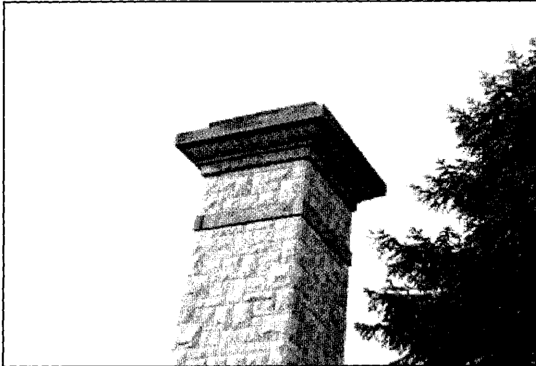
Figure 5.6: Attached chimney, view to the south. The granite belt course has spalled, and the metal chimney cap has stained the granite cornice.
