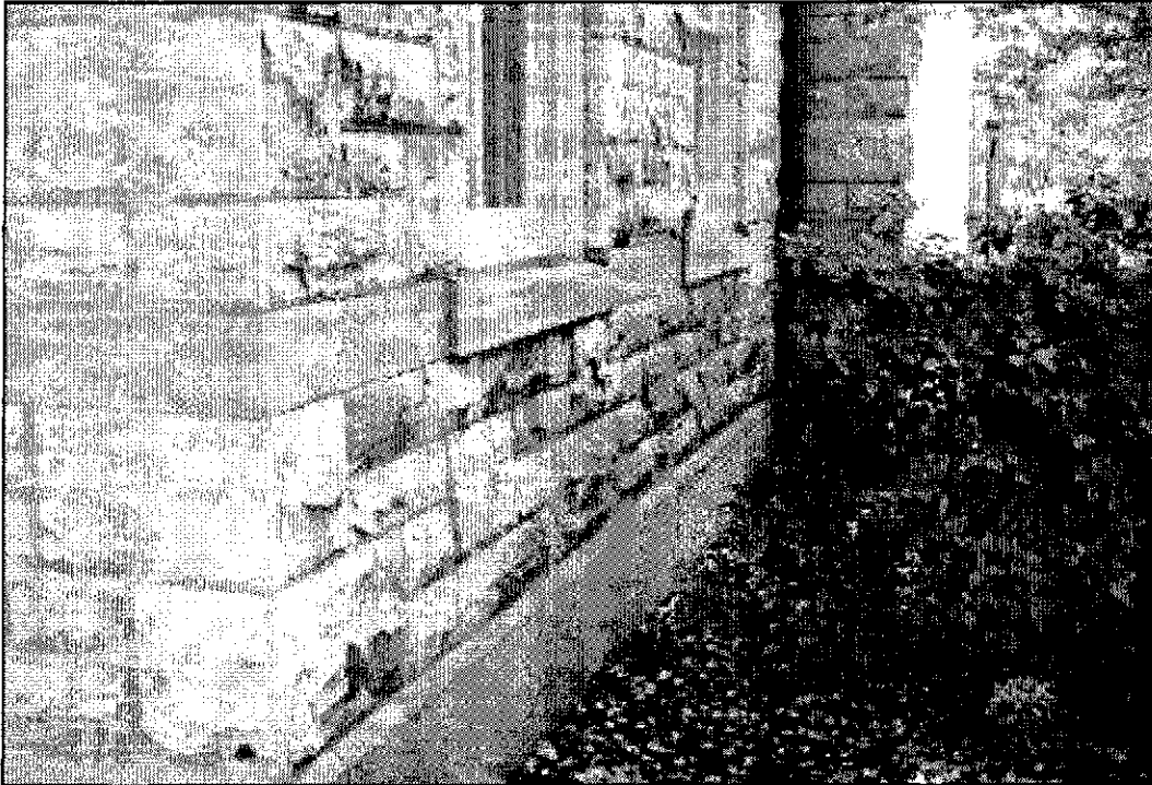
Figure 5.12: Northeast elevation with significant biological growth on underside of rock-faced finish marble and granite water table.
