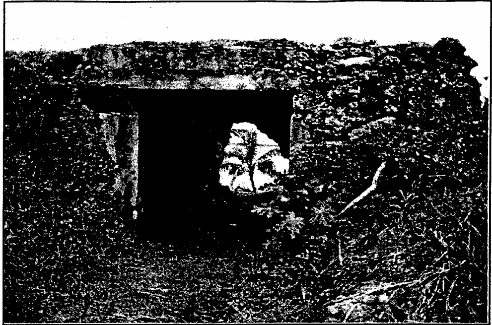
Figure 7. Ruin #23 in 1979. Japanese strong point at Gaan Point. A large reinforced concrete pillbox complex.
