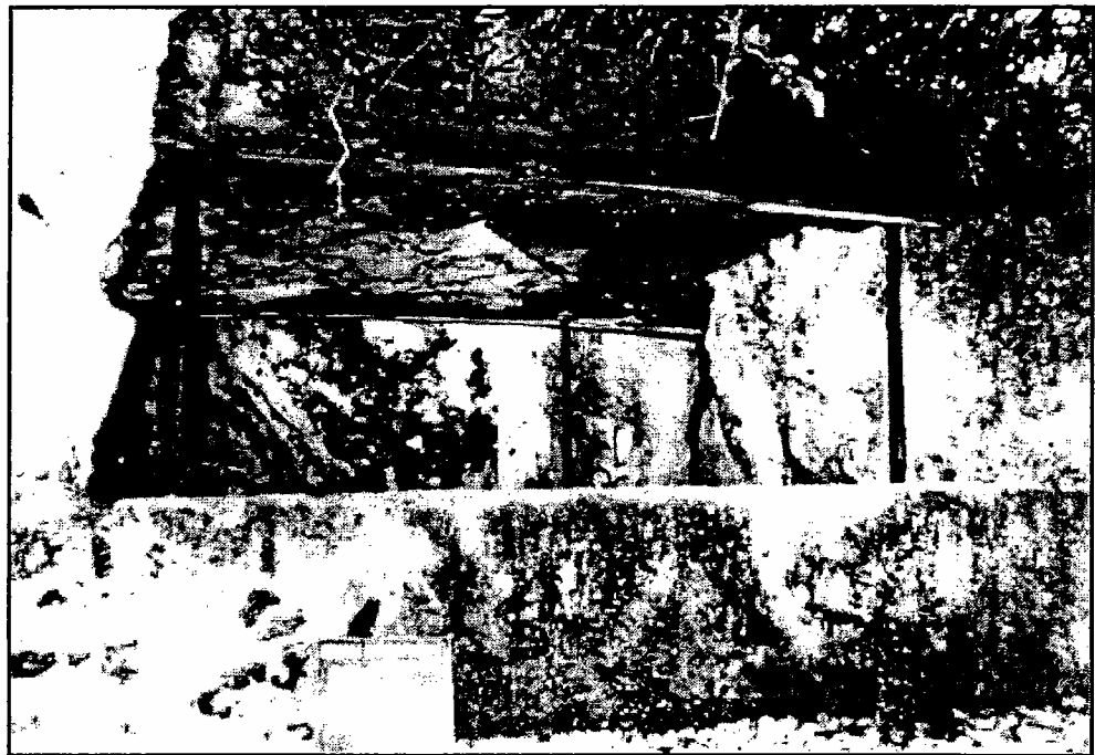
Figure 8. Ruin #62 in 1979. Japanese pillbox of flimsy reinforced concrete, with 150mm gun base.
