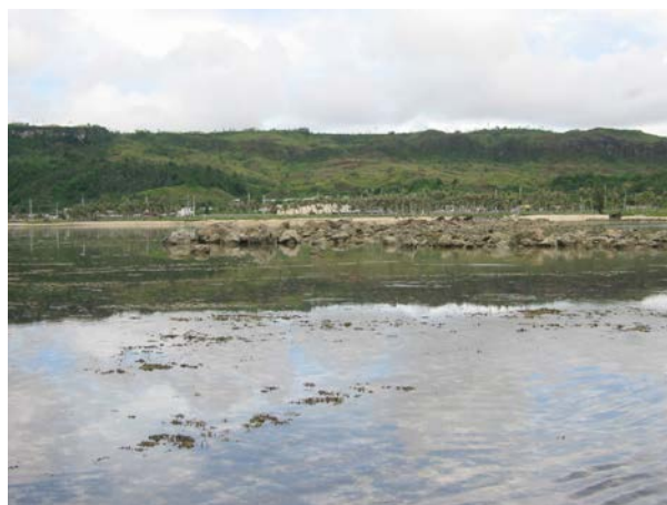
Figure 18. Breakwater feature (rubble in foreground) at Asan Beach Unit constructed by the U.S. Military in an attempt to buffer the sandy shoreline from high wave energy. National Park Service photograph by Deanna Greco (Grand Canyon NP), 2003.
