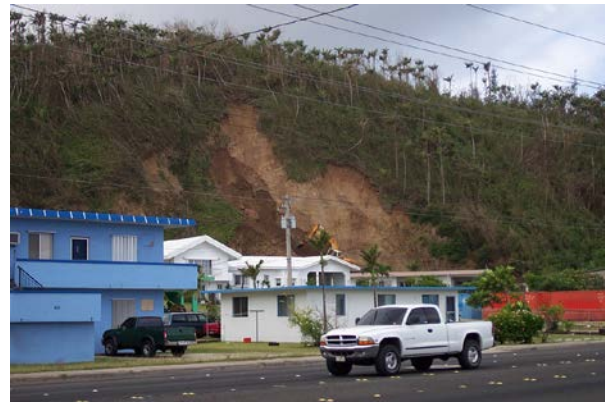
Figure 15. Local resident excavating into the toe of a hillslope failure near the boundary of the Asan Inland Unit (located at the top of the hill). Leaning trees on the hillside suggest long-term, ongoing slump issues at this location. Construction of a retaining wall at the back of the residence did not abate the problem. National Park Service photograph by Deanna Greco (Grand Canyon NP), 2003.
