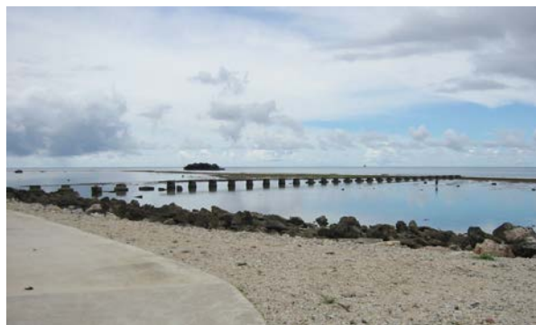
Figure 11. Exposed sewage outfall at Asan Beach Unit. National Park Service photograph by Deanna Greco (Grand Canyon NP), 2003.
