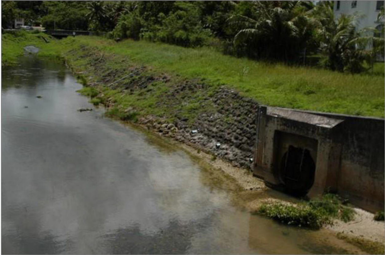
Figure 29. Channelization and streambank modification on the Asan River just upstream of Marine Corps Drive and the Asan Beach Unit. (Photo by T. J. Donaldson)
