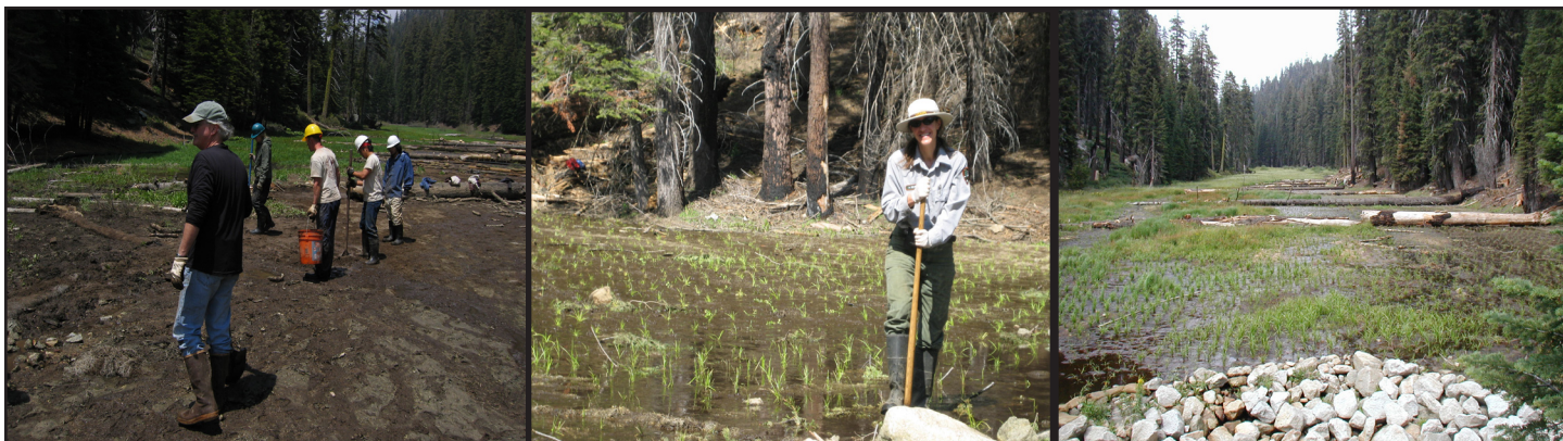
WRD staff and volunteers treating minor erosion channels at Upper Halstead Meadow after a wet winter, Sequoia National Park (Wolf, May 2008).
