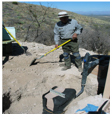
Installing new flow meter at Fort Bowie National Historic Site (Reber, 2008)
