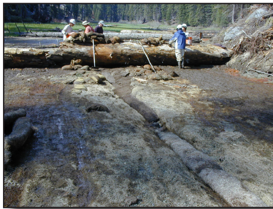
Filling minor erosion channels with coconut fiber logs and dirt, Upper Halstead Meadow, Sequoia National Park (Demetry, May 2008). Large logs were placed in 2007 to slow water flow.
