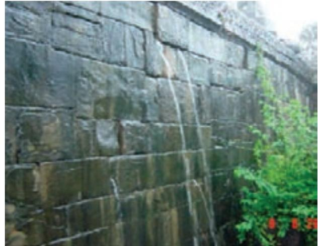
*Stormwater leaking through wall joints in the bottom tier after a prolonged rainfall (photo courtesy of the Authority for the Protection and Management of Angkor and the Region of Siem Reap). ♣*
