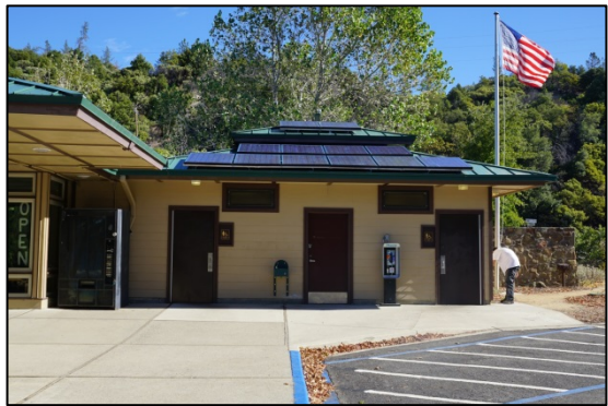
Image 6: Restroom addition. Image looking northeast.
