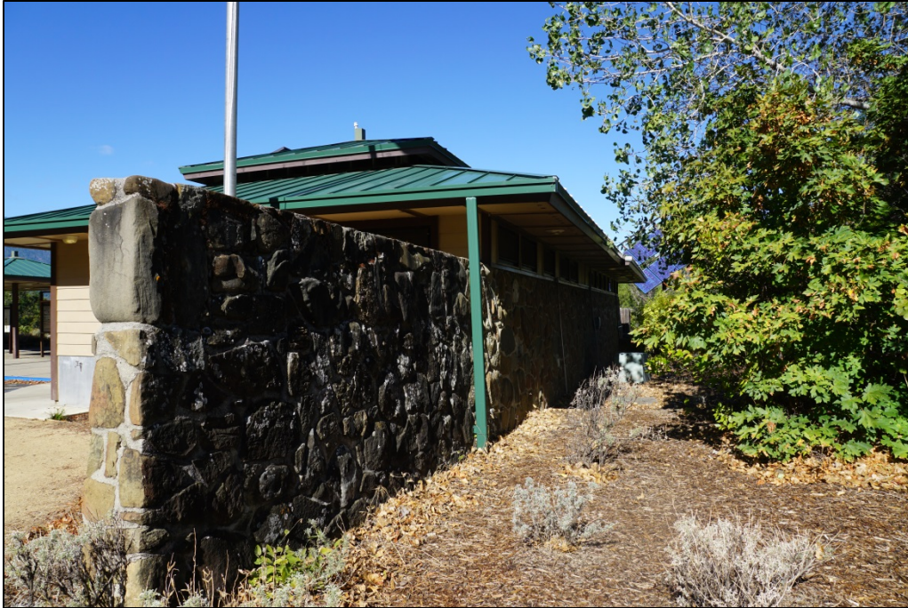
Image 27: Stone wall extension beyond addition. Differentiation in stone color is visible. Photo by Ashley Phillips, 2016
