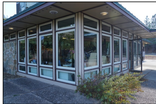
Image 4: Window Wall on Visitor Center. Image looking east.
