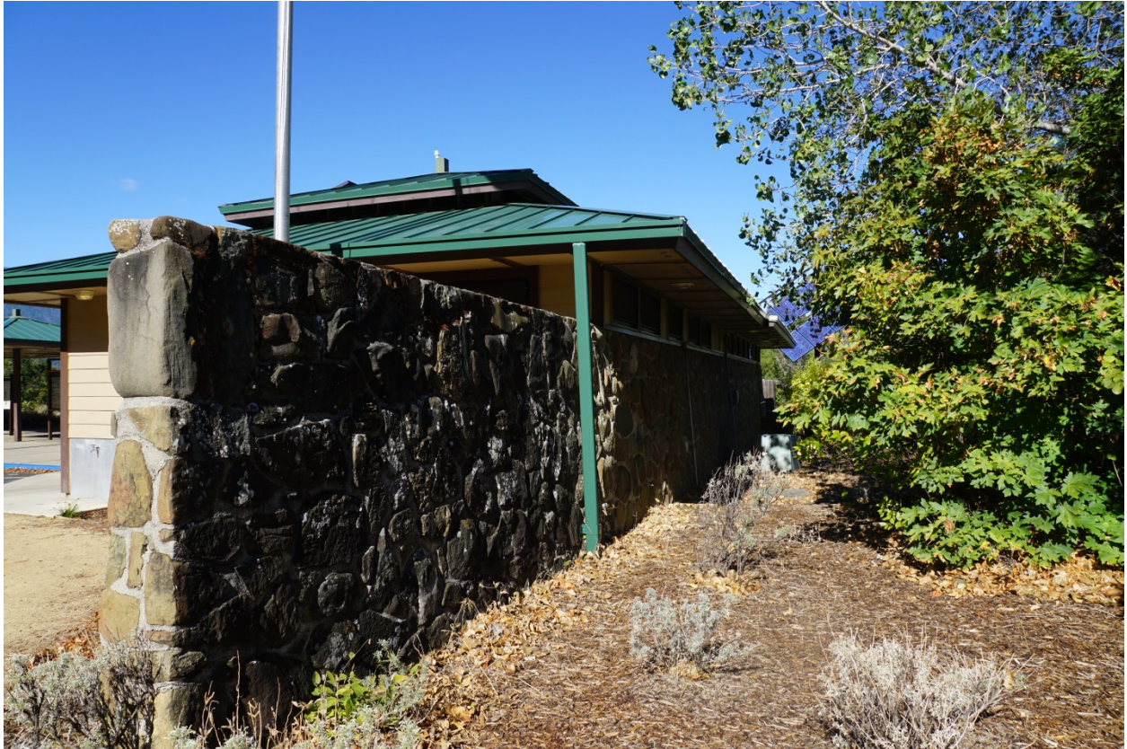
Image 33: Stone wall on northeast corner. Darker stone on non-historic portion is visible. Image looking west. Photo by Ashley Phillips.
