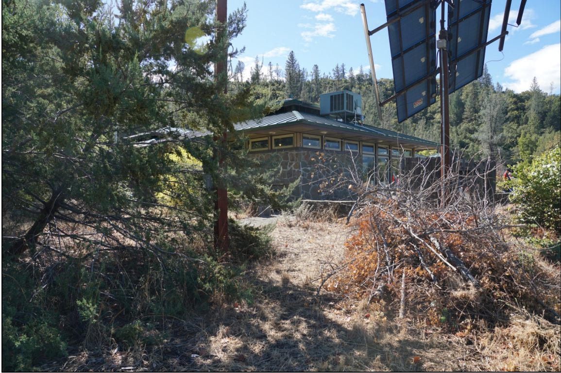
Image 23: Looking south. Image shows northwest corner of the main lock, solar panel, and fenced-in propane tank (obscured behind branch pile). Photo by Ashley Phillips, 2016.
