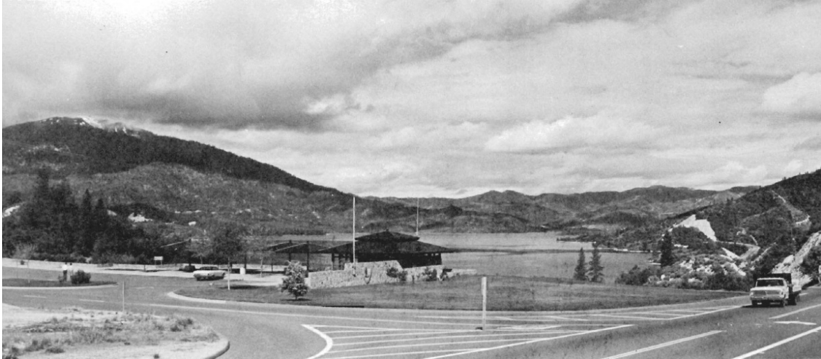
Image 15: Visitor Center Site circa 1972. Note the historic location of the flagpole and NPS arrowhead on the stonewall. Image looking west. Source: National Park Service, Master Plan for Whiskeytown National Recreation Area , Denver Service Center.
