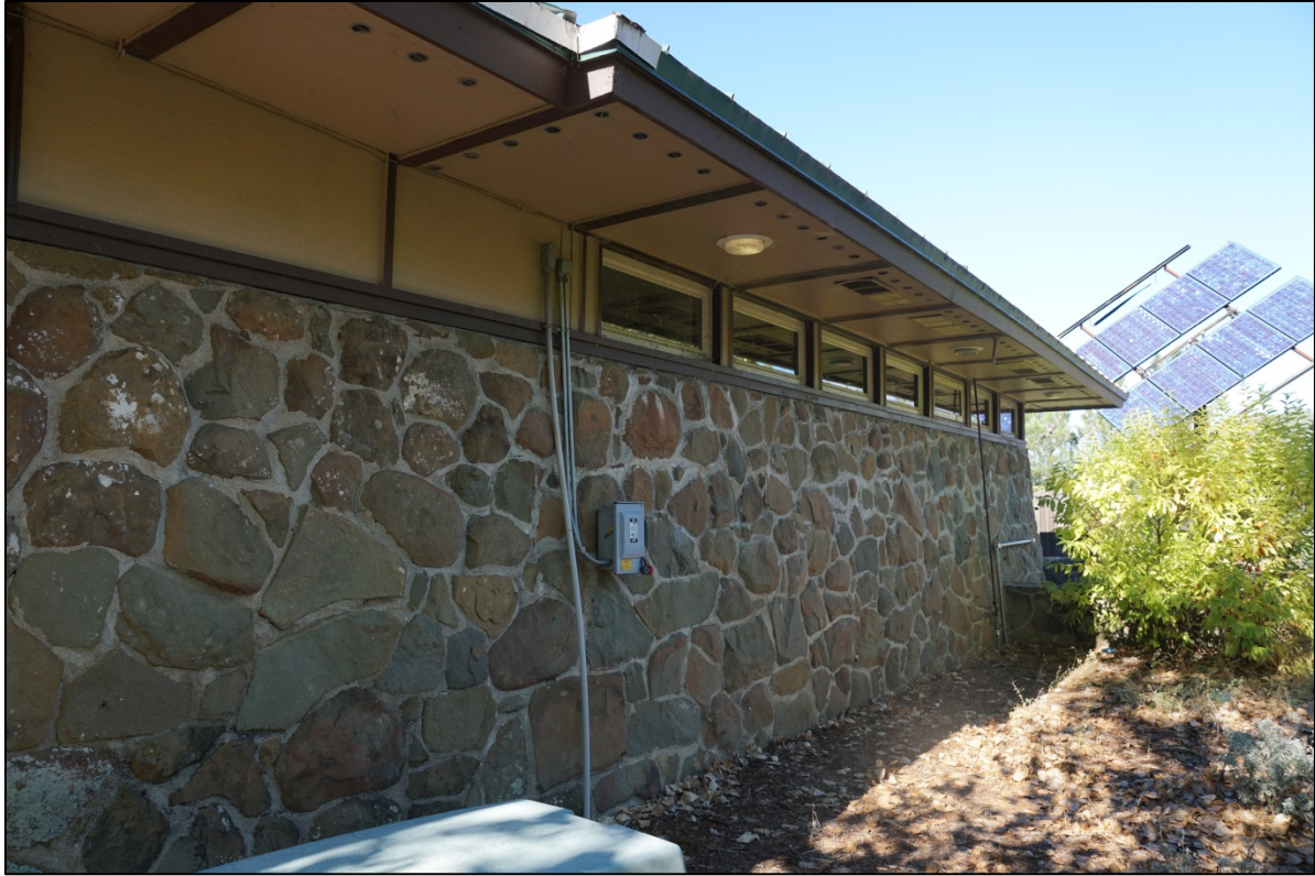
Image 22: Rear wall showing mortared stone work and pole mounted solar panel in the northwest corner. Photo by Ashley Phillips, 2016.
