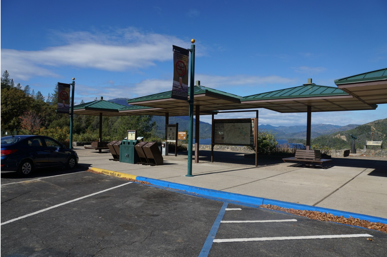
Image 32: Courtyard view from the parking lot. Image looking west.
