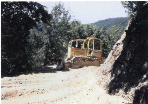
Outsloped roads help water to run off naturally.
