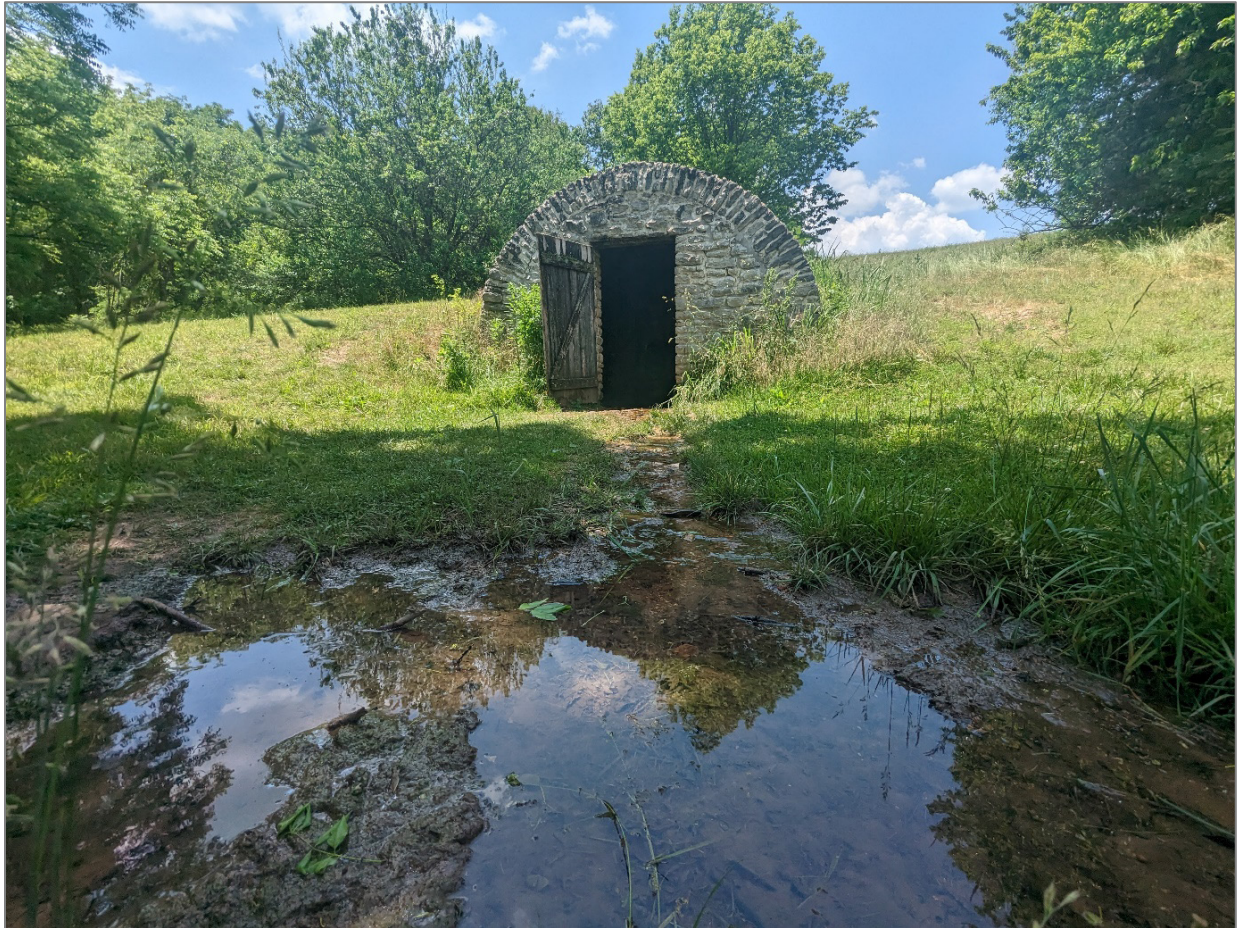
Figure 9. Photograph of spring water flowing out of the Ray Springhouse. The springhouse was built into a hillside and has a curved roof and sides with a front and back wall. The water flows toward a small, unnamed drainage and continues to join Wilson’s Creek near the Pulaski Arkansas Battery site. COLORADO STATE UNIVERSITY / MICHAEL BARTHELMES
