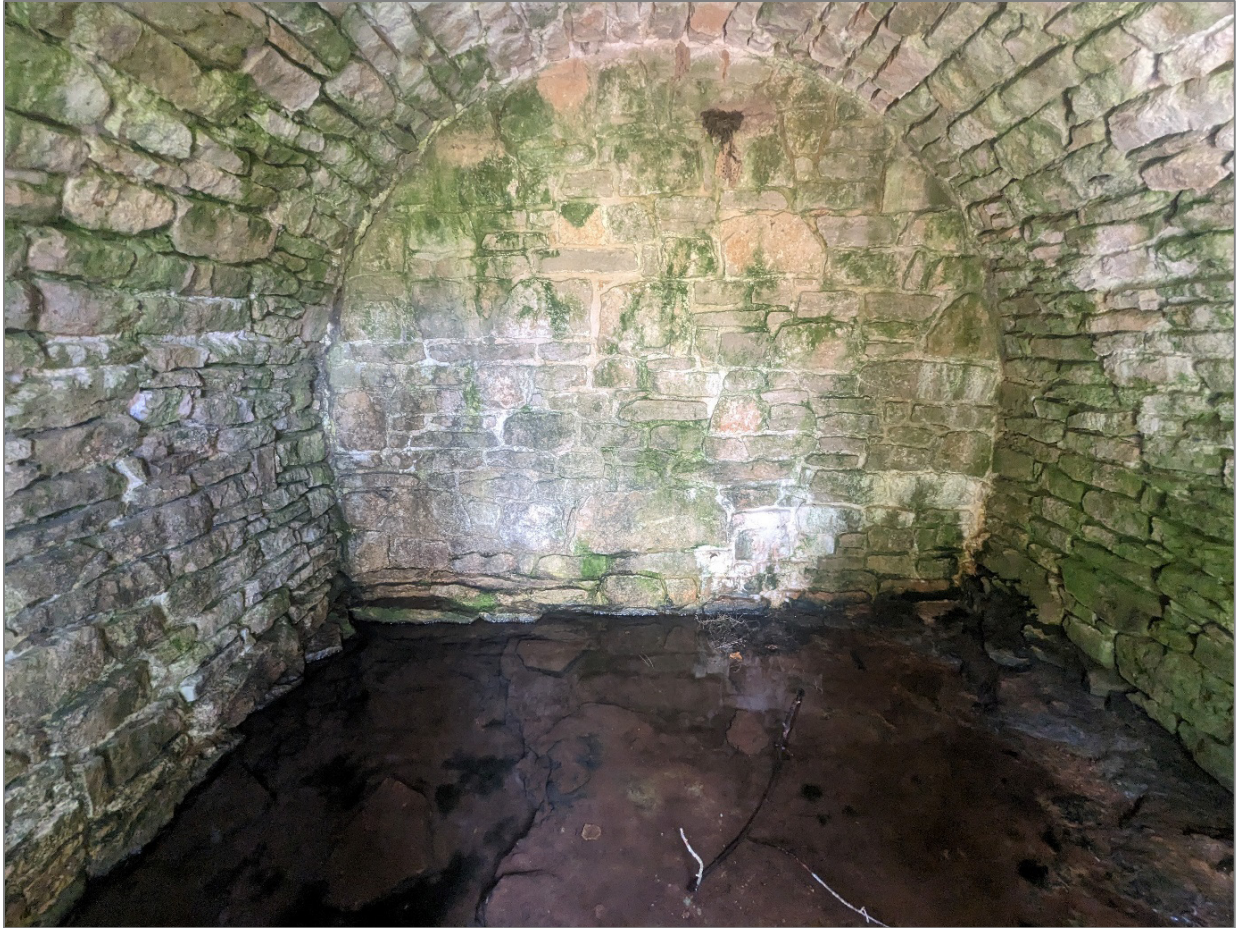
Figure 3. Photograph of Ray Springhouse interior. Constructed entirely of locally quarried Burlington-Keokuk limestone, the springhouse partially impounds a spring and, using the cool temperature of the spring water, provided a place for the Ray family to store food. The spring was also a source of fresh drinking water for the family and their animals.
