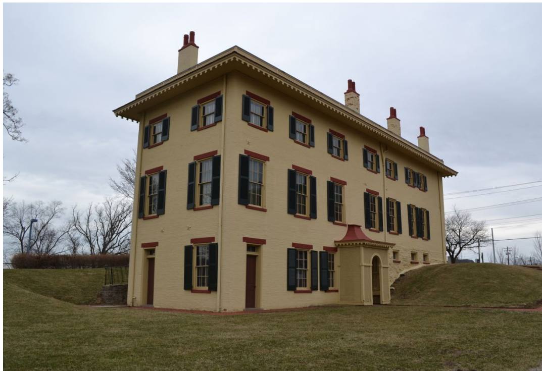
WILLIAM HOWARD TAFT HOME, Cincinnati, Ohio North and East (rear) elevations Photo by Liz Sargent, March 2014
