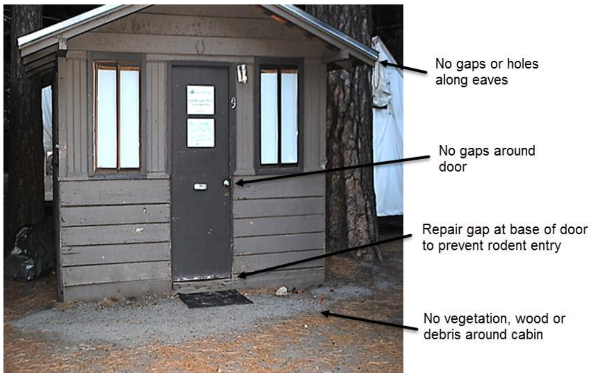
Figure 4: Additional points to evaluate on a cabin include gaps around eaves or door and the presence of vegetation, wood, or other debris around the foundation of the cabin. Figure credit: Bruce Badzik.
