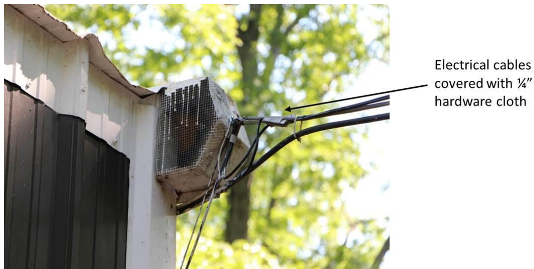
Figure 12: Electrical cables covered with \frac{1}{4} " hardware cloth at the cable/roof junction to exclude rodents at the cable entry point. Figure credit: NPS Figure.
