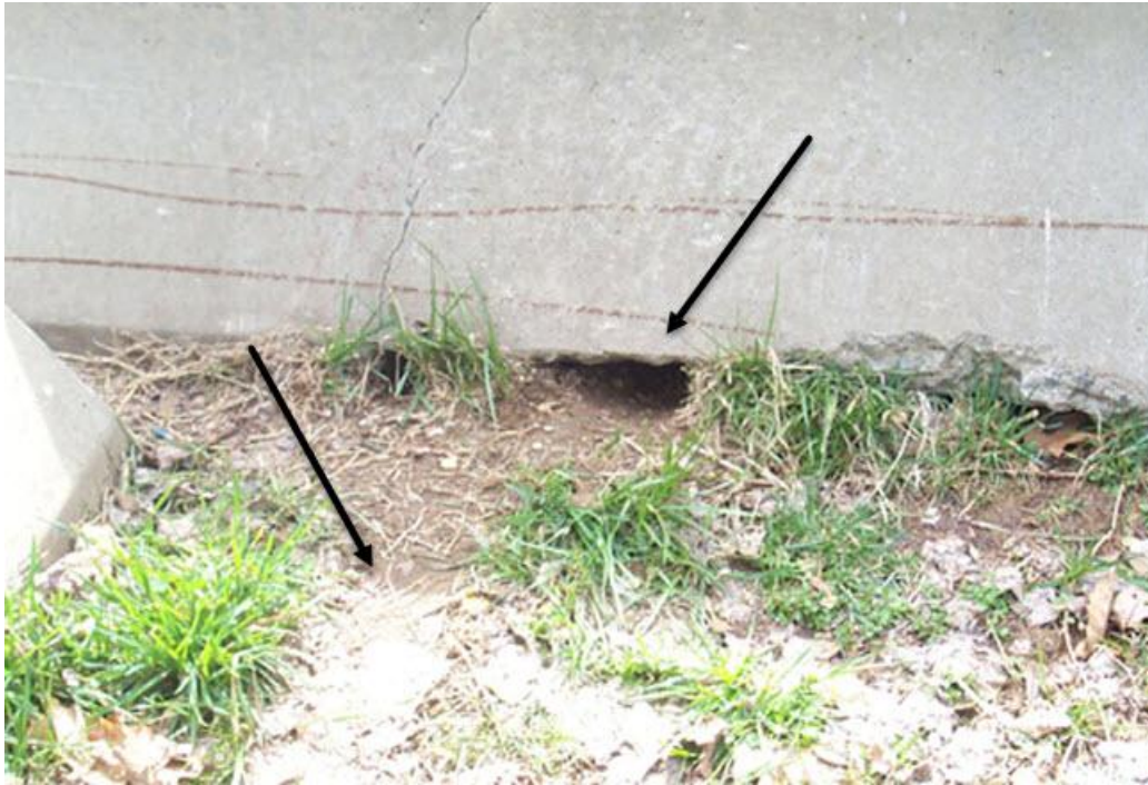
Figure 28: This active rodent burrow is located at the foundation of the building. Note the entrance and runway is clear of vegetation and the rodent has created a “run”. Figure credit: NPS Figure.
