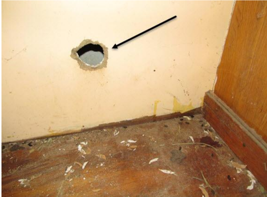
Figure 26: Pack Rat ( Neotoma sp.) entrance hole. Figure credit: Charles Conner.
