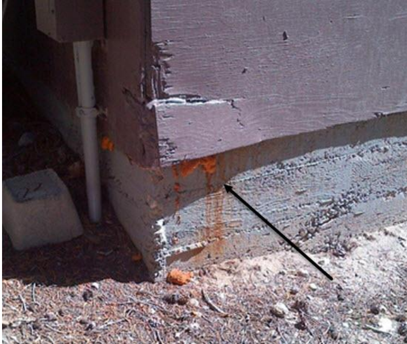
Figure 30: Expanding foam can be used to fill gaps. This foam must be trimmed and painted once dry to protect it from breaking down or becoming brittle in the sun's UV rays. Figure credit: NPS Figure.
