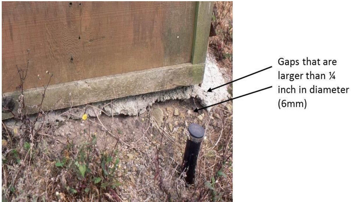
Figure 6: This foundation has a gap between the foundation and building providing potential rodent access into the building. Figure credit: NPS Figure.
