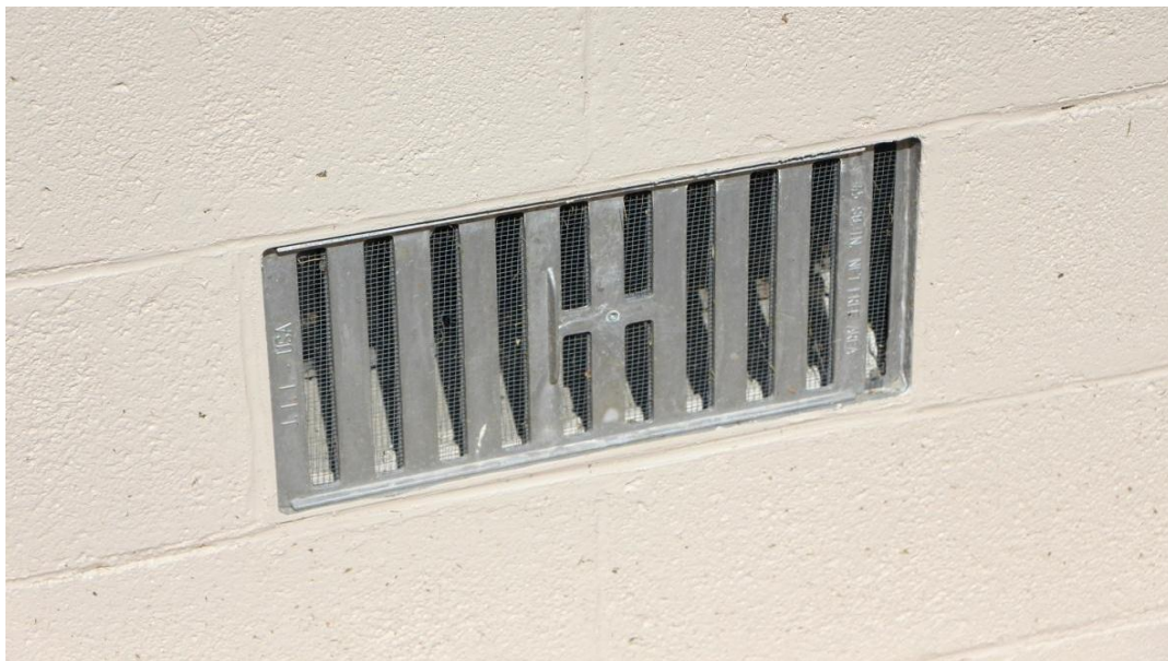
Figure 7: This crawl space vent is properly screened with 1/4" hardware cloth (visible behind the metal bars). Figure credit: NPS Figure.
