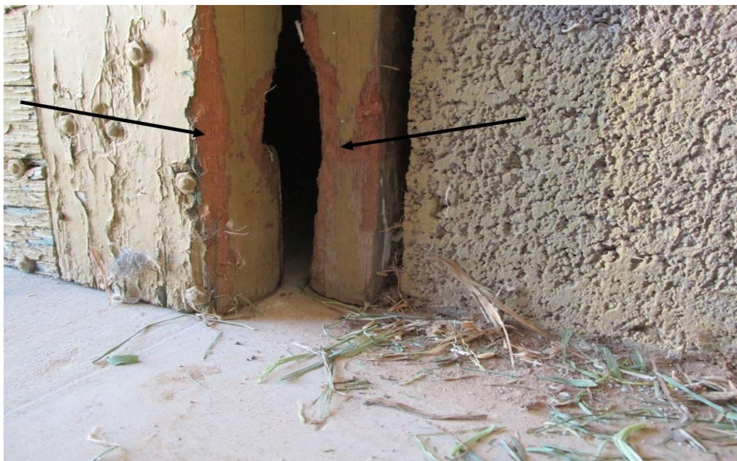
Figure 19: Evidence of packrat gnawing activity. Figure credit: NPS Figure.
