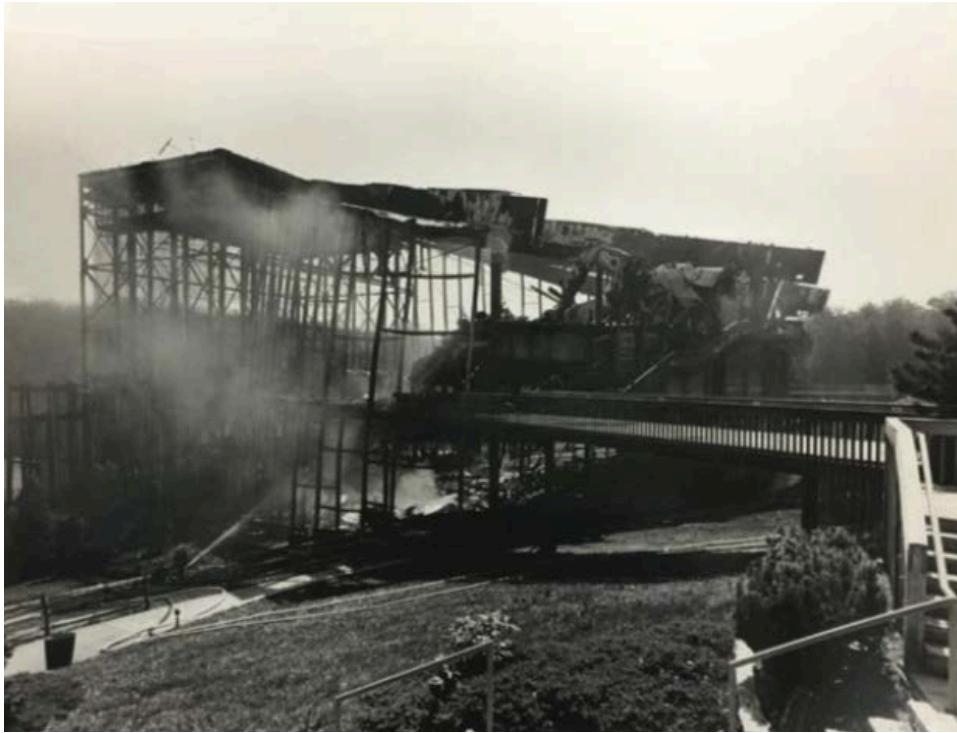
Figure 19. Aftermath of the fire, April 5, 1982 (source: Museum Resource Center NCRO B117 F1982-3).
