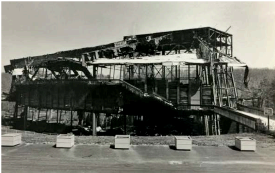
Figure 18. Aftermath of the fire, April 5, 1982 (source: Museum Resource Center NCRO B117 F1982-3).
