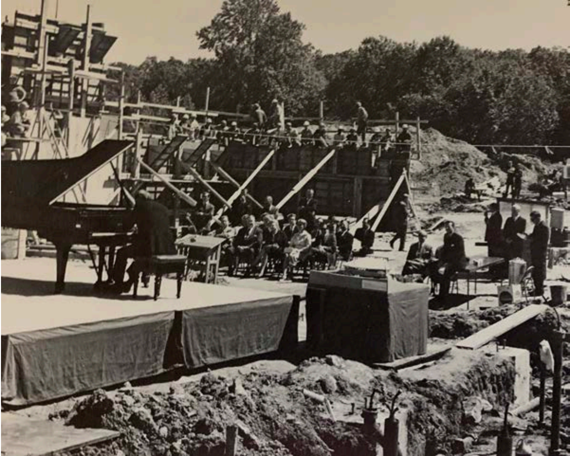
Figure 11. September 11, 1969: A concert by pianist Lorin Hollander took place during the construction of the Filene Center to help fund the Wolf Trap Foundation. It appears that the work at this point encompassed the foundation and utilities (source: Museum Resource Center, NCRO B117 F1969-71).
