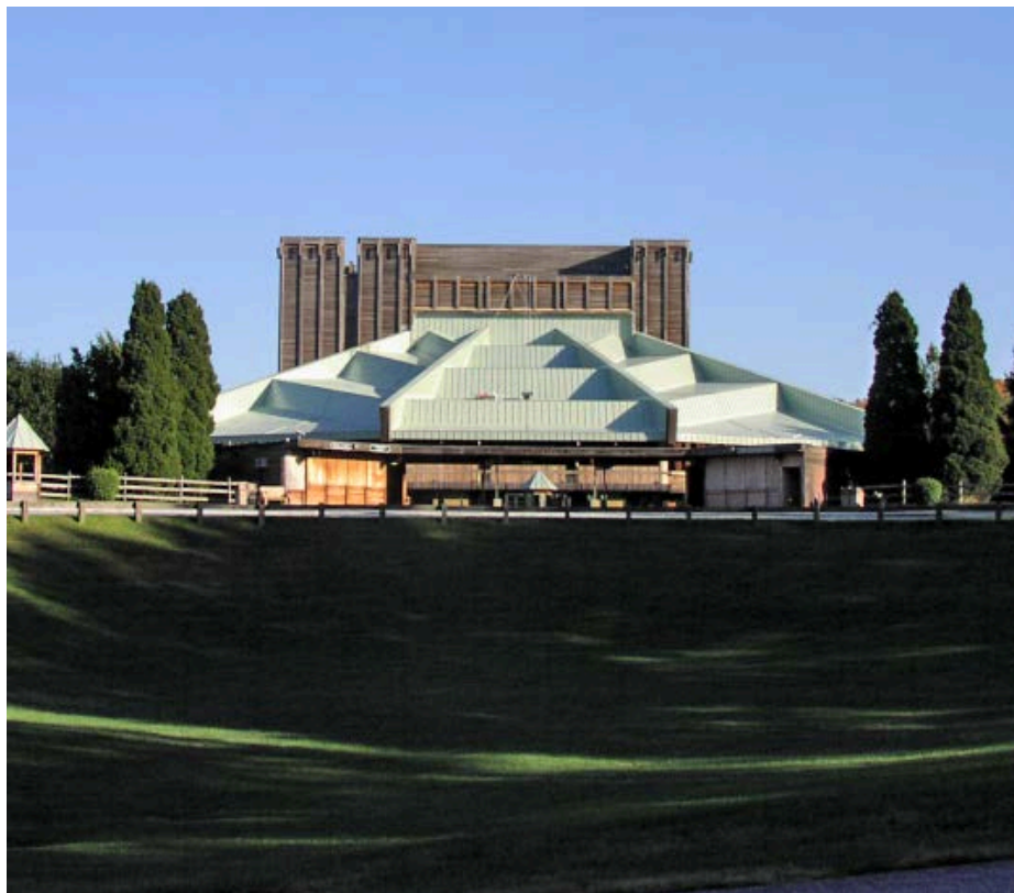
Figure 22. Photo of Filene Center II (2010 LRIP).
