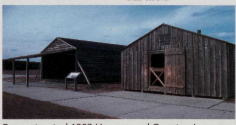
Reconstructed 1903 Hangar and Quarters/Workshop
