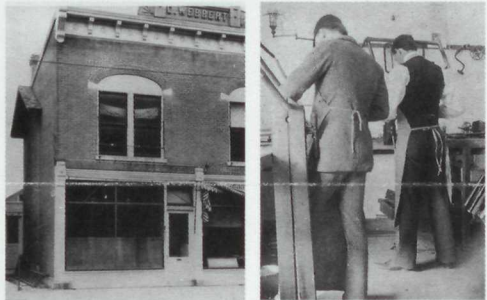
The Wright Cycle Company occupied part of this building in Dayton, Ohio, where Orville
