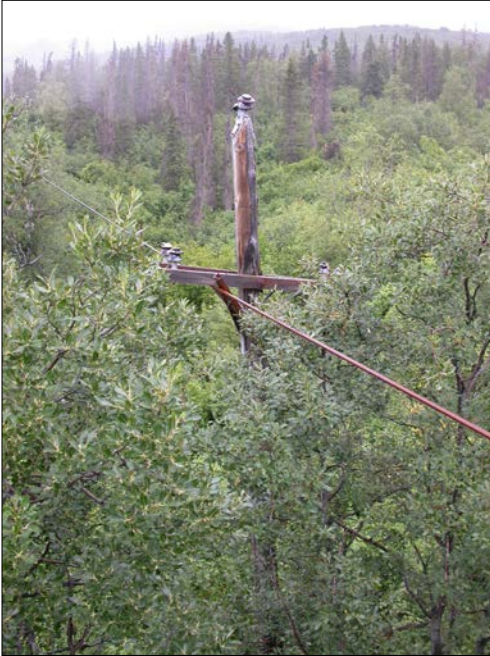
JT24: Jumbo Tower 18 (J24; T18), view E (NPS, 2003).
