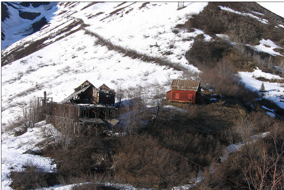
Jumbo Junction Station Complex, Operator's House (right), view E (NPS, 2006).
