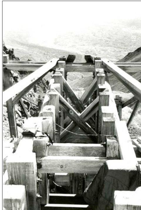
JT2: Jumbo Breakover Station 1, view S (NPS, 2003).
