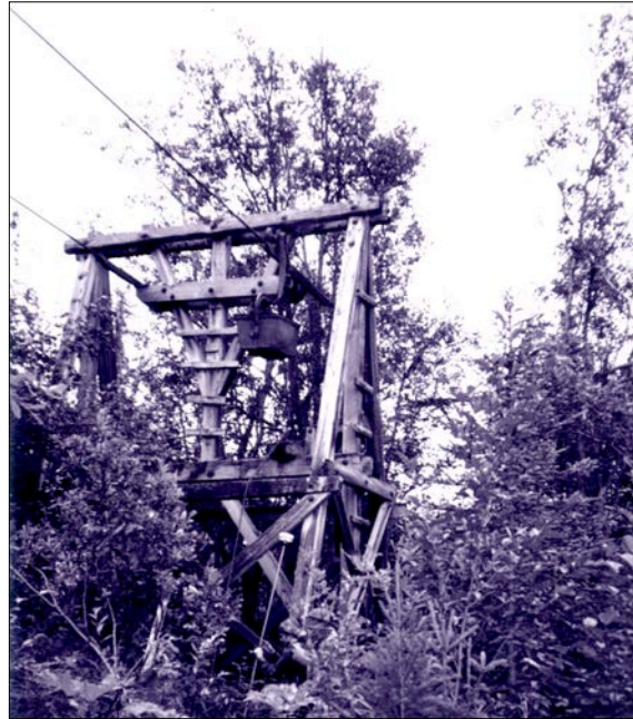
JT18: Jumbo Tower 12 (J19; T12), view SE (NPS, 2003).
