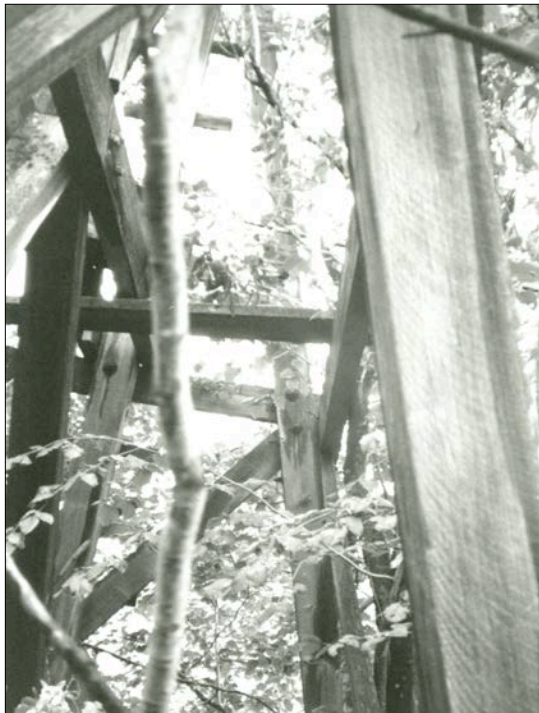
JT22: Jumbo Tower 17, view W (NPS, 2003).
