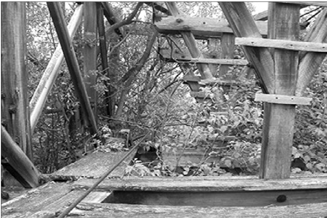
JT15: Jumbo Breakover Station 6 (J16; STA 6), view W (NPS, 2003).
