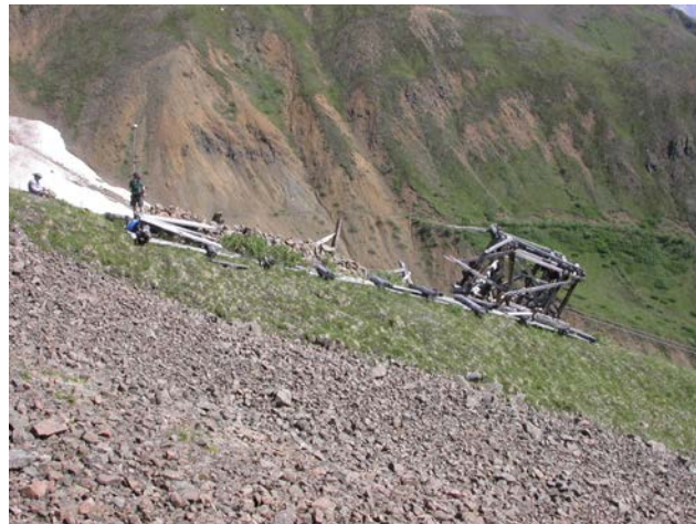
JT39: Snow Fence, view W (NPS, 2003).
