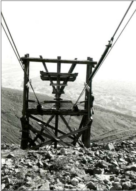
JT7: Jumbo Tower 4 (J8; T4), view SE (NPS, 1998).
