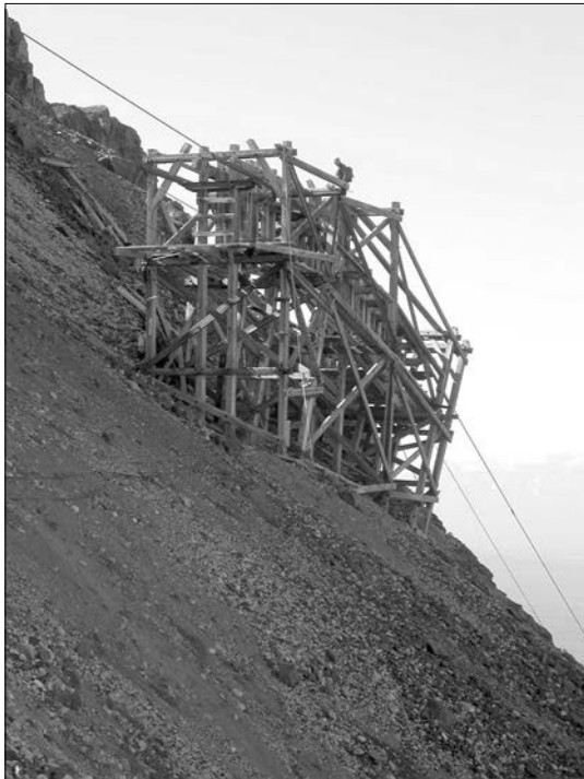
JT2: Jumbo Breakover Station 1, view S (NPS, 2003).
