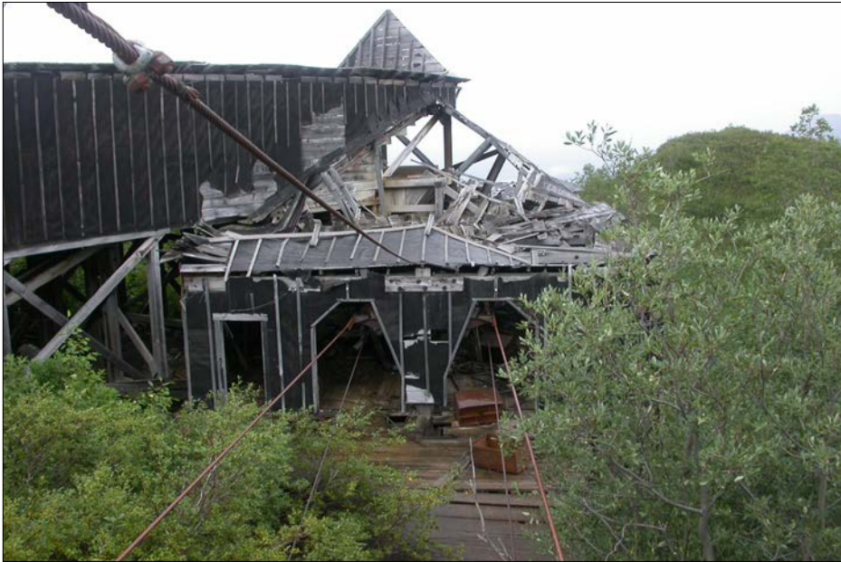
JT9: Jumbo Breakover Station 3 (J10: STA 3), view W (NPS, 2003).
