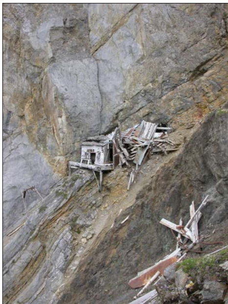
Erie Loading Station, view E (NPS, 2003).
