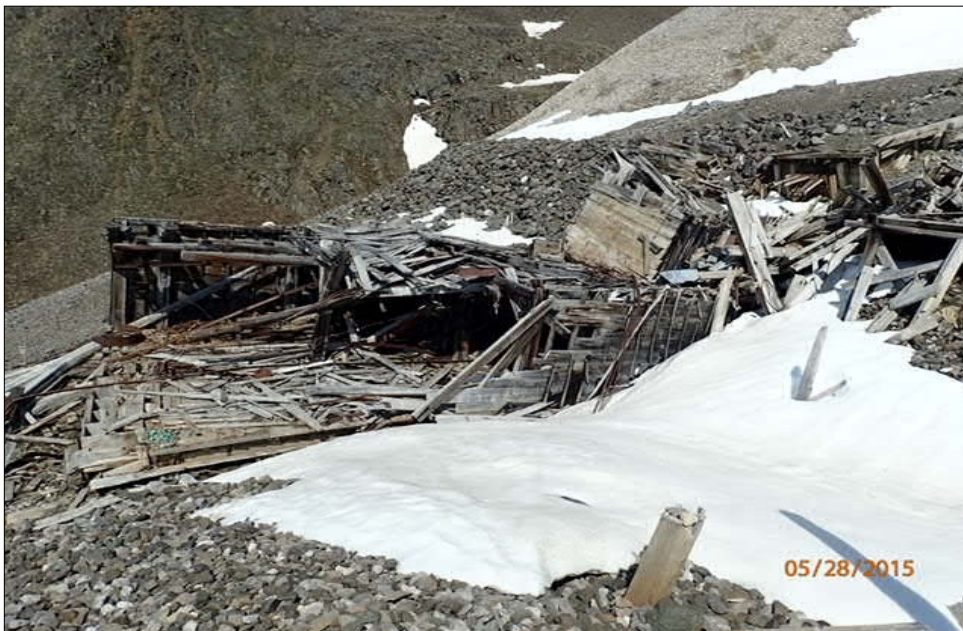
GT1: Sorting and Loading Station, view NE (NPS, 2015)
