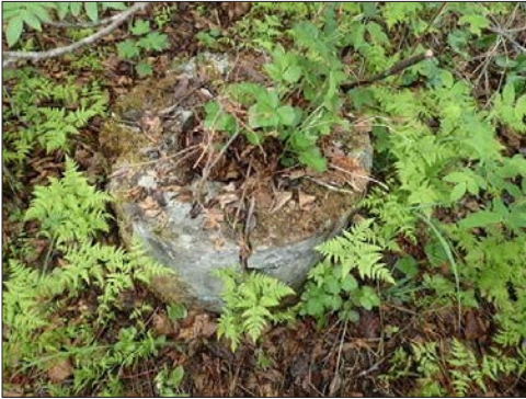
Foundation between BT15-16 (NPS, 2015)
