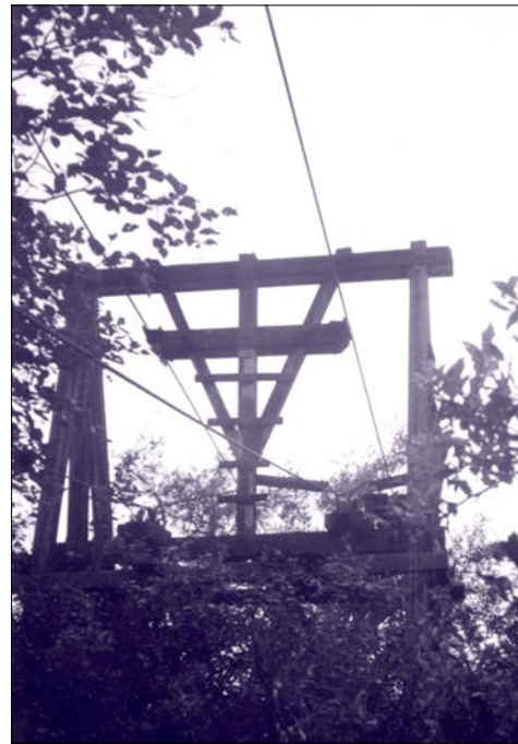
JT20: Jumbo Tower 14 (J21; T14), view E (NPS, 2003).
