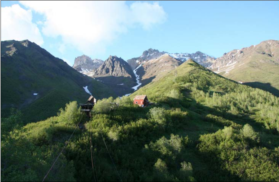
JT27: Transformer Tower (center), view E (NPS, 2008).
