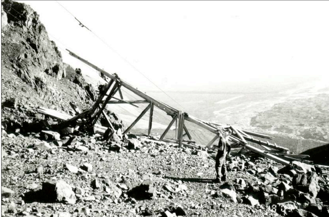
JT3: Jumbo Tower 1 (J4: T1), view SE (NPS, 2003).
