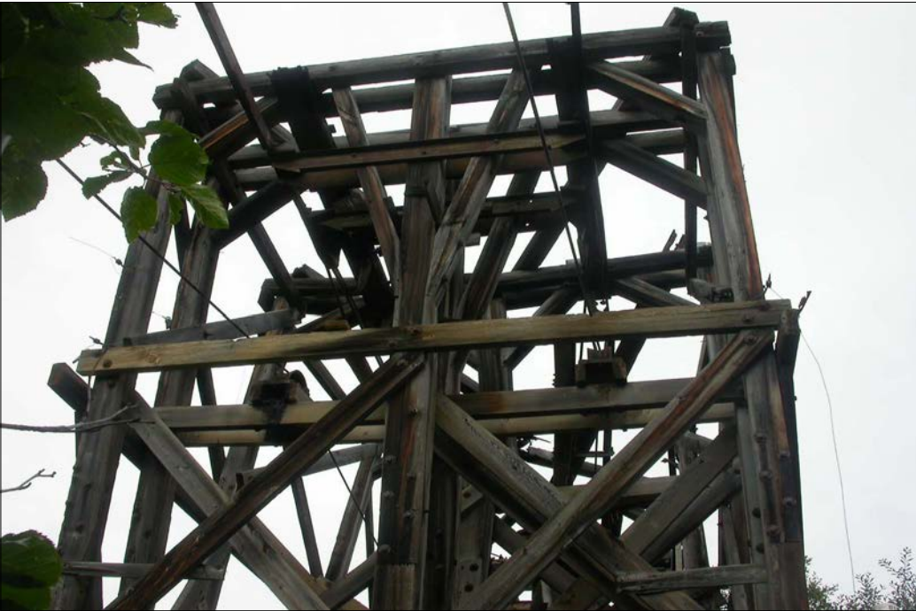
JT12: Jumbo Breakover A/T Station 5 (J13; STA 5), view E (NPS, 2003).
