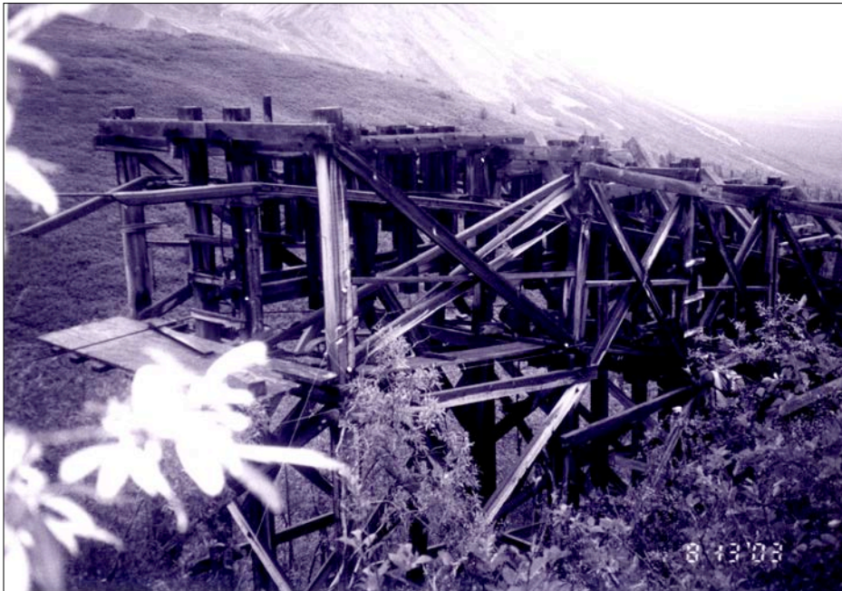
JT10: Jumbo Breakover Station 4 (J11: STA 4), view E (NPS, 2003).
