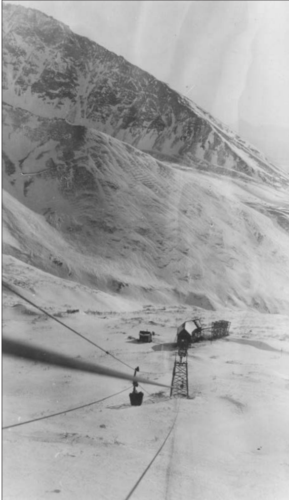
Bonanza Angle Station, c. 1922 (Courtesy of Geoffrey Bleakley).
