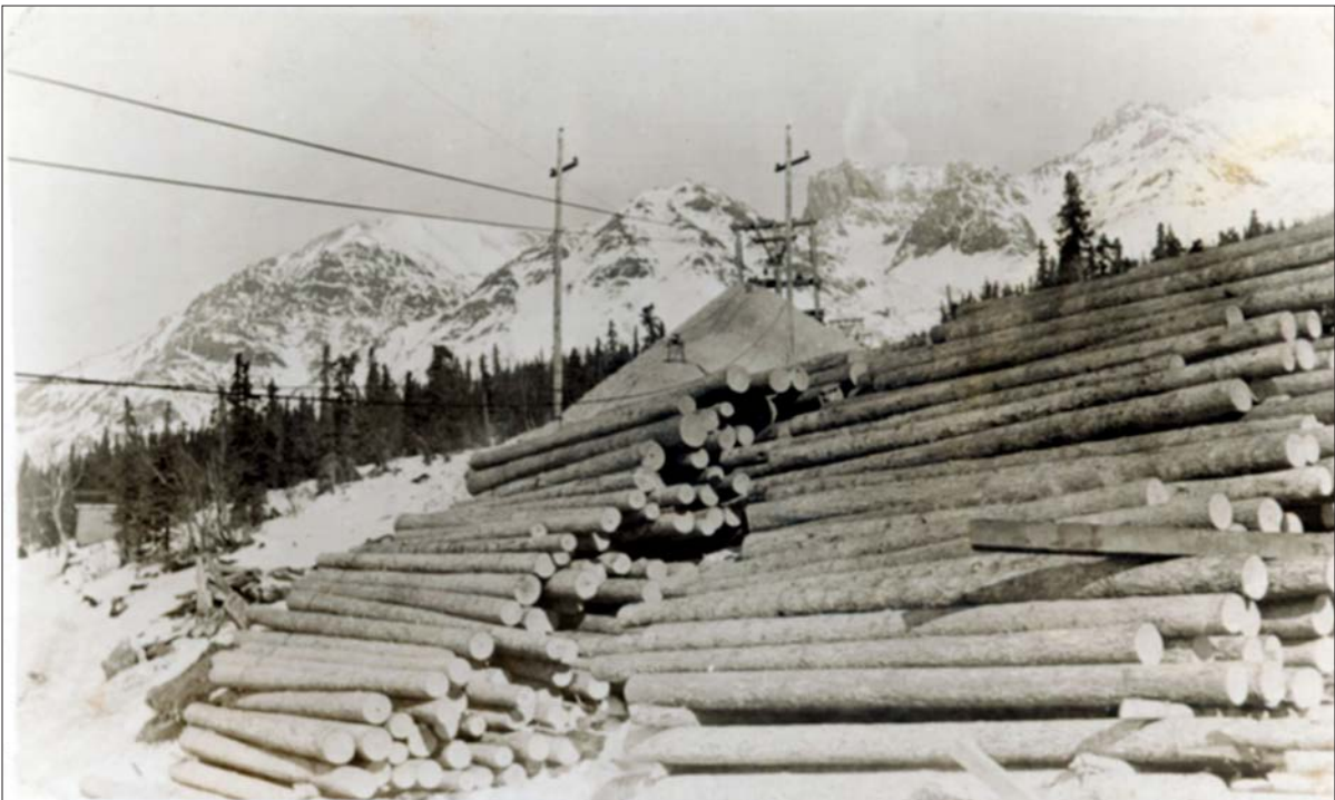
Construction of the Kennecott Aerial Tramways, c. 1908-1914 (Courtesy of the Cordova Historical Museum, 77-58-7).
