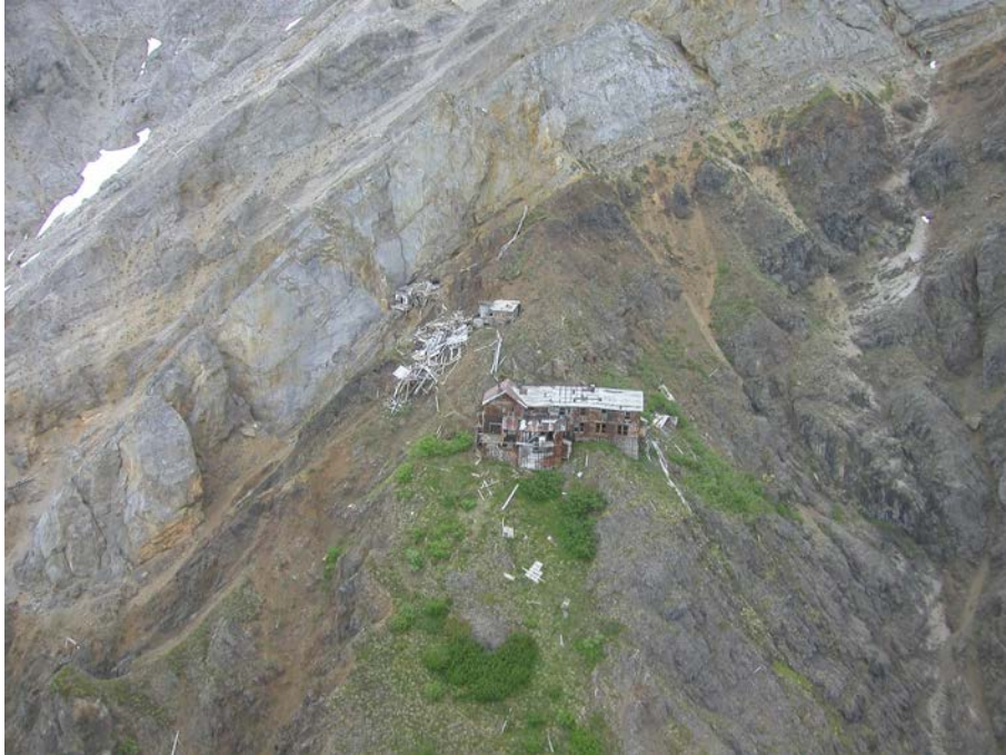
Erie Mine. Collapsed tower in bottom left corner (NPS, 2003).
