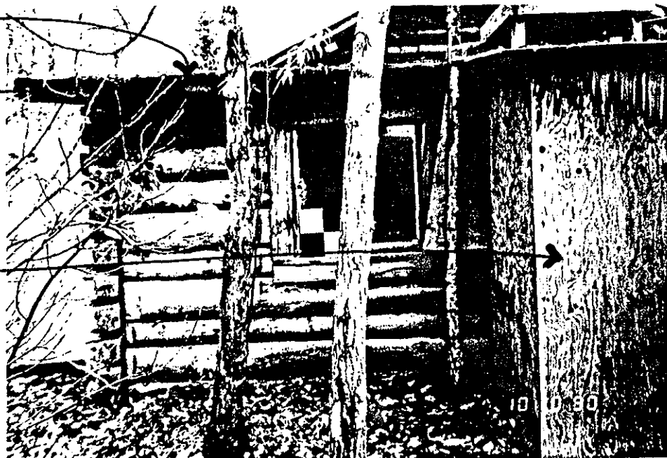
WEST ELEV - NW CORNER
