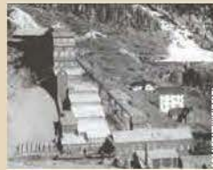
1915 The trunk train terminal is complete at the top of the Mill. Below it, a collection point for Mill tailings from sacking onto the tracks. A chute down the south side brings limestone tailings containing low-grade ore across the tracks, to be treated at the new Leaching Plant (the building with the smokestack).
