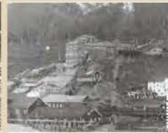
1924 Mill equipment is continuously added to and improved, and other additions are built to accommodate it. The Hancock jig addition built up the hill is expanded. Across the tracks, a Leaching Plant has been added to the Leaching Plant for wet Mill tailings, and both are in full swing.
