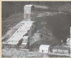
1911 The railway tracks have been laid, and a sucking shed at the bottom of the tracks to facilitate loading. The Mill's two main opposing fronts are erected and the train brings in equipment to fill them. A chute allows high-grade ore to bypass processing in the Mill and go straight to the bottom for sacking.
