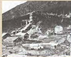
1917 A new Hancock jig addition emerges from the Mill's south face, built up the hill. Across the tracks, the Leaching Plant has been expanded and a series of conveyor belts built to deliver tailings.
