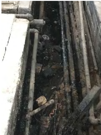
Photo 15 – Utilidor stained with Bunker C in the Powerhouse. Orientation: south. Date: 8/22/2017. Time: 1030.
