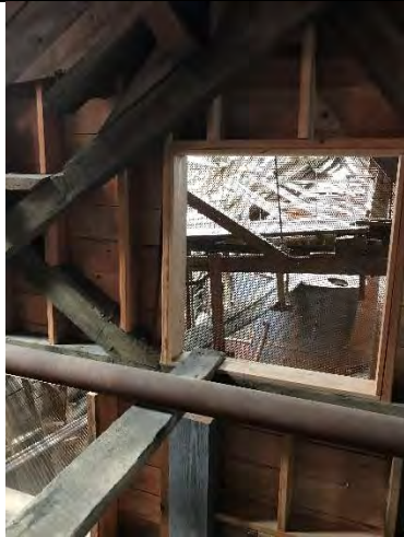
Photo 31 – Interior of Leach Plant showing old ammonia tanks. Orientation: south. Date: 8/22/2017. Time: 1118.
