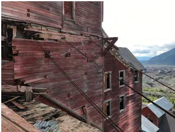
Photo 45 – North side of Mill Building. Note the original lead-based paint. Orientation: south. Date: 8/22/2017. Time: 1433.
