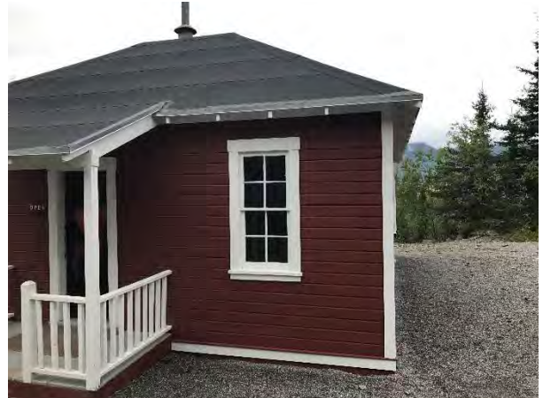
Photo 2 – Exterior of Kirkwood Cottage D. The building has been repainted. Orientation: west. Date: 8/22/2017. Time: 0939.
