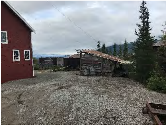
Photo 3 – Power Plant (left), Fuel Tank (center) and Storage Tank (right). Orientation: south. Date: 8/22/2017. Time: 0944.
