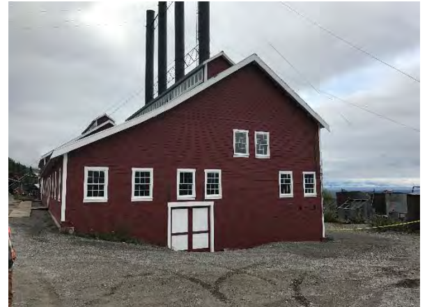
Photo 4 – Power plant Exterior. Orientation: southwest. Date: 8/22/2017. Time: 0944.
