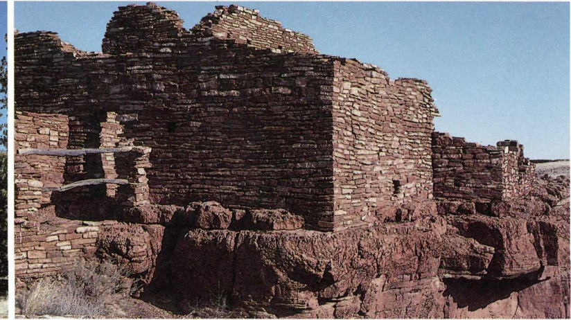
Standing on the edge of a 3/4-mile-long earth crack is the ruin known as Lomaki, or "pretty house." Earth cracks,
