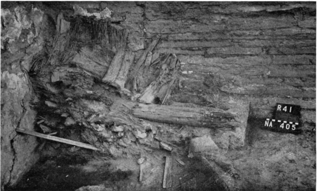
Collapsed roof. Note vigas, shakes, and juniper bark.
