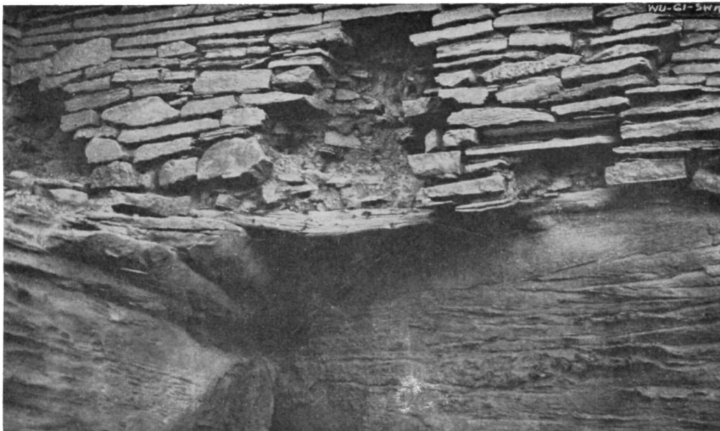
Pole-supported wall before repair, above you at Post 13.
