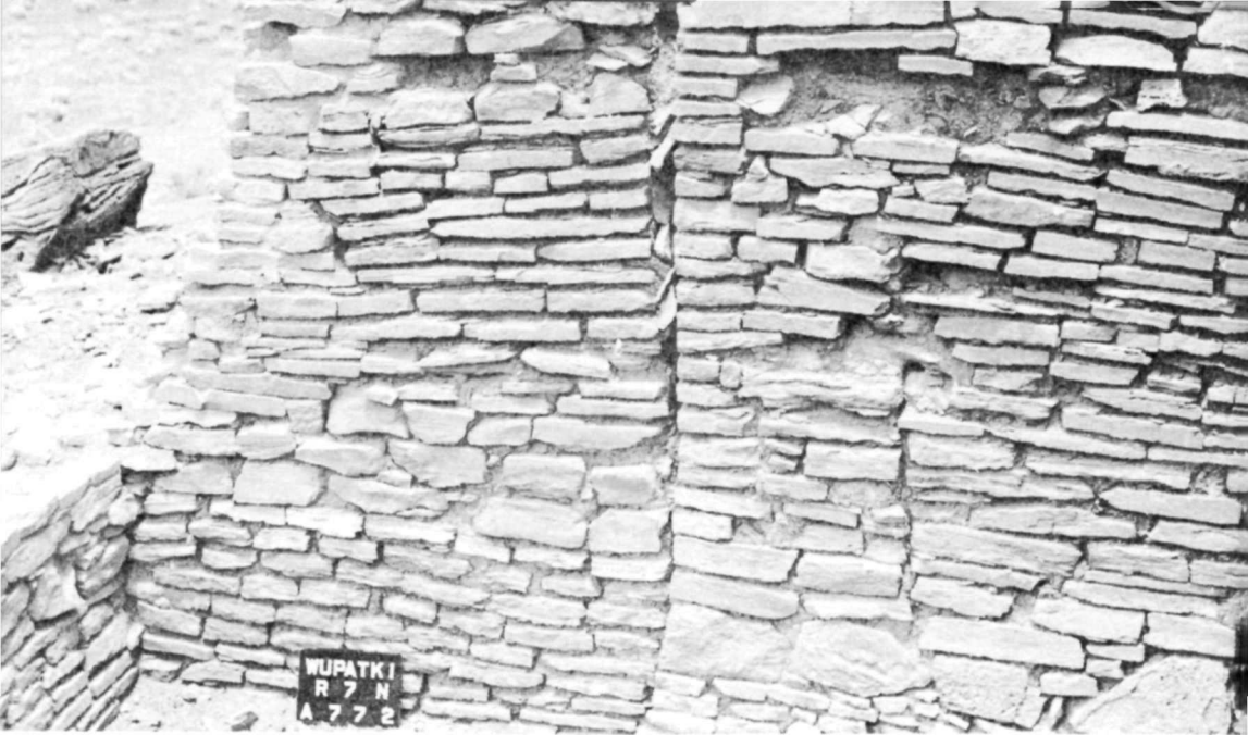
Break in wall due to lack of bonding.
