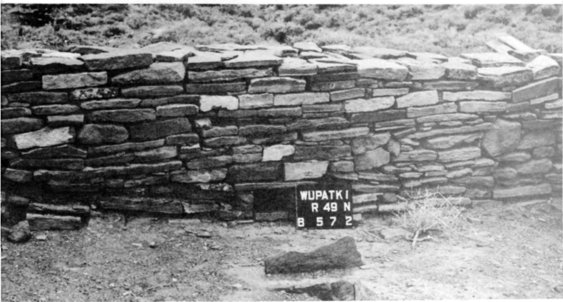
Room with firepit with a deflector between it and ventilator in wall.
