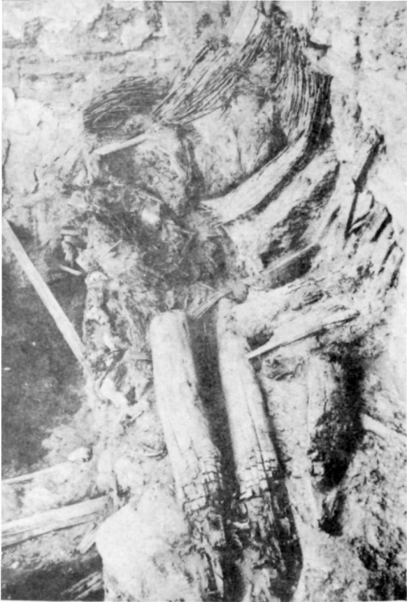
Collapsed roof. Note main beams, split beams, and juniper bark.
