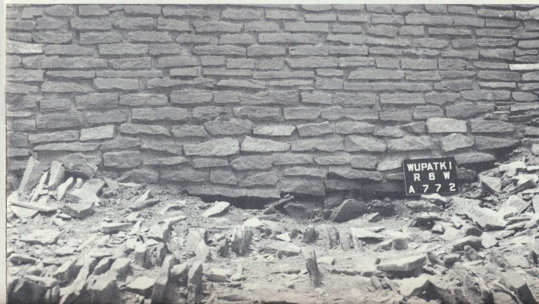
In the foreground is a collapsed wall that fell intact.
