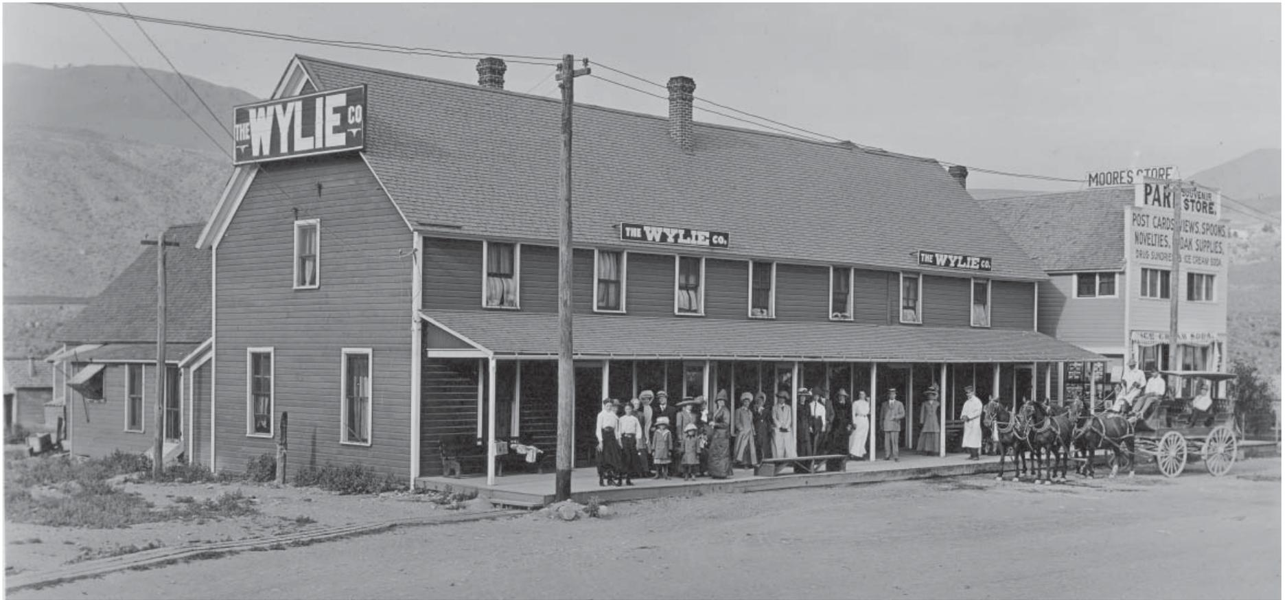
structure was a 1 ½ stories wood-framed building with simple lapboard siding. A single-story covered boardwalk spanned the entire southern façade and two brick chimneys rose from the primary roof. The windows were single-hung one-over-two windows on the upper story and larger single hung windows with four divided lights on the top and bottom.
