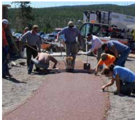
Yellow Iron Excavation in Jackson provides Yellowstone with its first FilterPave permeable, recycled pavement.
