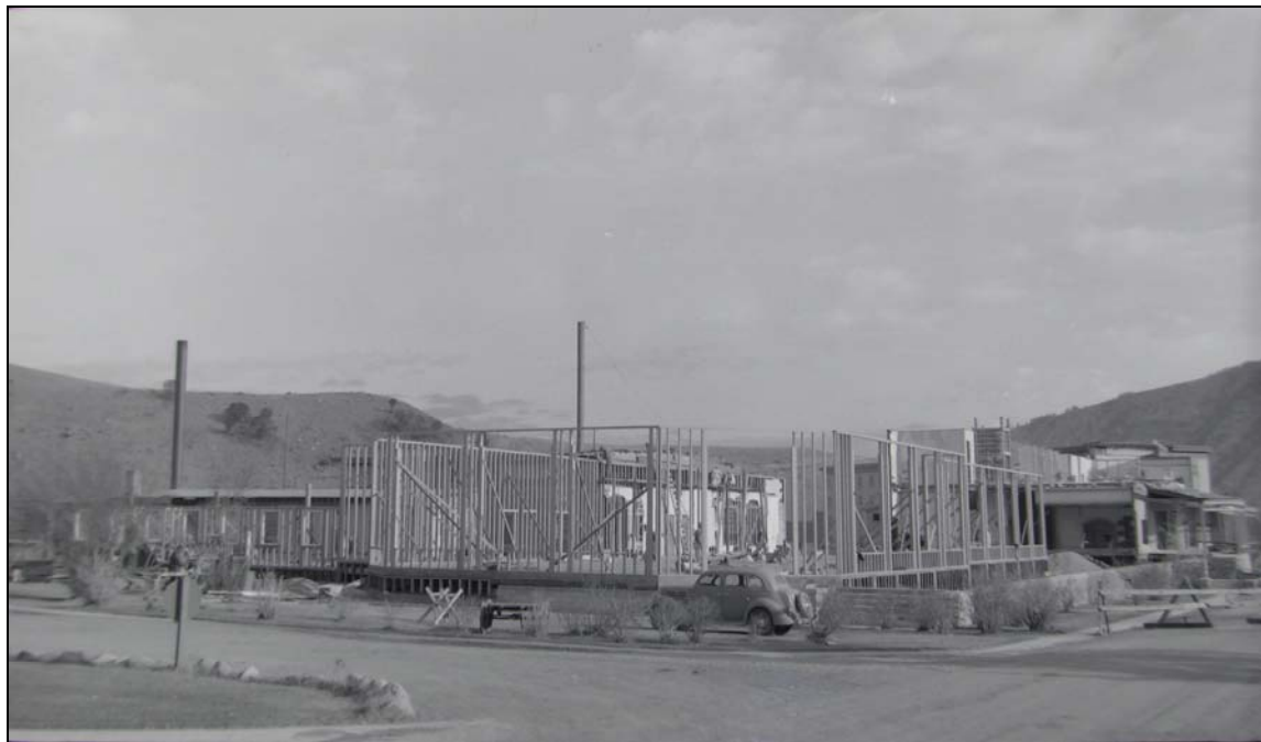
Figure H-6. Foundation and wall framing for the new dining room, October 24, 1936. (Photo No. 20773, Box W-16, Freezer 1, Yellowstone Photo Archives).
