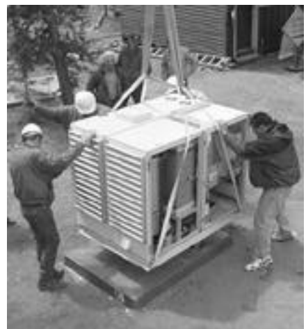
Fuel cell being installed at West Entrance on May 6, 2002. NPS photo.
