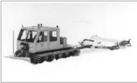
Early snow groomer 1975. By 1971, the NPS began to groom the roads regularly in order to make travel by over-snow vehicle more comfortable. This is one of their early grooming machines. NPS photo.
