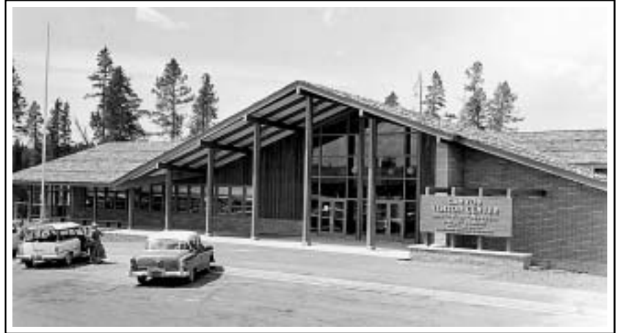
The Canyon Visitor Center, now eligible for the National Register, in 1958. NPS photo.
