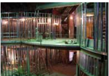
State-of-the-art lighting and climate control systems will reduce energy consumption and provide optimal indoor air quality.
