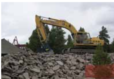
Concrete from the old visitor center was crushed and reused as fill material for the new building.
