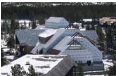
The building has been wrapped in energy-saving and weatherproof Tyvek CommercialWrap®, courtesy of a generous donation from DuPont Building Innovations.
