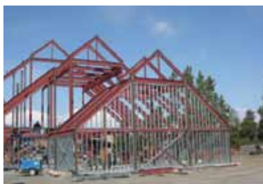
The building uses frames made of recycled steel obtained locally, which reduced transportation costs and fuel emissions.
