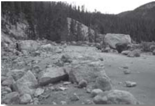
The road at Gibbon Falls was blocked by boulders shaken loose by the earthquake. NPS Photo
